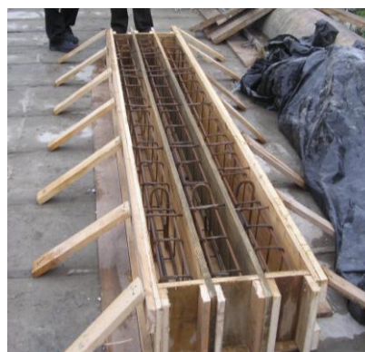
Figure 13. Moulds with placed reinforcement.
