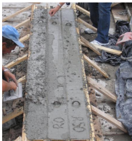
Figure 14. Finishing of the beams concrete surface.
