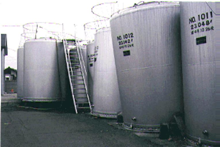
Wherever there was lateral spreading of soils and retaining structures along the shoreline, extensive damage was observed to tank farms (tank tilting), silos (tilting and collapses), cranes, stacks, and other such structures. Several tall, industrial, reinforced concrete stacks were leaning, and at least one collapsed. The collapsed stack was observed at a steel facility along the waterfront in Nishinomiya. The upper one-third of the stack broke off and embedded into the adjacent building.
