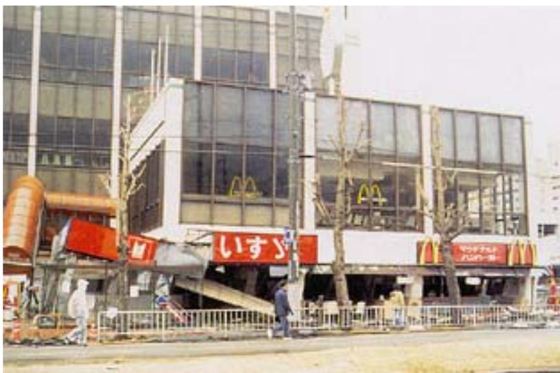
Top: Mid-height collapse of a concrete-frame building.
