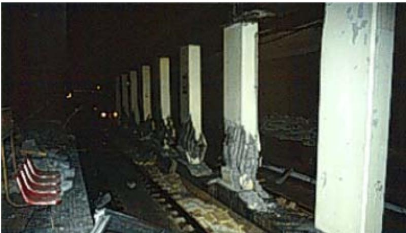
*Top: A section of the severely damaged Shinkansen (Bullet Train) elevated roadway. The structure is very stiff and very strong, but had inadequate shear reinforcement.*
