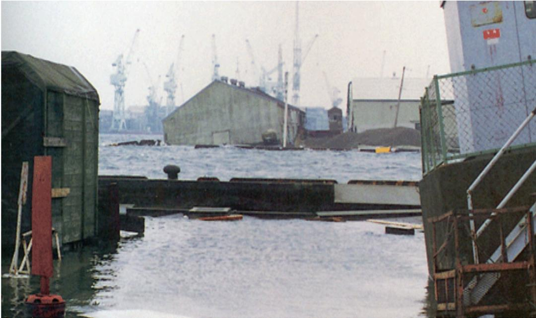
Top: Partially submerged pier and buildings at the older section of the Port of Kobe.
