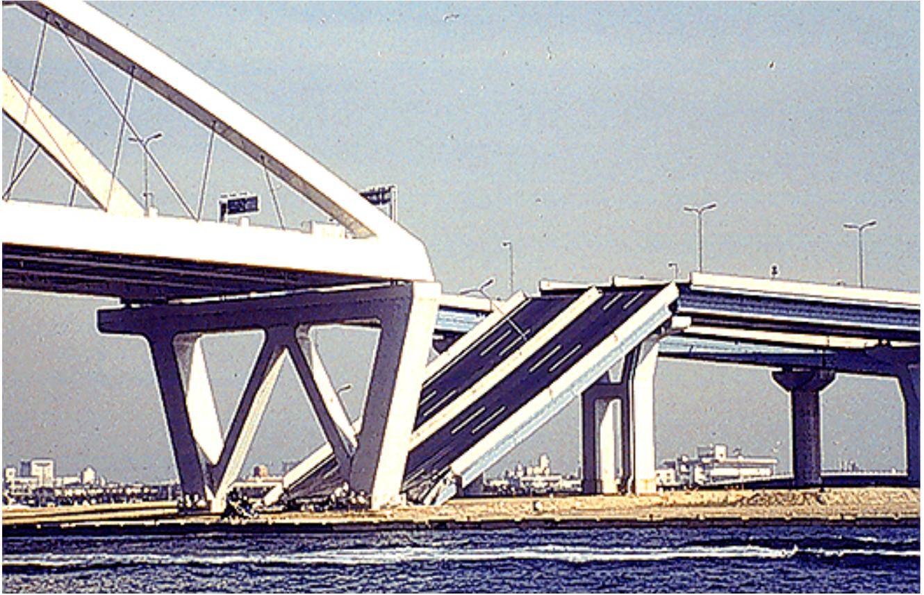
*Top: The collapsed approach to the 252-meter-long main span of the Nishinomiya Bridge east of Nishinomiya Port on the new Wangan Expressway. The failure was caused by inadequate strength and capacity of the mechanical bearings to take very large displacements in both the transverse and longitudinal directions.*
