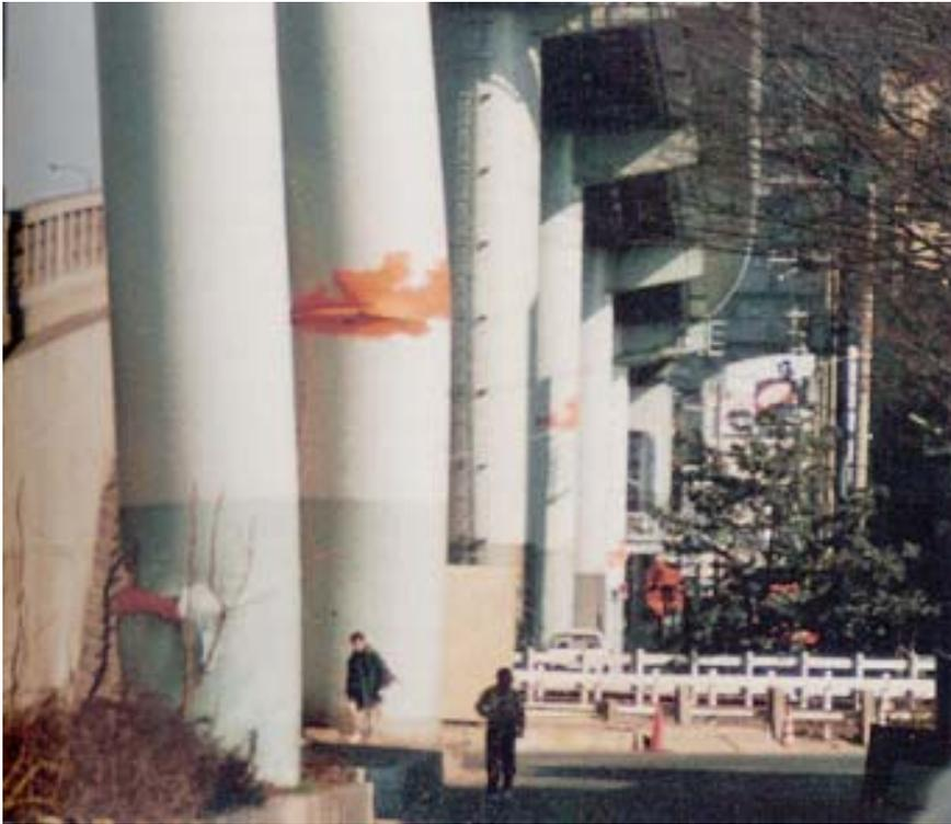
*Top: Buckling failure (bending) of steel-encased columns supporting the Hanshin Expressway.*
