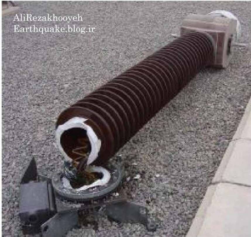
Figure 2: A broken CT
