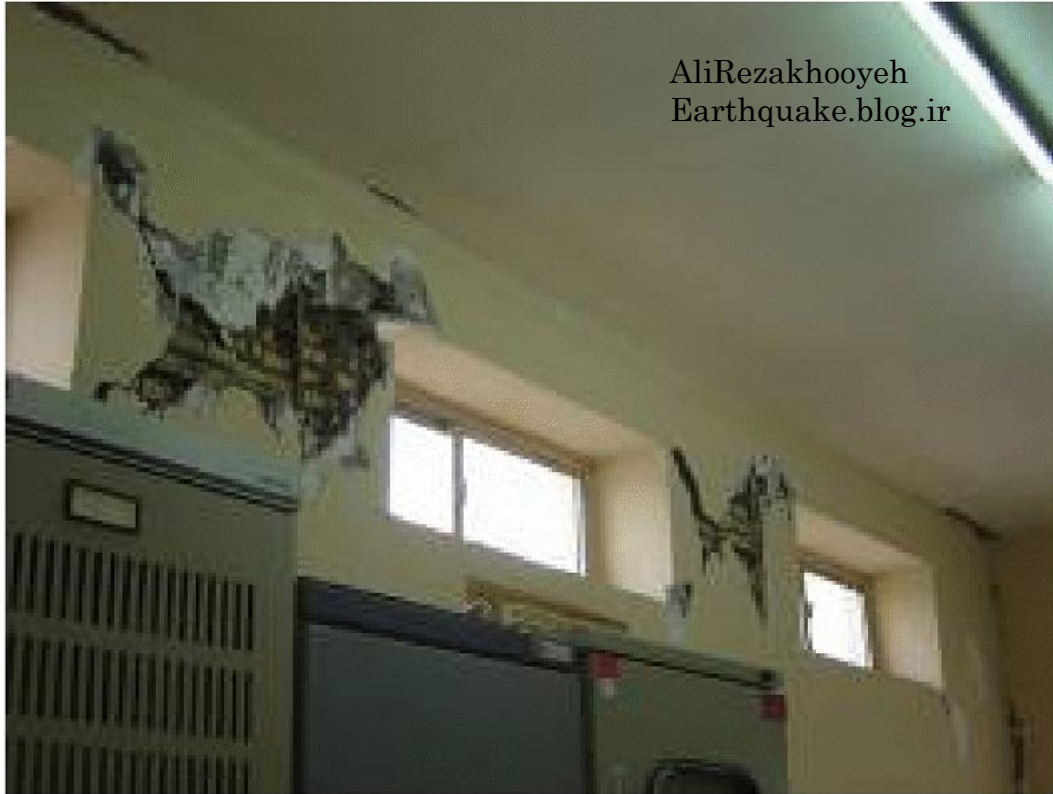
Figure 12: Damages to control building
