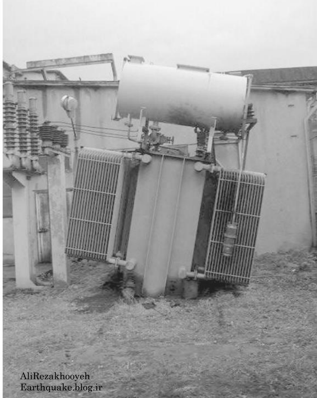
Damage to a transformer at the SEKA paper mill was expected to shut down this unit for several weeks.
