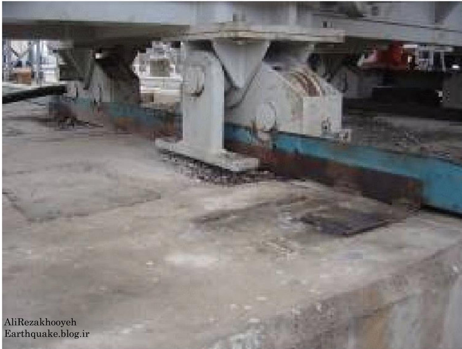
Figure 10: Transformer base after retrofit
