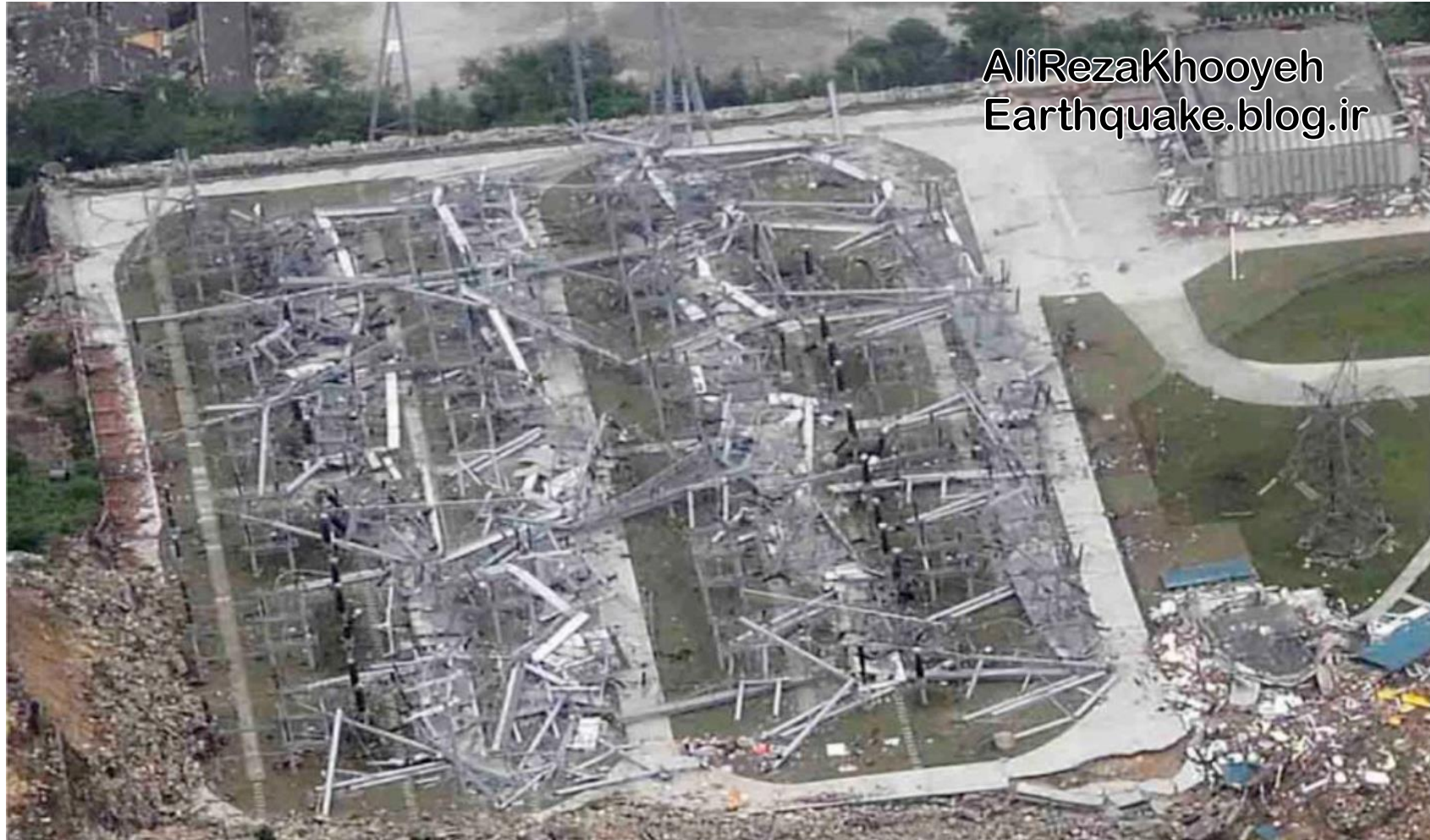
220 kV Ertai Substation, Yingzhou
