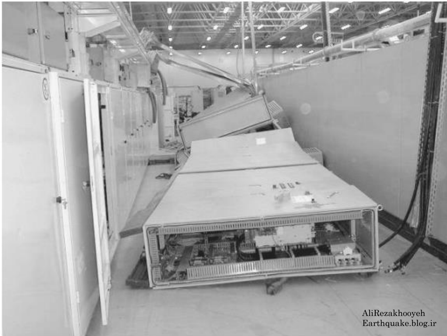
Collapse of unanchored cabinets at the Toprak Saglik facility.
