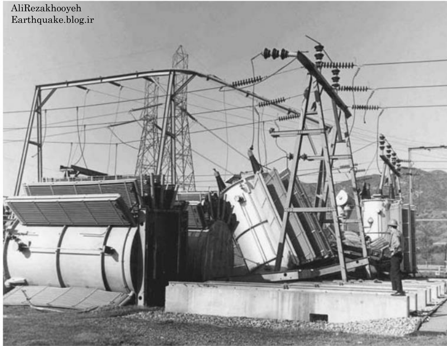
Damage to transformers due to inadequate anchorage.
