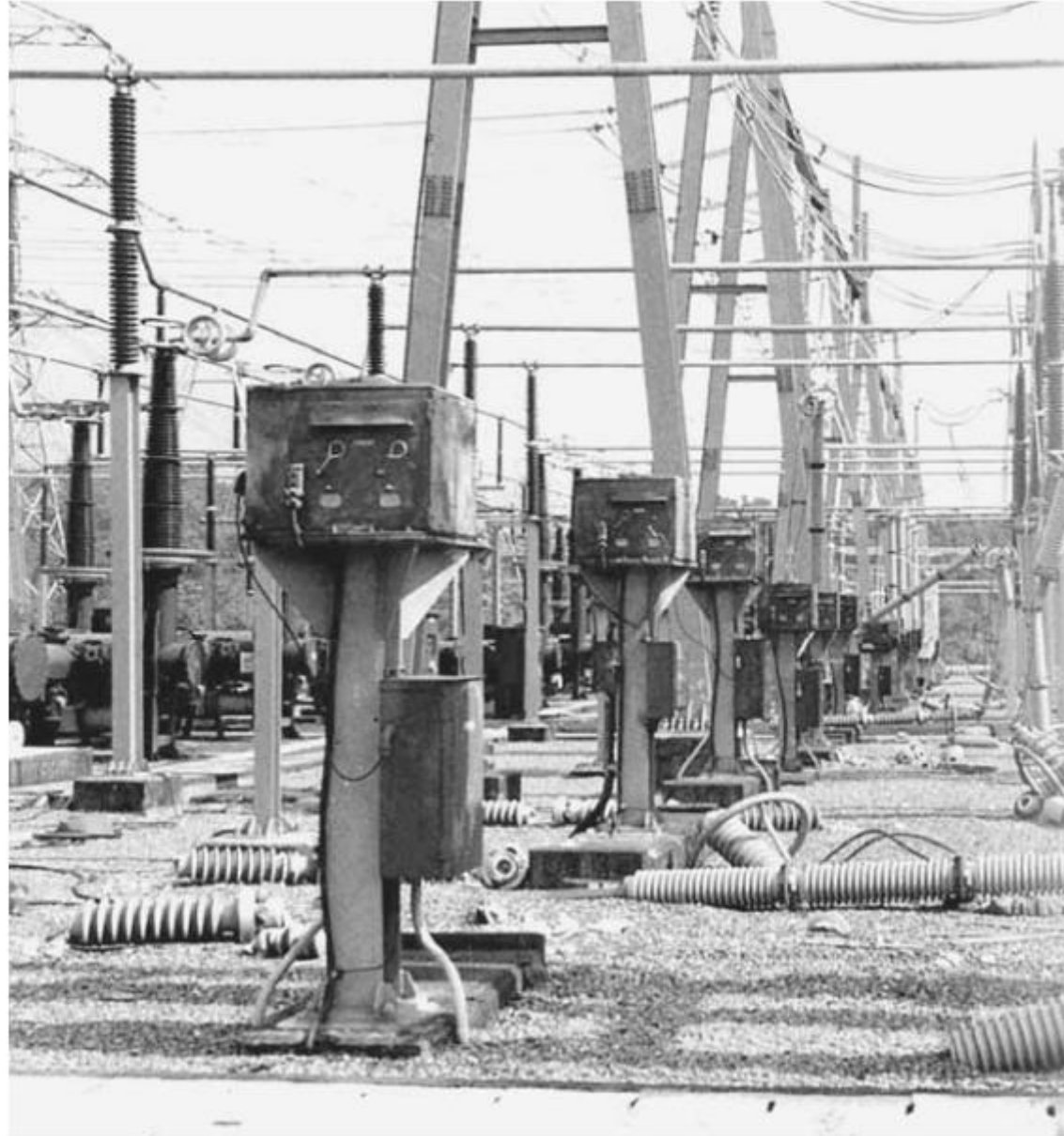
FIGURE 25.2 Damage to switchyard equipment.
