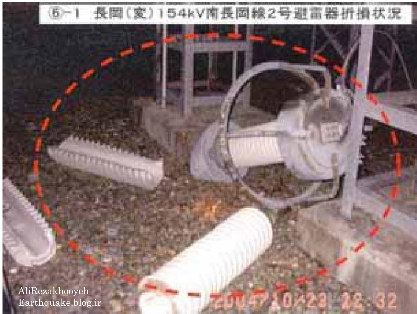
Figure 1 Lightning arresters of all three-phases were broken in Nagaoka Sub. (JSCE, 2004)
