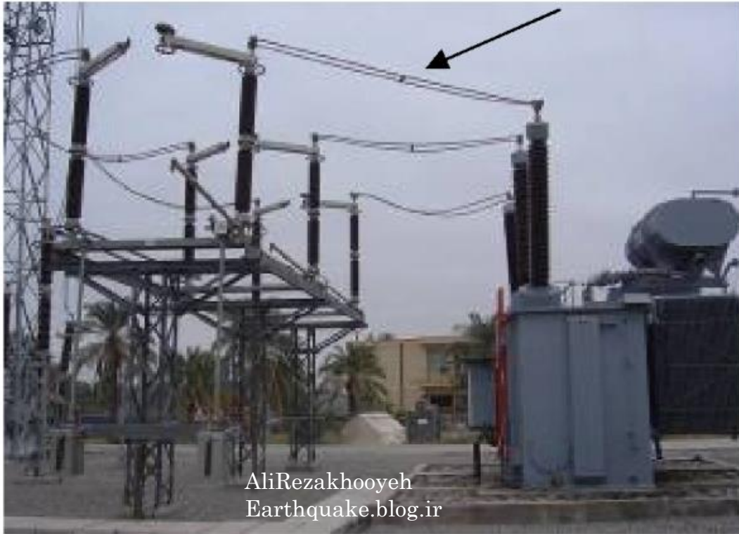
Figure 6: Pulled conductor
