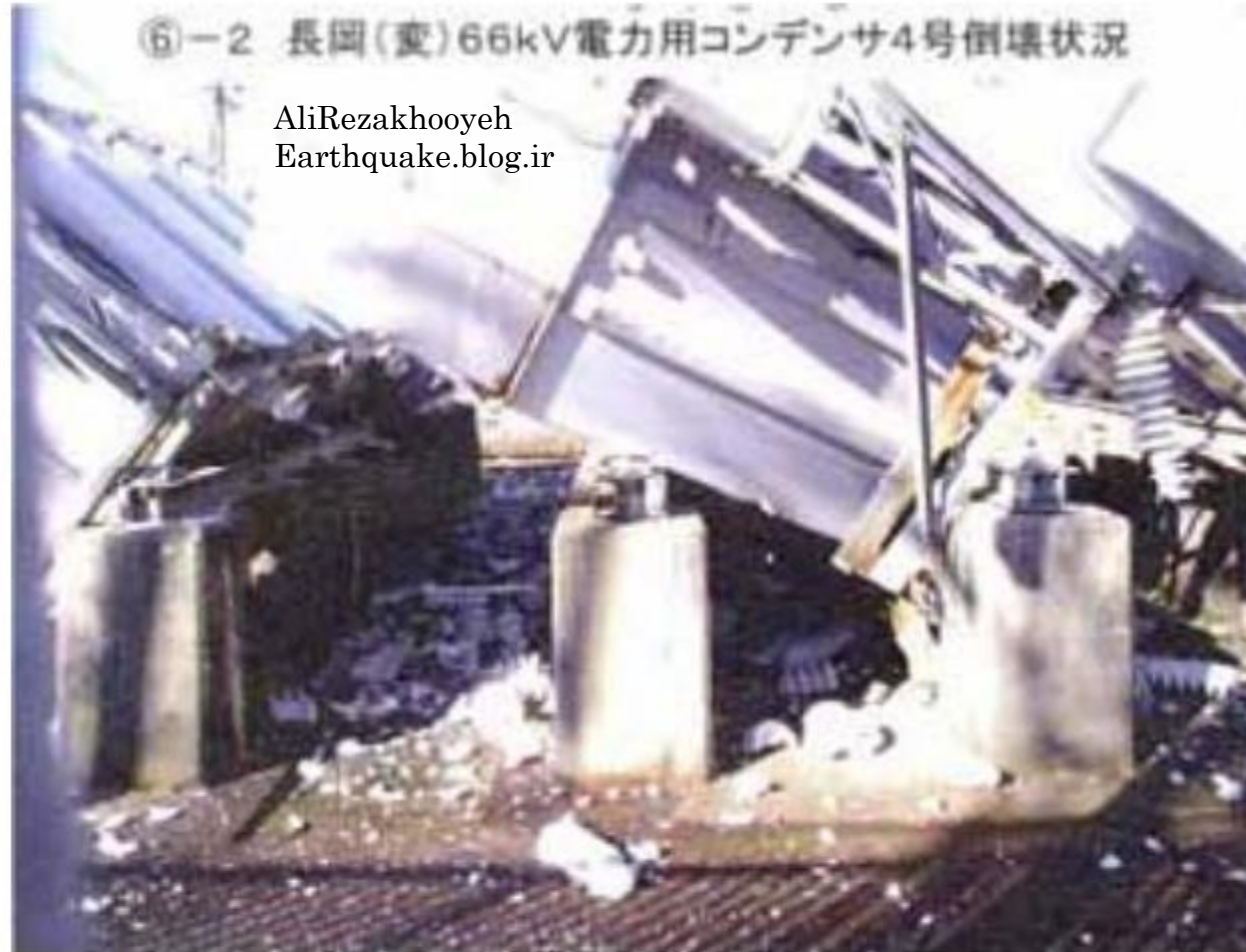
Figure 3 Failure of condenser in Nagaoka sub. (JSCE, 2004)
