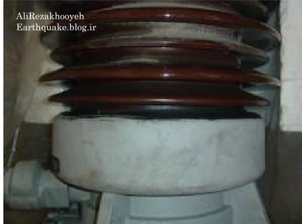
Figure 15: Damaged bushing
