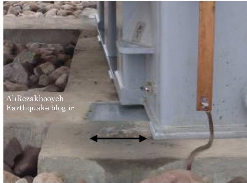
Figure 7: Sliding of non-anchored equipments
