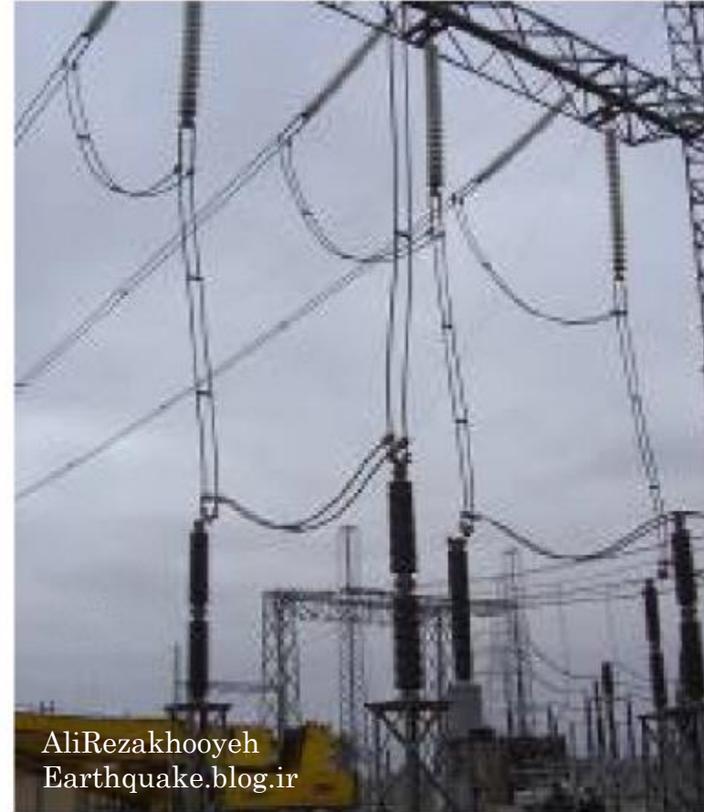
Figure 9: PI and voltage transformers
