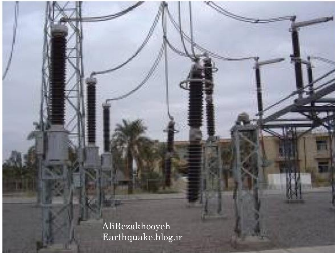
Figure 8: Broken surge arresters
