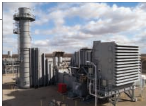
FIGURE 3. The modern aero-derivative gas turbine installation shown here includes a 100-MW gas turbine. The inlet air system, gas turbine and exhaust gas system are also shown
