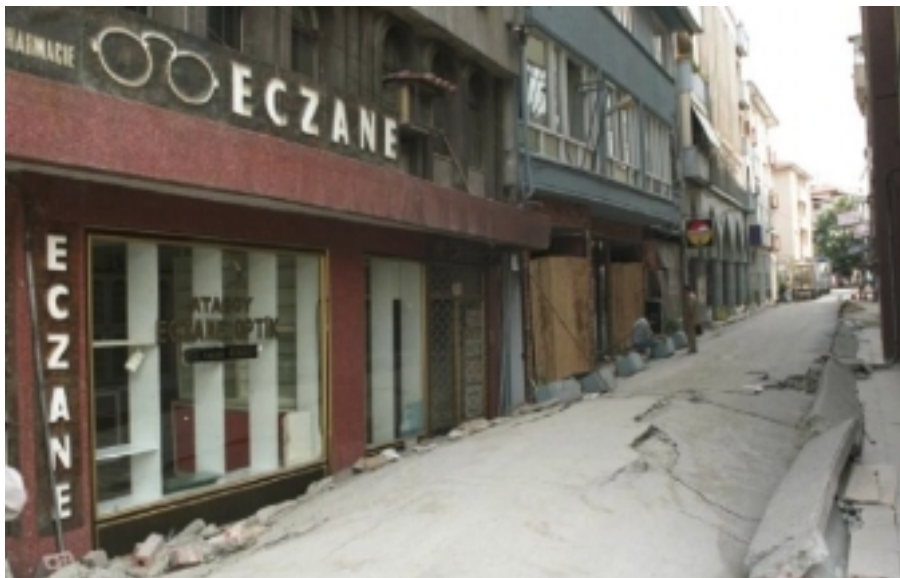
Figure 13. Building in Adapazari that sank into the ground and the displaced soil heaved
