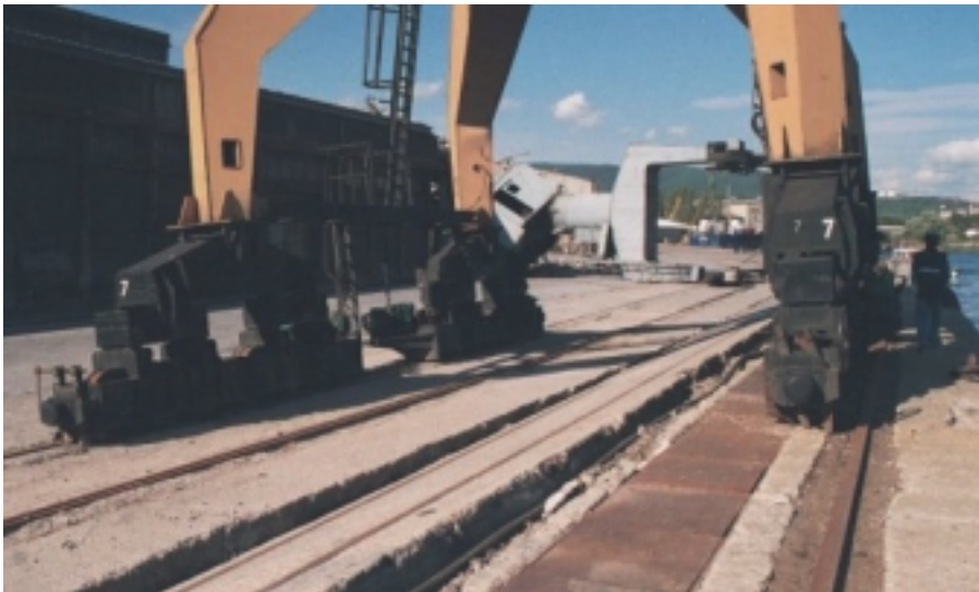
Figure 30. Damage at Derince Port in Kocaeli Earthquake
