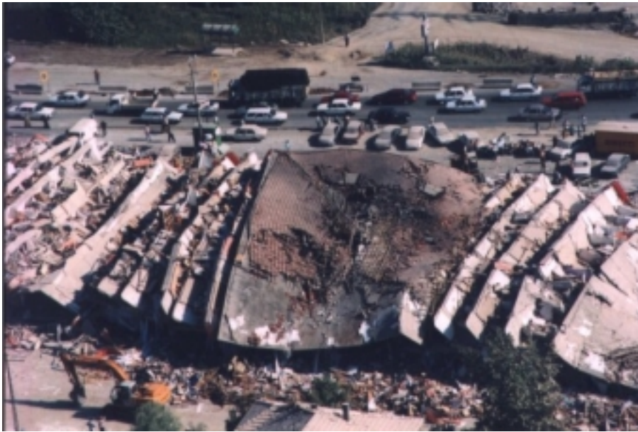
Figure 18. A “pancake” type collapse in Kocaeli Earthquake
