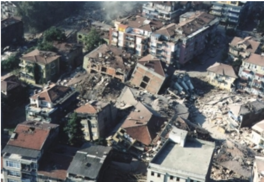
Figure 17. A general view of building damage in Duzce
