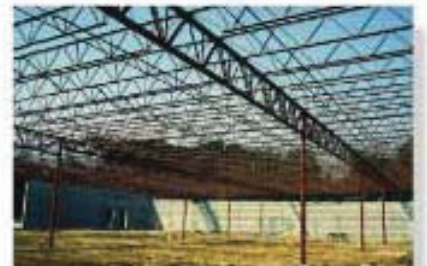
Typical interior steel pipe columns used to support the roof of a single story building.
