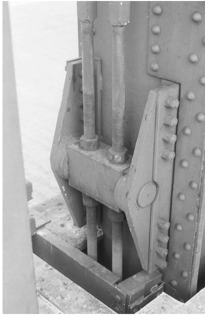
Figure 5-13 Span Drive Vertical Lift Bridge—Operating Rope Adjusters. The adjusters are attached to the towers. The ends of the operating ropes are tensioned and adjusted by means of the threaded rods.
