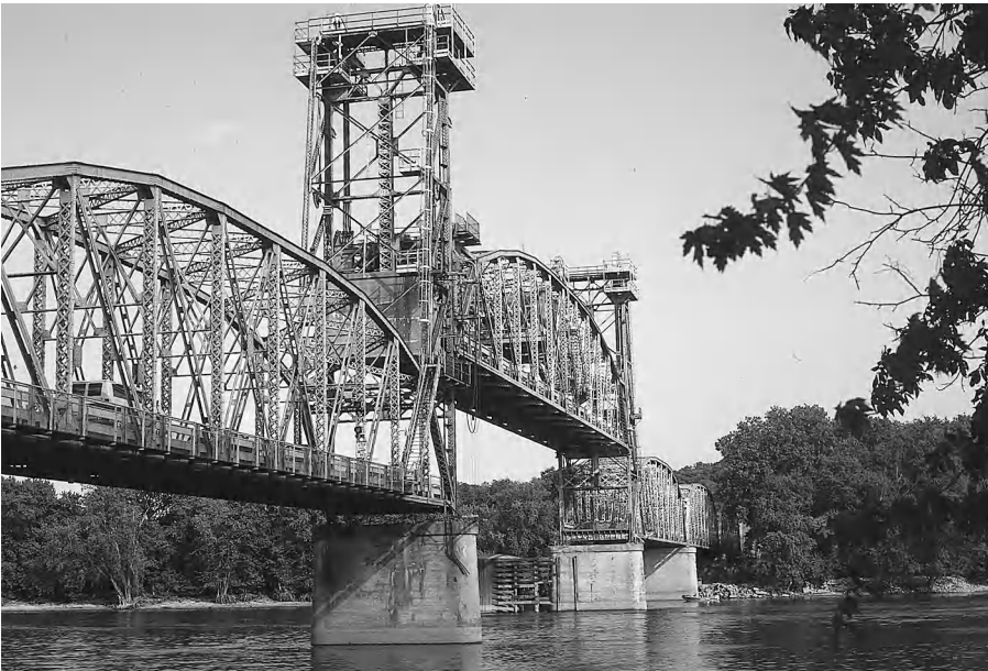
Figure 5-15 Strauss Vertical Lift Bridge. This example, over the Illinois River, is now in the process of being removed and replaced with a high level fixed bridge. It is a fairly conventional vertical lift span, but is operated by racks and pinions instead of ropes (see Figure 5-16).
