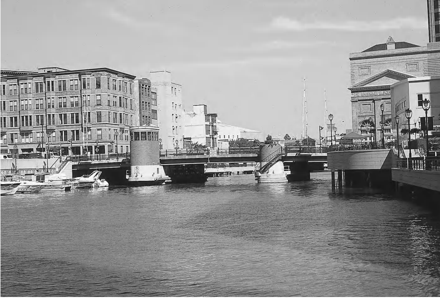
Figure 5-21 Towerless Vertical Lift Bridge. Several of these modern towerless vertical lift bridges cross the Milwaukee River in downtown Milwaukee, Wisconsin.
