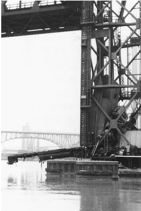
Figure 18-1 Accident at Railroad Vertical Lift Bridge. The bridge was opened as the train was approaching, with insufficient time or distance to stop. (Photo courtesy of John McCown.)
