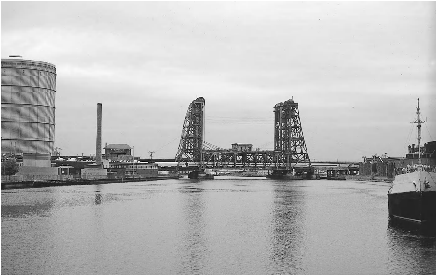
Figure 3-1 Dock Bridges, Newark, New Jersey. This is a combination of three semi-independent vertical lift bridges. The nearest has one track; the middle has two tracks at two different elevations, with one at a gradient; the far one has three tracks.
