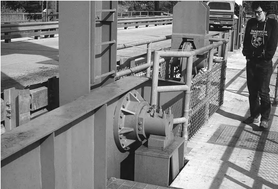
Figure 4-11 Trunnion Detail—Strauss Overhead Articulated Counterweight Bascule. The near trunnion is the main trunnion, the counterweight trunnion is to the rear.
