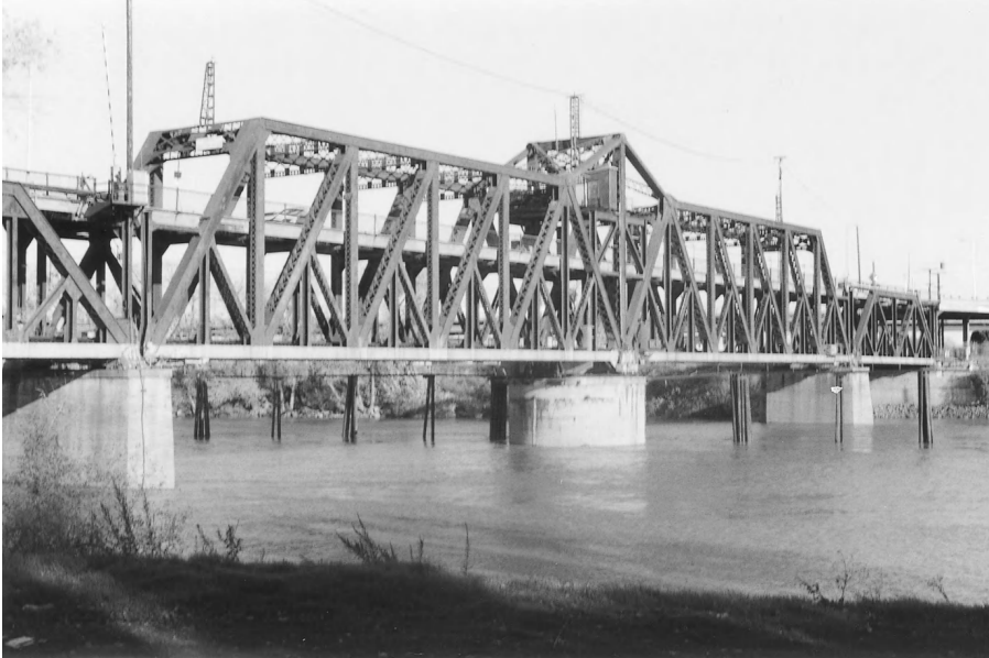
Figure 6-4 Very Large Center Bearing Swing Bridge. This bridge was one of the first successful very large swing bridges not to be supported on a rim bearing. It is even heavier than the bridge shown in Figure 6-3.
