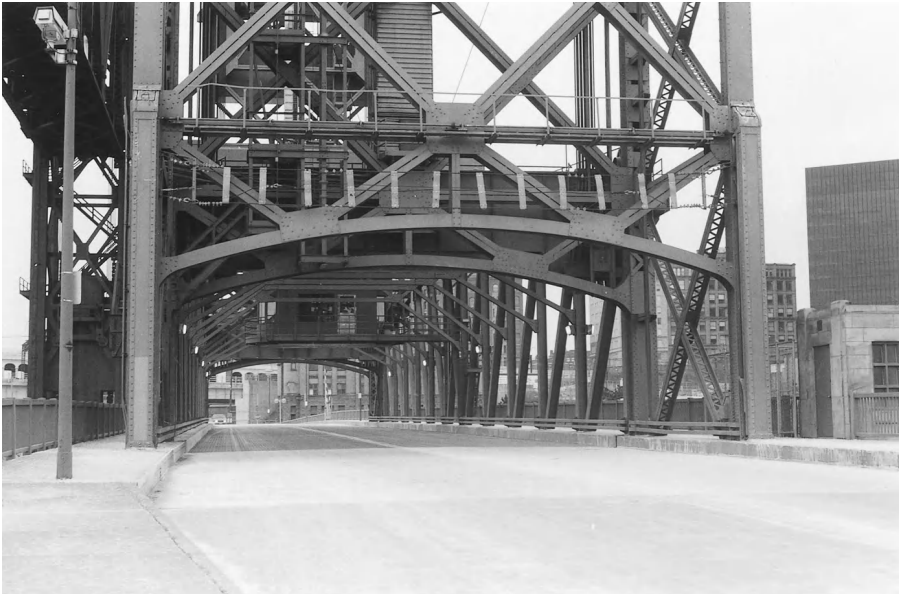
Figure 18-2 BSMB Impact-Absorbing Barrier Gate. This gate, shown in the raised position, drops to block the roadway when the bridge is to be opened. If a vehicle hits the gate, the gate extends, slowing the vehicle, and the impact causes wire ropes to be drawn through a braking mechanism, absorbing the kinetic energy of the vehicle.
