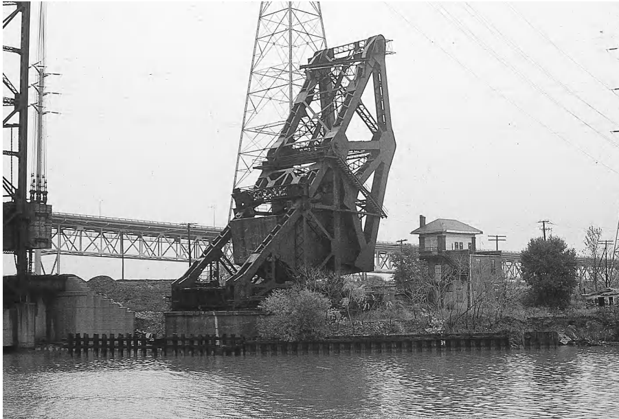
Figure 10-1 Bascule Bridge Remains after Collision with Ship. This bridge was not fully protected from impact as a ship passed in the narrow channel. The bascule span was completely torn free of its supports.
