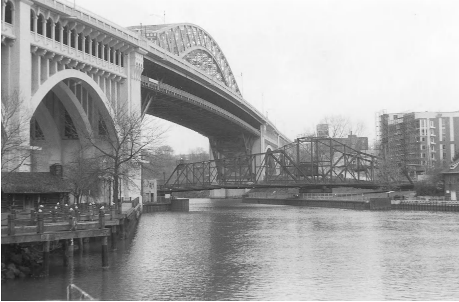
Figure 6-7 Swing Bridge under Fixed Bridge. This application of swing bridges, to fit under a high-level fixed bridge, has been repeated in congested areas.
