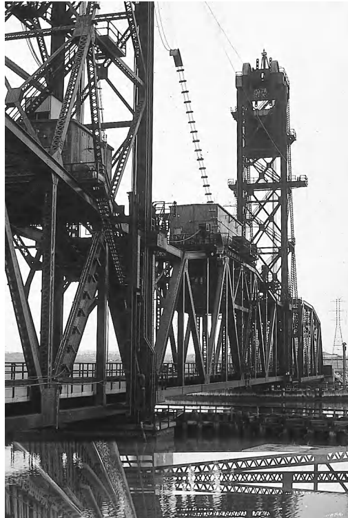
Figure 12-4 Vertical Lift Bridge Auxiliary Counterweight. The diagonal ropes extending from the center of the vertical lift span to the towers reach down and connect to weights hanging alongside the tower legs. These ropes pull up on the span when it is down, and down when it is up, compensating for the weight of the counterweight ropes.
