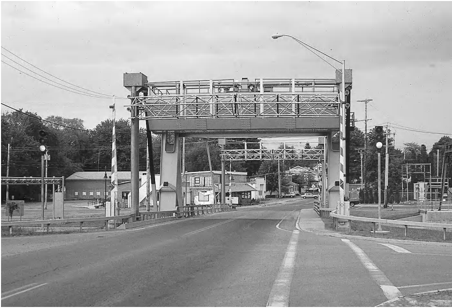
Figure 18-3 Entwistle Metal Bender Barrier Gate. This gate, shown in the raised position, drops to block the roadway when the bridge is to be opened. If a vehicle hits the gate, the gate extends, slowing the vehicle, and the impact causes stainless steel strips or bars to be drawn through a convolution of rollers, absorbing the kinetic energy of the vehicle.
