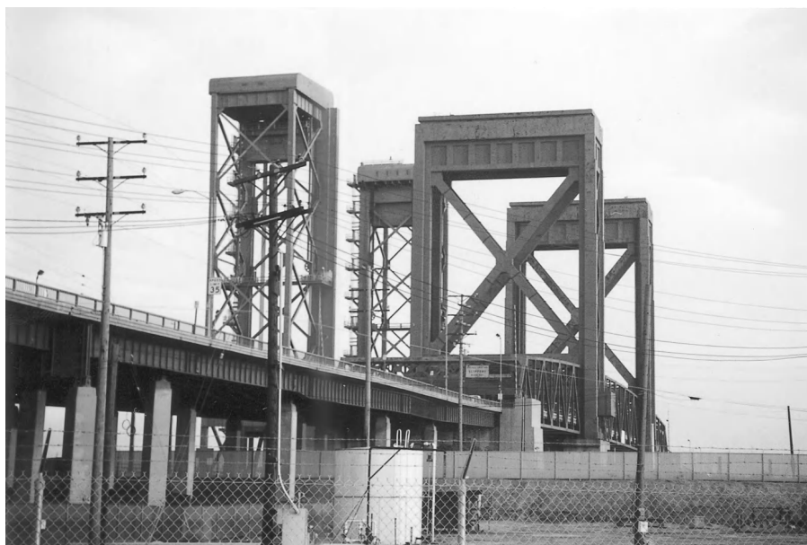
Figure 5-2 Commodore Schuyler Heim Bridge, Long Beach, California. This bridge on the right, built in 1948, is a very wide tower drive vertical lift span. The adjacent bridge is the relatively new (1997) Alameda Corridor bridge to Terminal Island.
