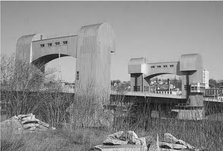
Figure 5-4 Troy-Green Island Vertical Lift Bridge. This bridge has four separate counterweights, one in each tower.
