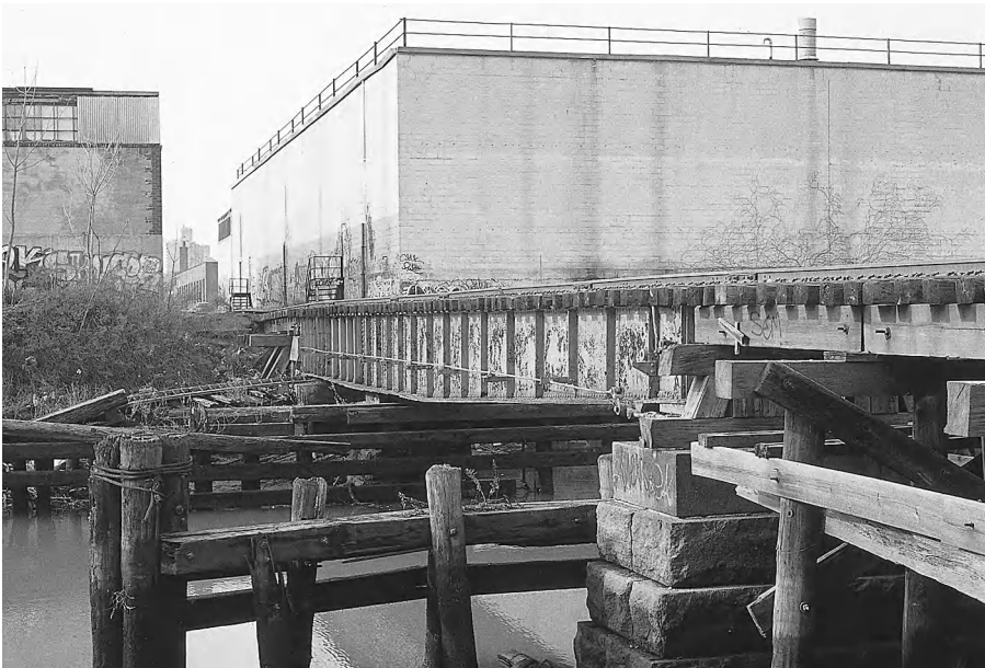
Figure 6-6 Bobtail Swing Bridge. Typical of such structures of older construction.
