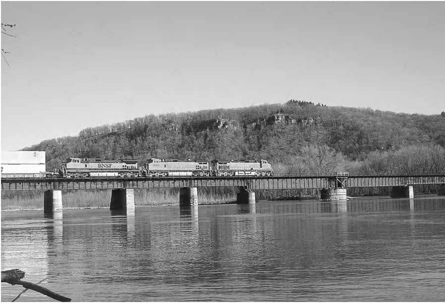
Figure 3-6 Removable Span over the Wisconsin River. This bridge, built in 1908, has probably never had to be displaced for navigation since it was erected. The removable span is one of the large girder spans supported at one end by the round pier.
