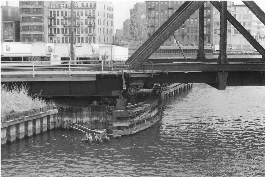
Figure 13-5 Swing Bridge Eccentric Roller End Lift. This type of lift is not very common. The mechanism rotates an eccentric shaft, causing the roller to lift or lower, lowering or raising the end of the swing span.
