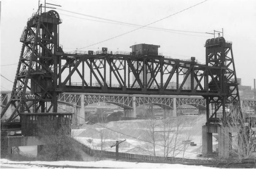
Figure 5-6 Waddell Type Span Drive Vertical Lift Bridge. This type of vertical lift bridge is driven via ropes from the machinery room on the vertical lift span.
