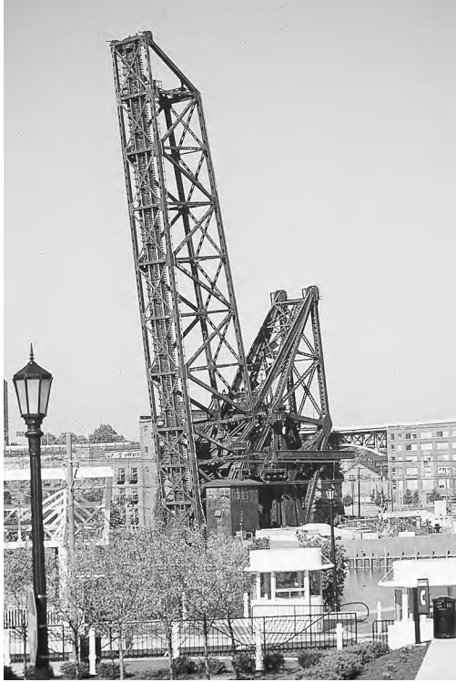
Figure 4-10 River Street Bascule, Cleveland, Ohio. This single leaf, single track heel trunnion bascule bridge span length is more than 220 ft.
