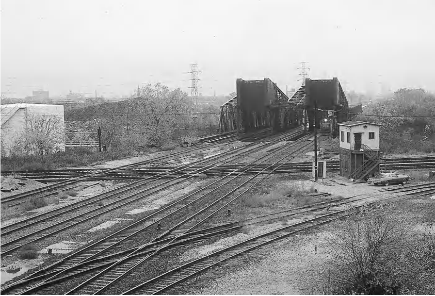
Figure 3-2 Western Avenue Bascule Bridges, Chicago, Illinois. This cluster consists of four independent single leaf Scherzer rolling lift bascule spans. The bridges were oriented in alternating opposing positions to allow them to be closer together. The bridges did not originally have machinery installed; although it was later put in, they no longer operate.
