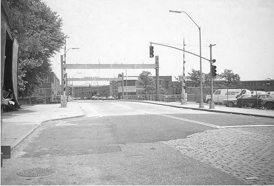
Figure 18-5 Rigid Barrier Gate. This gate is a solid box member. It is driven down the poles on the side of the roadway to block traffic. It has little impact-absorbing capacity and is thus best deployed on local streets with slow traffic, as shown.
