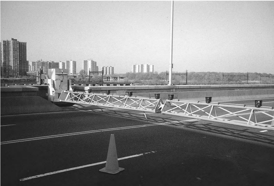
Figure 18-4 B&B Type Barrier Gate. The gate contains an annealed stainless steel rope, which, when the gate is engaged, blocking the roadway, stretches across from side to side. A vehicle impacting the gate causes the wire rope to stretch, elastically and plastically, absorbing the kinetic energy of the vehicle.
