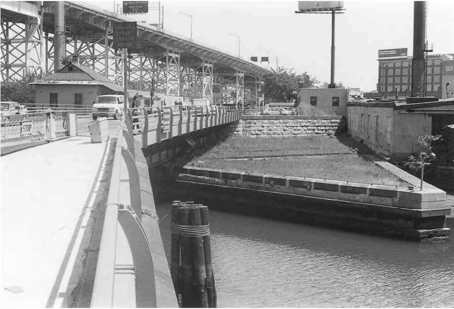
Figure 3-9 Borden Avenue Retractable Span, New York City. This bridge, built in 1904, is no longer operable, and its replacement with a fixed span is being considered.
