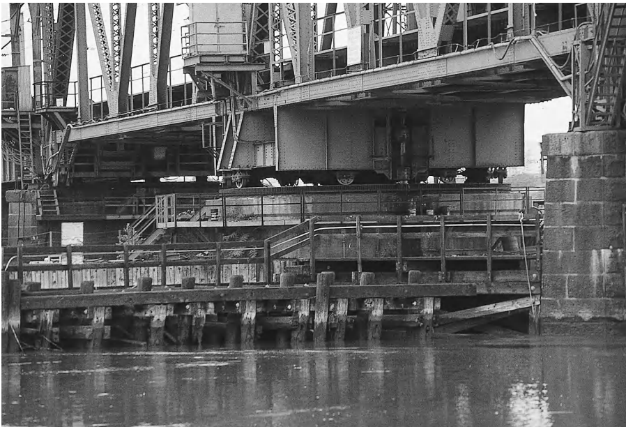
Figure 28-1 Swing Bridge Balance Wheels. The center bearing swing bridge superstructure requires stabilization when not on its live load supports. Balance wheels, spaced around a circular track, are used.
