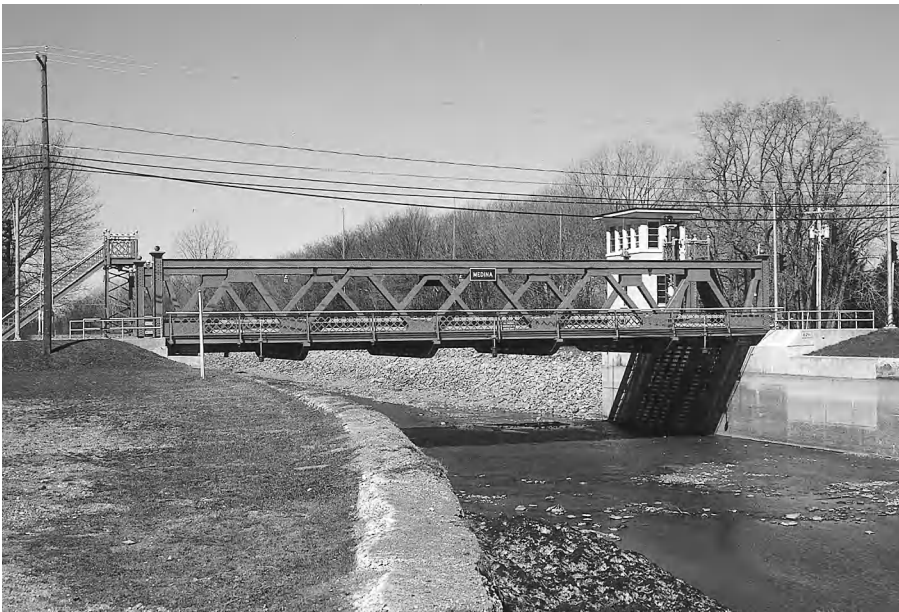
Figure 5-20 Erie Canal Bridge at Medina, New York. This is one of many similar vertical lift bridges on the New York State Barge Canal between Rochester and Buffalo, New York.
