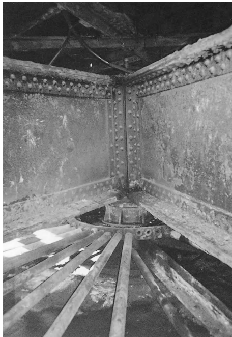
Figure 6-5 Swing Bridge Combined Bearing Center Pivot. This type of bearing supports part of the dead and live load; the rim bearing rollers support the rest.
