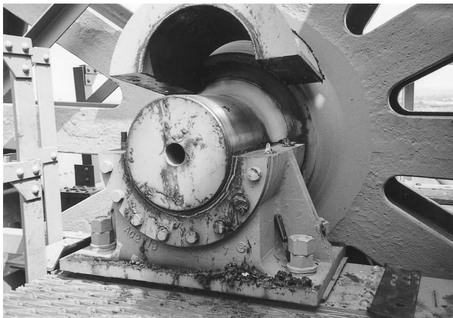
Figure 32-1 Inspection of Vertical Lift Bridge Counterweight Sheave Shaft. The shaft journal has been cleaned, and dye penetrant has been applied to test for cracks.
