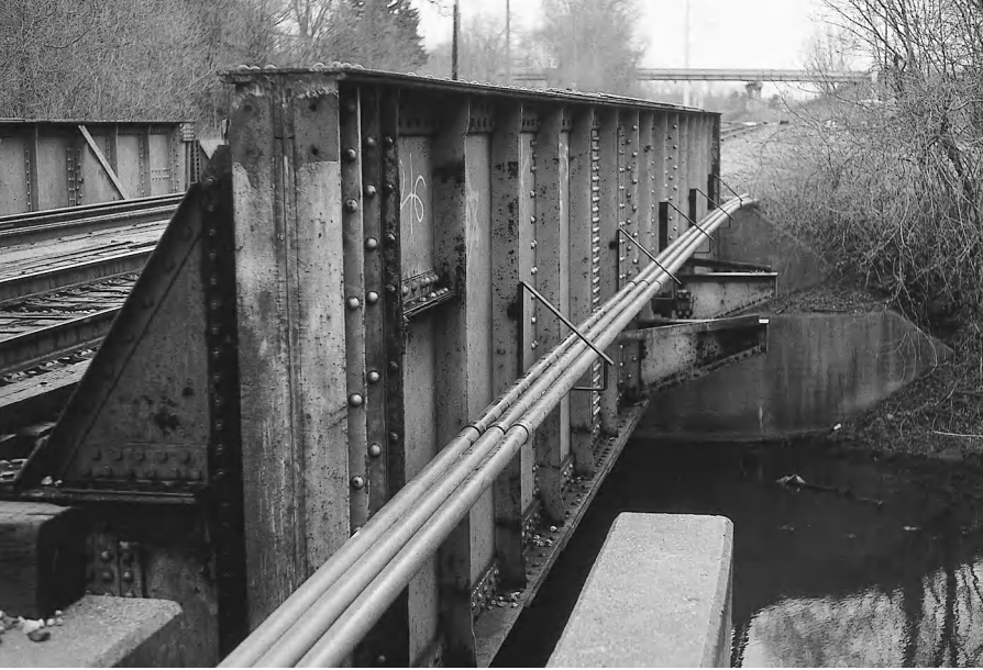
Figure 3-7 Former Vertical Lift Span. This bridge, over the Fox-Wisconsin Waterway at Portage, Wisconsin, was deactivated in approximately 1970 by having the machinery and towers removed.
