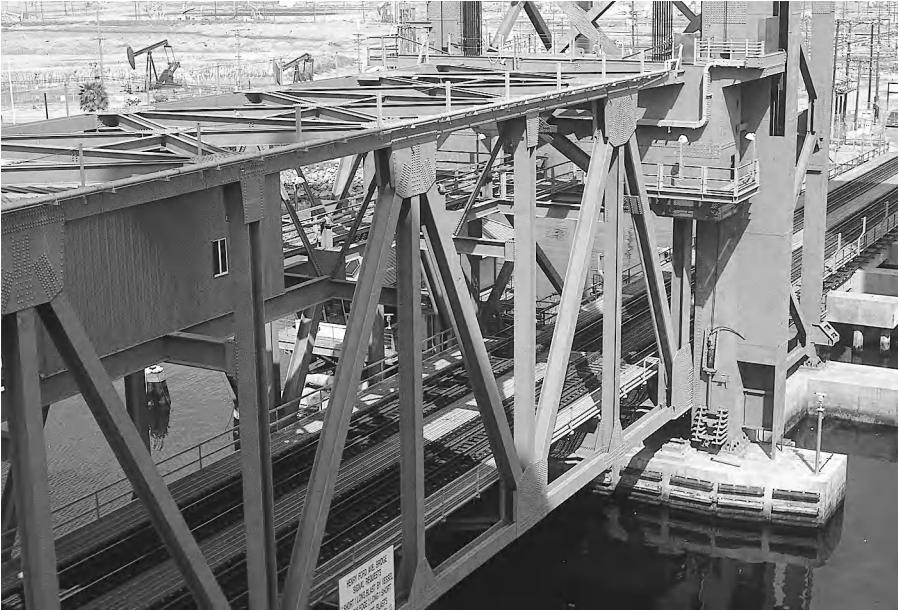
Figure 5-14 Span Drive Vertical Lift Bridge. This new example carries the Alameda Corridor onto Terminal Island. It has operating drums at each corner of the vertical lift span, powered via shafting from the central operator's and machinery house on the moving span.
