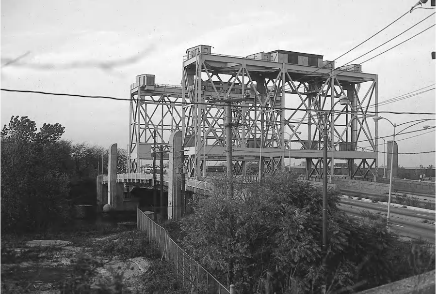
Figure 3-3 Western Avenue Vertical Lift Span, Chicago, Illinois. This bridge was constructed as a fixed bridge, then had machinery added; the machinery was then removed, and finally (after this photo was taken) the towers were removed.
