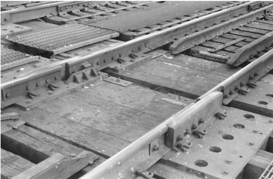
Figure 11-12 Miter Rails on Bascule Bridge. These rails are firmly fastened down onto the superstructure of the approach, in the foreground, and the bascule leaf, at the far side of the joint.
