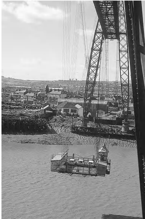
Figure 3-8 Newport Transporter, Wales. This type of device was once fairly common for providing transport across busy waterways, particularly at harbors. This example has been removed, and none of the type are believed to be in existence any longer.
