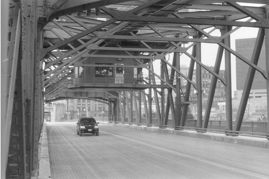
Figure 18-11 Vertical Lift Bridge Operator's House. This house provides a view of the roadway as well as the waterway for the bridge operator while he remains at his controls.
