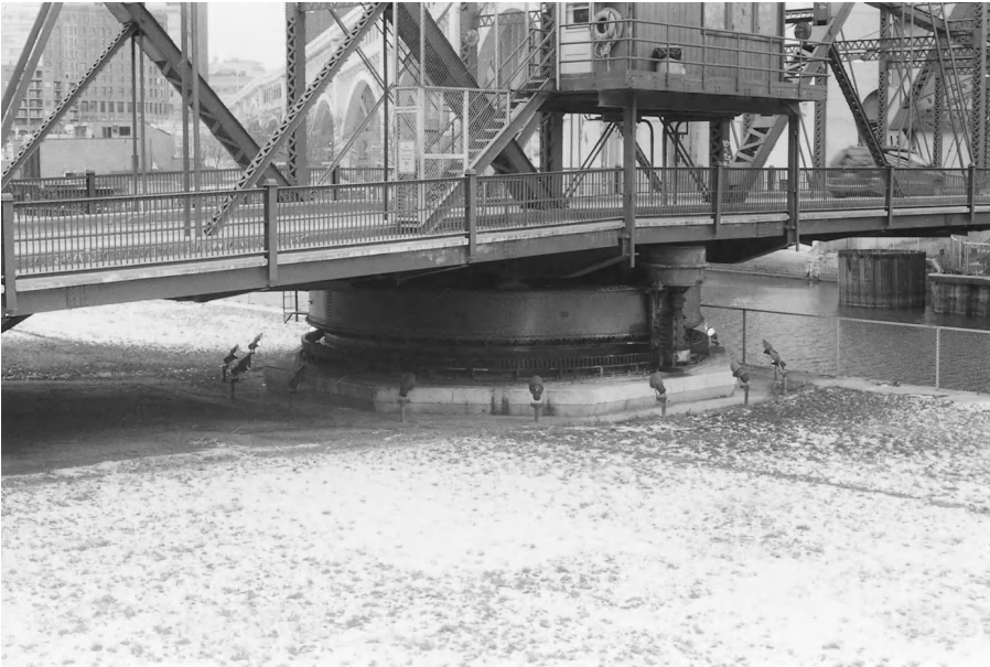
Figure 13-2 Swing Bridge Rim Girder. This swing span has had its girder and rollers replaced with a new unit assembly.
