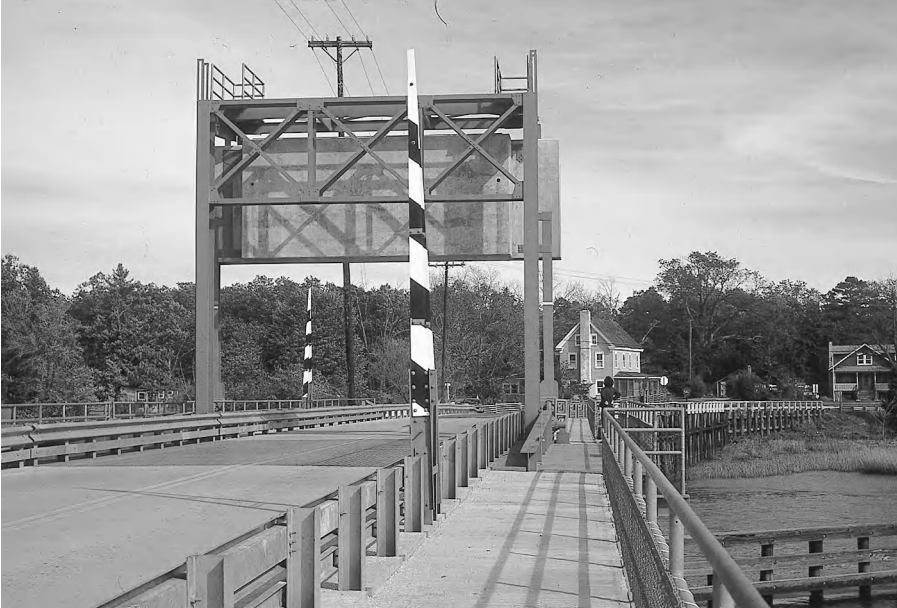
Figure 4-12 New Strauss Overhead Counterweight Bascule. In spite of evidence that this type of bridge is prone to failure, this example was constructed in the 1980s.
