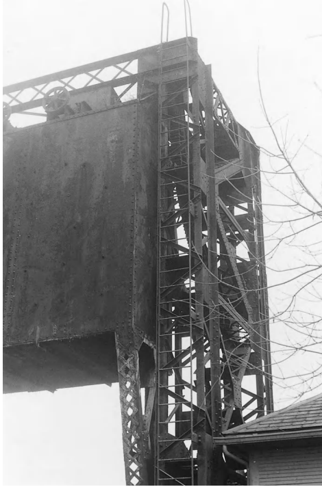
Figure 18-10 Chain Type Hand Drive. This bascule bridge is manually operated. The pulleys on top of the counterweight are fitted with chain loops, operated by persons on the ground, to raise and lower the bridge.
