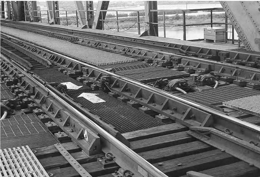
Figure 13-6 Miter Rails on Swing Bridge. These rails are firmly fastened down onto the superstructure of the approach, on this side of the arrows in the foreground, but are lifted mechanically on the end of the swing span, at the far side of the joint, to allow the bridge to be opened for navigation.
