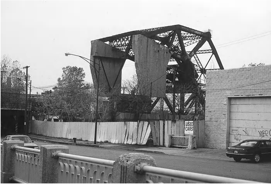
Figure 4-9 Bascule Split Counterweight. This arrangement allows a somewhat smaller superstructure to support the counterweight. It is frequently seen on heel trunnion bridges, as shown here; it is also used on rolling lift bridges.
