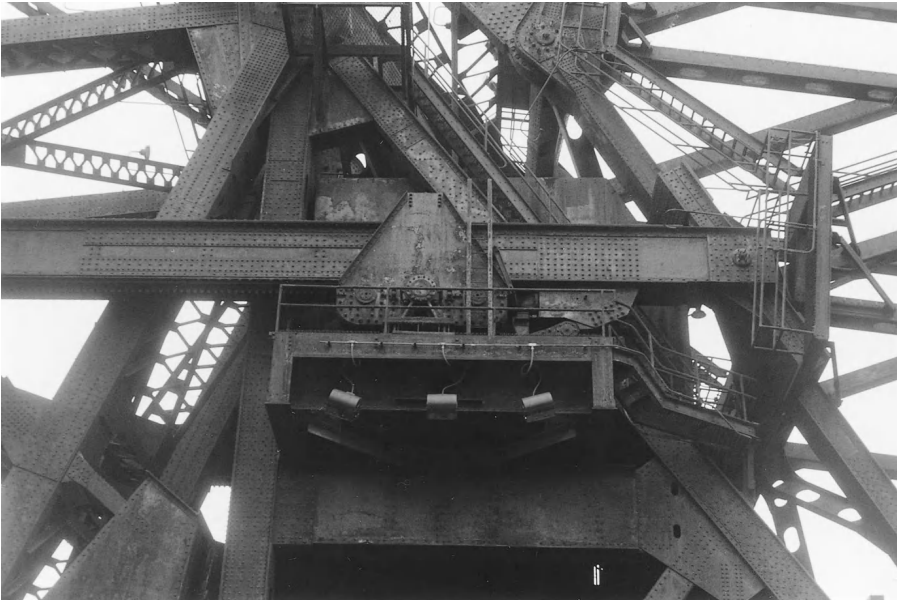
Figure 14-2 Operating Machinery for Heel Trunnion Bascule Bridge. The machinery, mounted on the A-frame supporting the counterweight, connects to the operating struts, one on each side of the bridge, via the carriers that engage the pinions to racks mounted on the underside of the struts.
