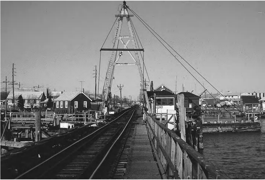
Figure 3-5 Shear Pole Swing Span. This bridge, on the south shore of Long Island, was replaced by a rolling lift bascule a few years ago.
