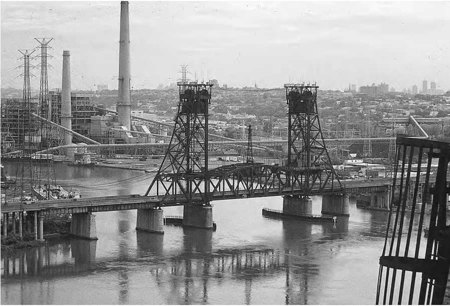
Figure 12-5 Vertical Lift Bridge Auxiliary Counterweight. The diagonal ropes extending from the mast reaching up from the center of the vertical lift span to the tower tops reach down and connect to weights hanging alongside the tower legs. These ropes pull up on the span when it is down, and down when it is up, compensating for the weight of the counterweight ropes.
