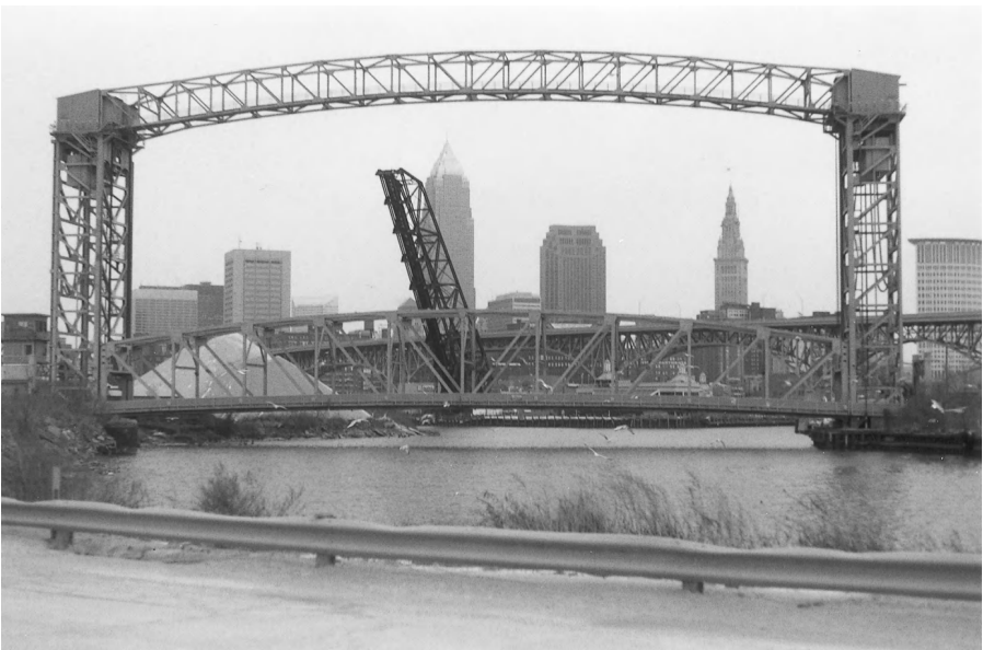
Figure 5-5 Tower Drive Vertical Lift Bridge. This type of vertical lift bridge is driven from the tops of towers. It usually has no machinery on the vertical lift span.
