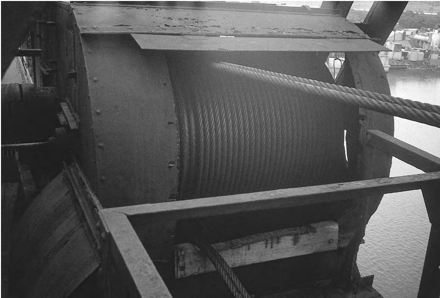
Figure 5-12 Operating Rope Drums for Waddell Type Vertical Lift Span. Each of four mechanically synchronized drums pulls in and plays out pairs of ropes as the bridge opens and closes. The ropes of each drum connect to the corresponding corner of the moving span. One pair extending to fixed connections at the top of the tower, called the uphaul ropes, and one pair extending and fixed to the tower base, called the downhaul ropes.
