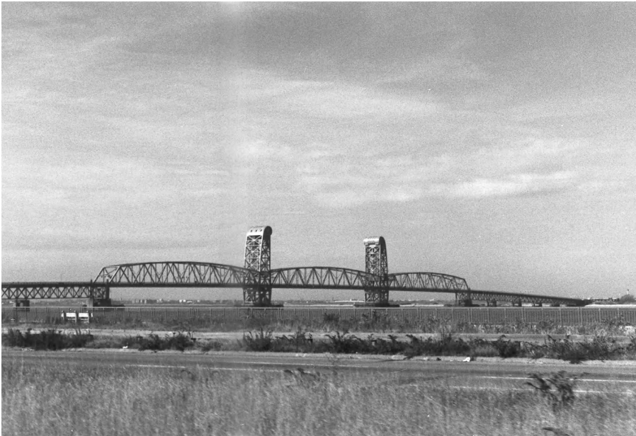
Figure 7-4 Marine Parkway Bridge. Efforts were made to produce an attractive superstructure on this through-truss vertical lift bridge.
