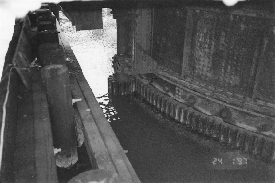
Figure 7-6 Swing Bridge with High Water. This movable railroad bridge, constructed at a low elevation, has its rack pinion, rack, and track partly submerged at each high tide.
