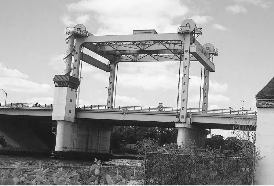
Figure 5-3 Span Tower Drive Vertical Lift Bridge. This example was built in the 1970s on the New Jersey shore. As this type is expensive to construct, it is less popular than other types.
