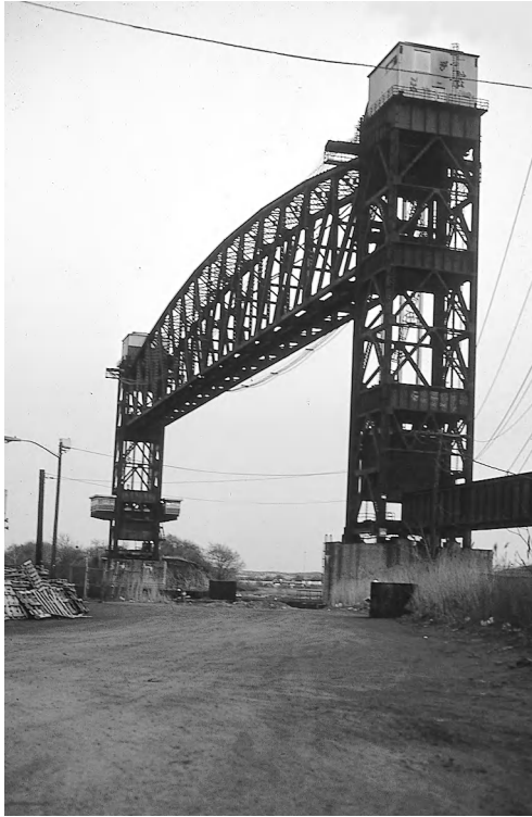
Figure 5-17 Tower Drive Vertical Lift Bridge. This particular vertical lift bridge is one of the world's longest. It spans Arthur Kill on a busy part of the New York harbor. This type of vertical lift bridge has no machinery on the moving span. Two separate drives, one on the top of each tower, operate the bridge. The drives must be coordinated to avoid tilting of the vertical lift span.
