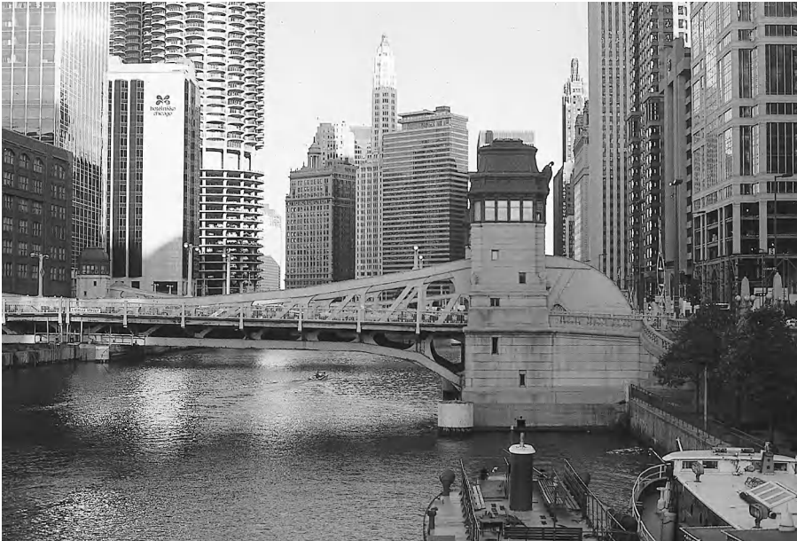
Figure 18-12 Ornate Operator's House. This house controls the La Salle Street Bridge over the Chicago River.
