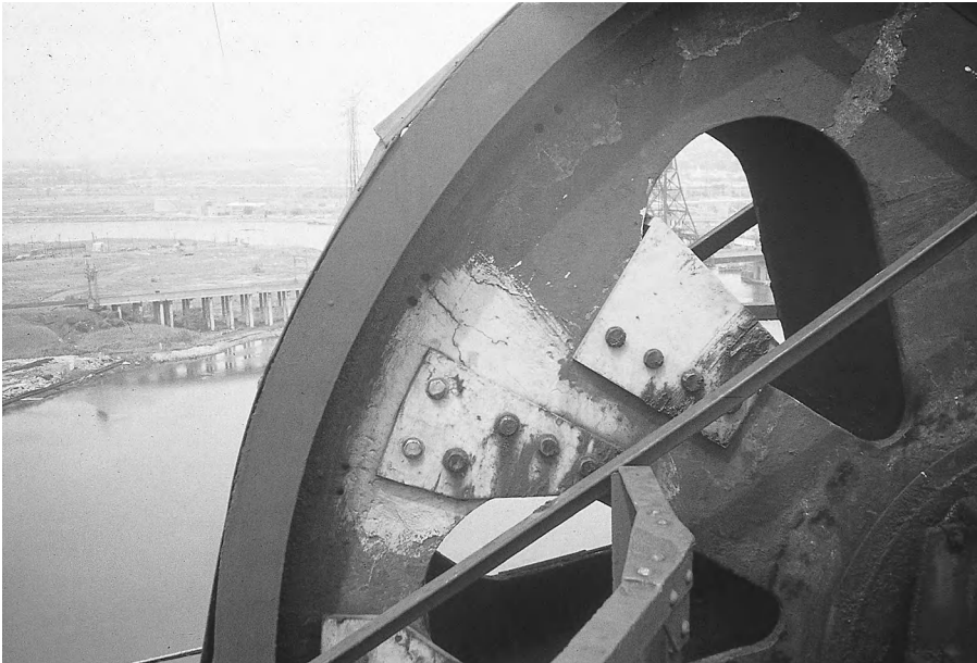
Figure 12-3 Vertical Lift Bridge Cracked Counterweight Sheave. The cracks in these sheaves appeared shortly after the bridge was put into service. The cracks were likely the result of manufacturing defects rather than any service conditions. The repairs shown have held up for about 20 years; it is questionable whether the repairs were needed at all.
