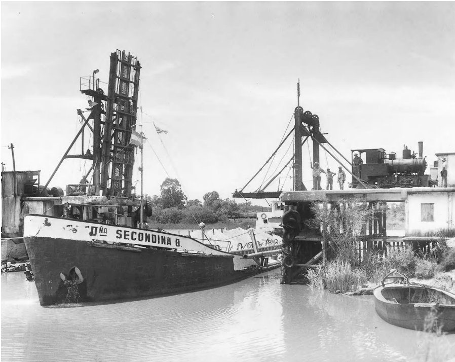
Figure 4-5 Combination Cable Stay—Simple Span Double Leaf Bascule Bridge. This bridge is located in Uruguay, on the north shore of the Rio de la Plata. It is about 70 years old, but is believed to still be in operation. The bridge is actually used as a loading dock for transloading sand from small railcars to the small ships or barges as shown in the photo. (Photo courtesy of Ron Ziel.)
