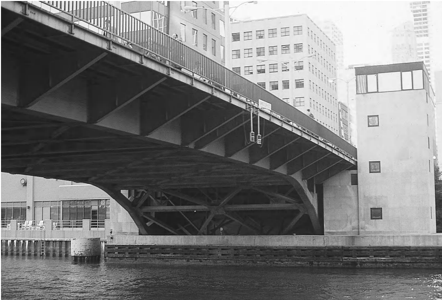
Figure 18-13 Modern Operator's House. This house controls the Madison Street Bridge over the South Branch of the Chicago River.
