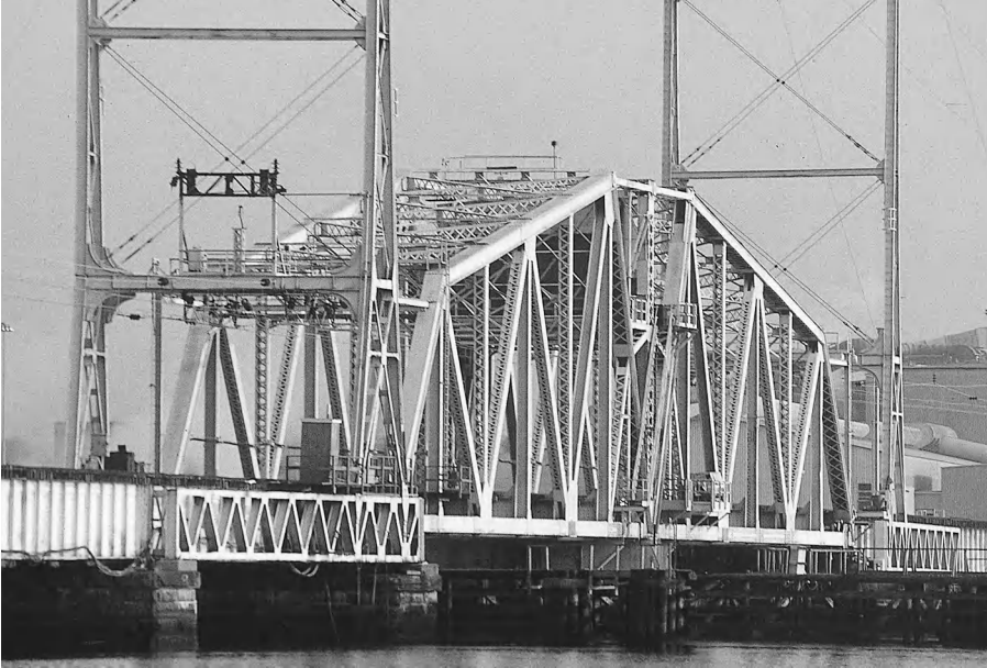
Figure 6-3 Large Center Bearing Swing Bridge. This bridge was one of the first successful large swing bridges not to be supported on a rim bearing.
