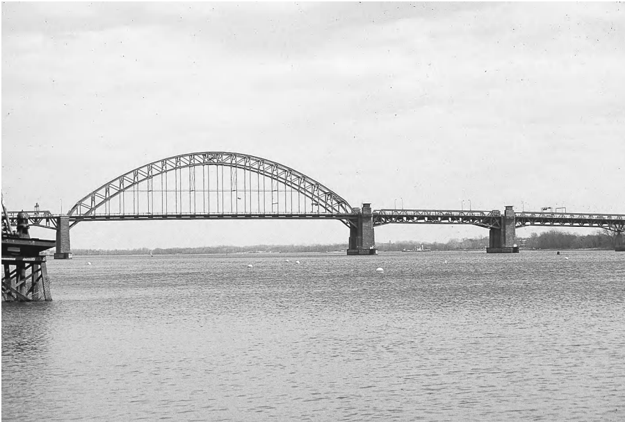
Figure 4-4 Double Leaf Rolling Lift Bascule Bridge. The bascule span is to the right of the arch bridge. It acts as an arch to carry live load, with compression joints at the upper chords at the center of the span.
