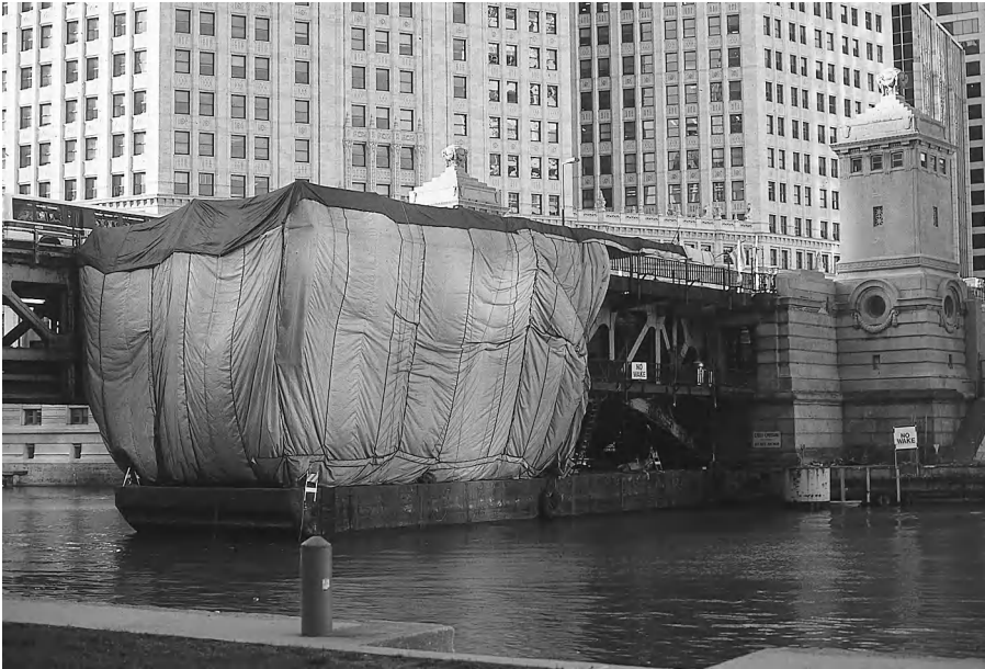
Figure 4-7 Michigan Avenue Bridge, Chicago, Illinois. This is a double leaf, double-deck twin bascule span. It has a total of eight deck sections. The western, or upstream, twin is under reconstruction here, so that the eastern twin is visible to the rear.
