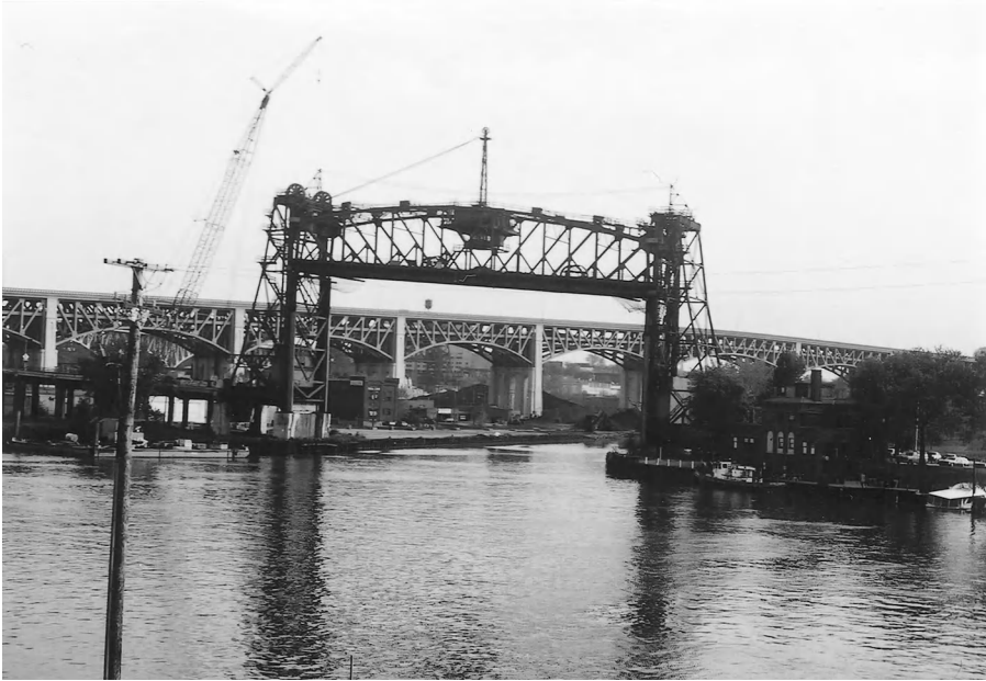
Figure 19-1 Vertical Lift Bridge under Repair. This bridge was found to have severely deteriorated counterweight sheave shafts. It was left in the raised position, supported on posts at each corner, while the counterweight ropes, sheaves, and shafts were replaced.
