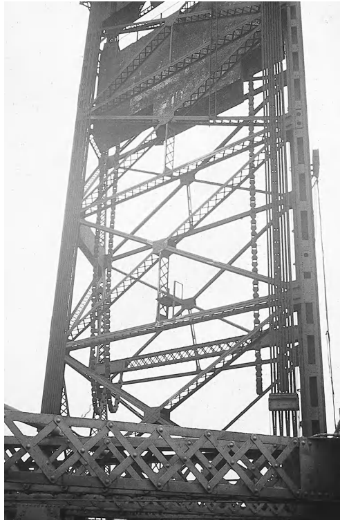
Figure 12-6 Balance Chains for Vertical Lift Bridge. These devices were once commonly used to compensate for the weight of counterweight ropes passing over their sheaves as the bridge operated.
