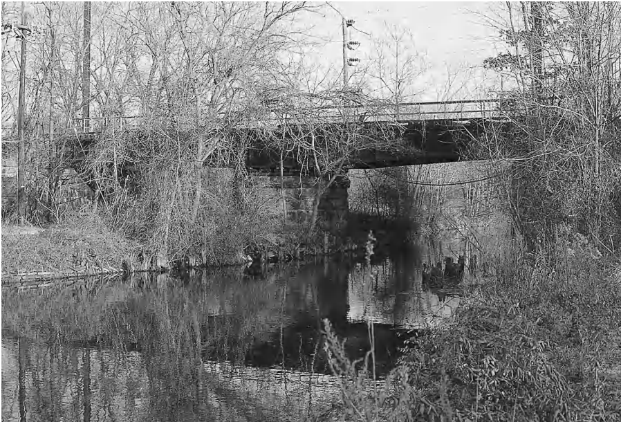
Figure 7-7 Swing Bridge over Delaware and Raritan Canal. This bridge, built in 1905, has probably not opened since the canal was closed in the 1930s. The canal is in a small valley, and rather than build a single movable span with additional approach spans or fill, a symmetrical swing span was constructed, although only one arm is over water. The canal towpath passes under the second arm of the swing span.
