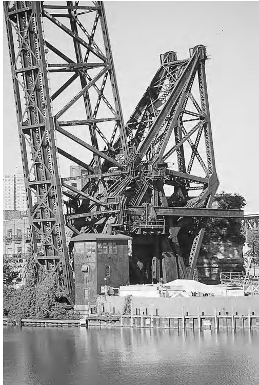
Figure 14-1 Operating Strut for Heel Trunnion Bascule Bridge. This is the most typical operating strut arrangement. The strut is pinned to the heel portal of the moving span, and connected to drive machinery resting on the A-frame tower supporting the counterweight.
