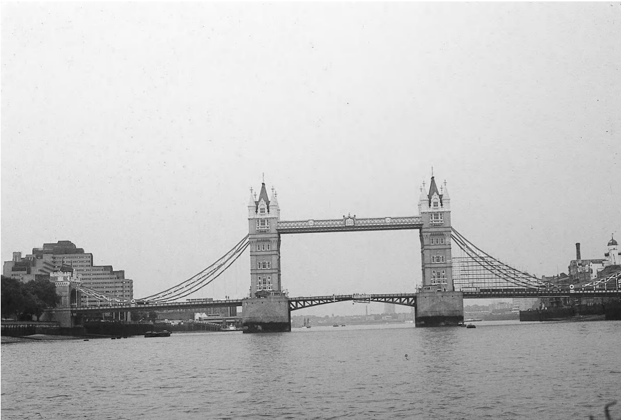
Figure 2-6 Tower Bridge, London, England. This bridge is a combination suspension bridge and double-leaf bascule. The upper cross member above the bascule span is necessary to sustain the longitudinal tension of the suspension cables, which are actually iron bars.
