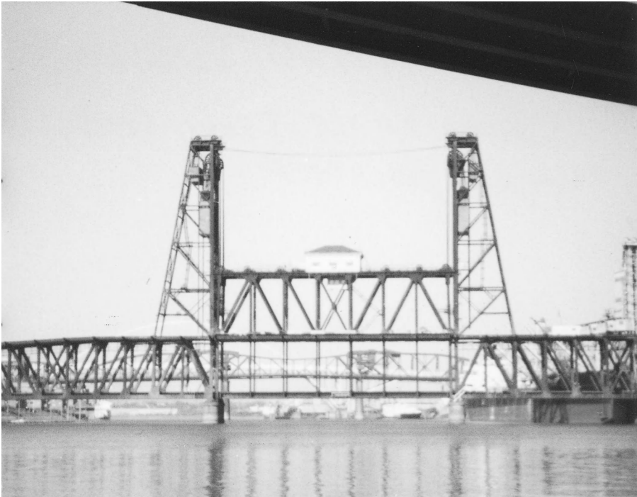
Figure 5-9 Double-Span Drive Vertical Lift Bridge. This is the Steel Bridge in Portland, Oregon. The lower deck can lift while the upper deck remains stationary, or both decks can lift.
