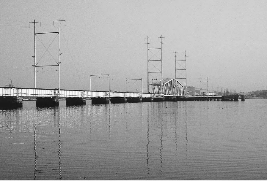
Figure 9-1 Raritan Bay. This location is typical of many in placing a movable bridge in danger of being struck by vessels, particularly if high winds are prevalent.
