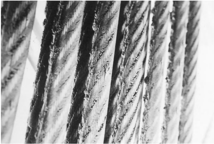
Figure 12-2 Worn Counterweight Ropes for Vertical Lift Bridge. The rope wires have large wear spots. There are many broken wires that can be seen. These ropes were replaced as a result of these findings.
