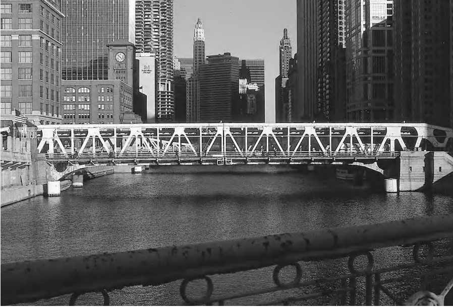
Figure 4-17 Double Deck Double Leaf Bascule. This bridge carries Wells Street and pedestrians on the lower level, and the CTA elevated rapid transit line on the upper level.
