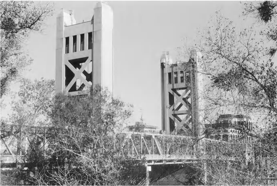
Figure 5-22 Tower Bridge, Sacramento, California. This bridge is an unusual span drive type, in that efforts have been made to produce an architecturally pleasing effect with the bridge superstructure. This is one of the few span drive vertical lift bridges with any sheathing on the towers, for instance.
