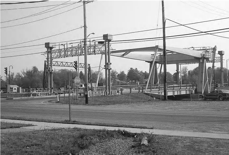
Figure 9-2 Culvert Street Bridge, Phoenix, New York. This is one of the few “European”-type heel trunnion bascule bridges constructed recently in the United States. It has a few unique features, including a multigirder redundant superstructure, isolation of live load from the operating machinery, and machinery mounted on the counterweight. The warning gates are adjacent to the cross-street intersection.
