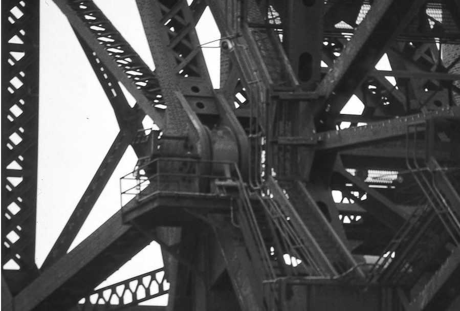
Figure 31-2 Bascule Bridge Trunnion Bearing. This bearing supports one side of the counterweight of a large heel trunnion bascule bridge. The size of the bearing can be gauged by the handrail below it.
