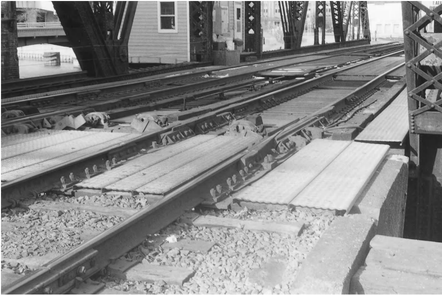
Figure 16-1 Miter Rail Locks on Swing Bridge. These miter rails are of the cast “Conley” type. Each movable miter rail has a separate electrical lock that trips when the moving rail is fully engaged with its mate on the approach span.
