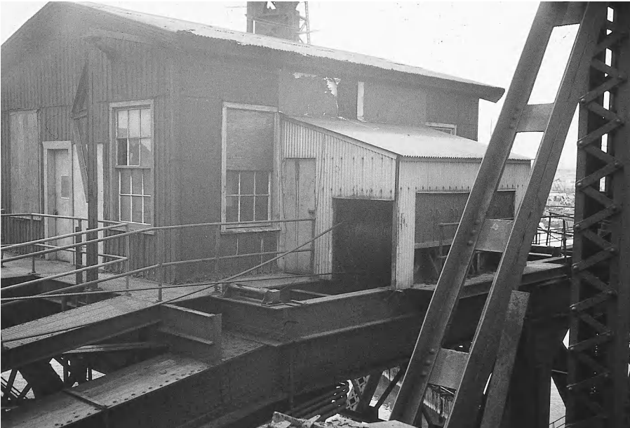
Figure 17-19 Machinery House. This house protects the main drive machinery of a Waddell vertical lift bridge. The bridge is operated from elsewhere.
