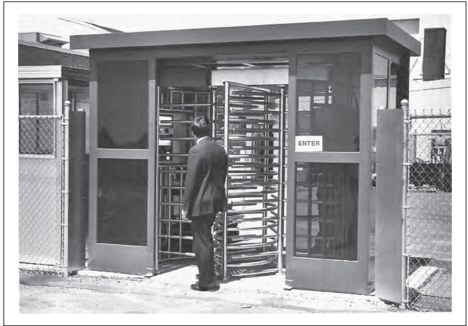
FIGURE 22-26 Dual rotor video turnstile access control system
