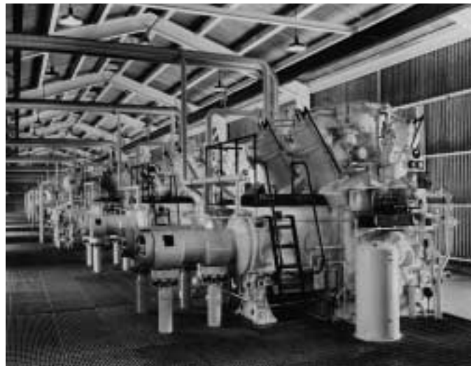
Figure 14-33. Gas engine driven parallel compression cylinders in process gas plant service. Note that the front side of gas engines are on the right with high-pressure compressor cylinders extending horizontally left. Also note the suction side pulsation drums on top of compressor cylinders, mid-way. (Used by permission: Cooper-Cameron Corporation, Reciprocating Products Division.)
