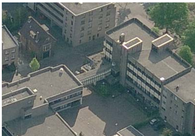
Figure 5, Oblique image showing a corridor connecting two buildings, hanging free in space.
