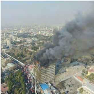
Figure 3: Aerial view of the building during the fire on January 19, 2017, showing the shopping mall at rear.
