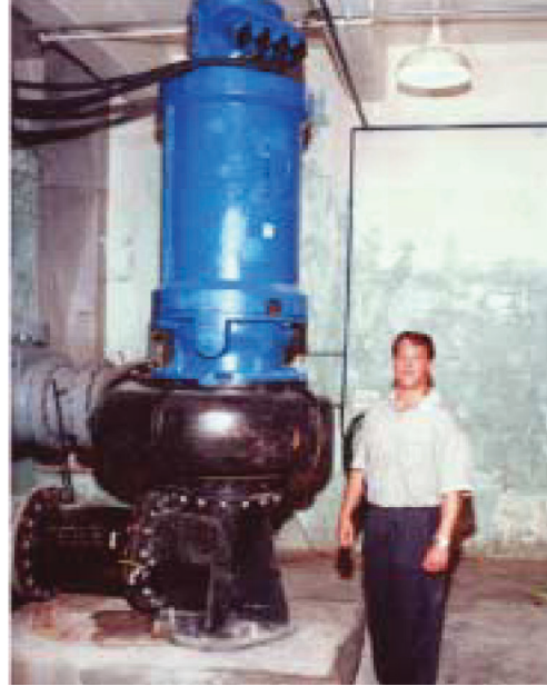
Figure 4. Dry-Well Submersible.
