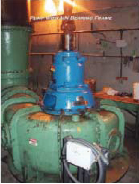
Figure 14. New POA in Place.
