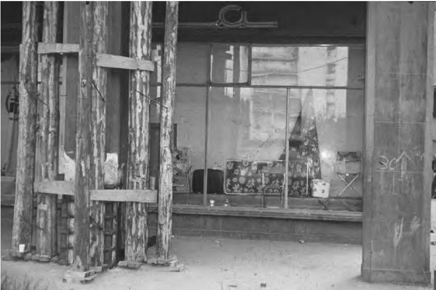
Figure 12.16 Timber propping of a damaged column; Bucharest, Romania (1977).
