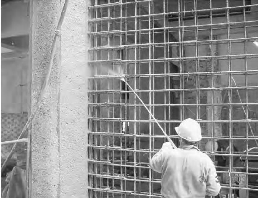
Figure 15.1 Dedusting and wetting of the old concrete and reinforcement at the complex of the Army Pension Organization (Athens).
