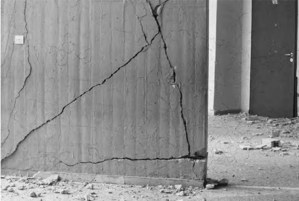
Figure 11.15 Shear wall failure: Kalamata, Greece (1986) failure to shear and in parallel to bending.
