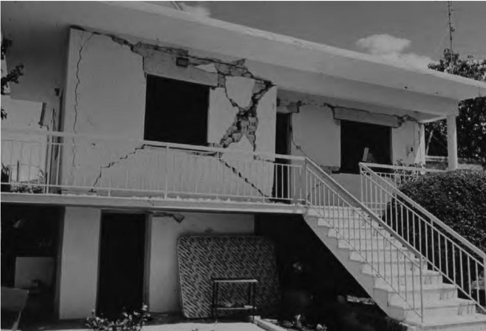
Figure 11.31 Damage to masonry walls: Kalamata, Greece (1986).
