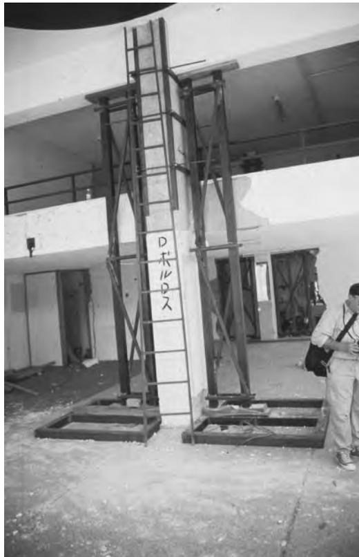
Figure 12.18 Steel profile props for the repair of a damaged column; Kalamata, Greece (1986).
