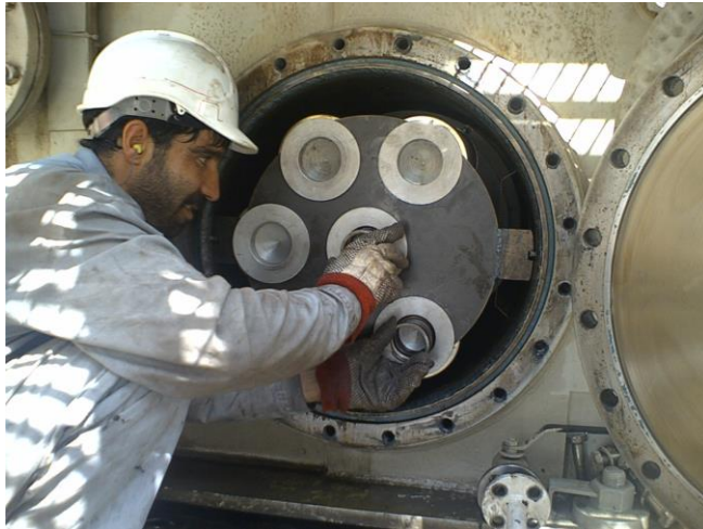
Figure 29: Disposable Lube Oil Filters (Picture Belongs to Unit 106 of phases 2&3 of S.P.G.C.)
