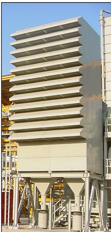
Figure 6: A Filter House Containing Self-Clean Filter (Picture Belongs to Unit 106 of Phase 2&3 of S.P.G.C.)
