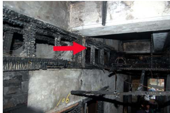
Fig. 4 Relative location of transom window for room 106 and hall ceiling.
