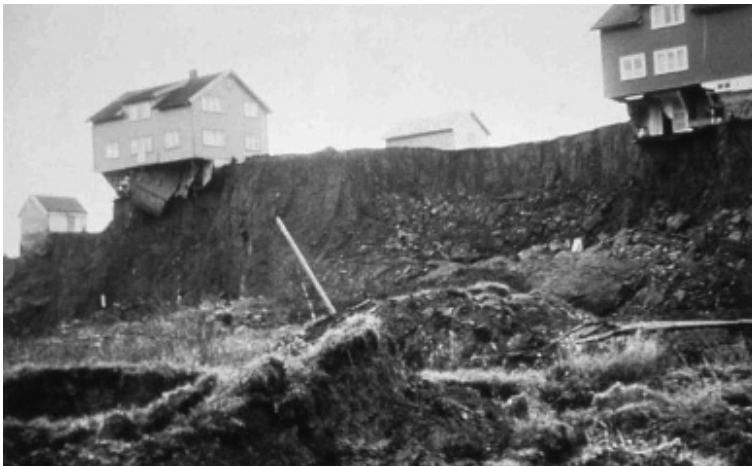
Figure 5.27 Damage observed following the Rissa quick clay flow-slide (photo: Norwegian Geotechnical Institute – NGI).
