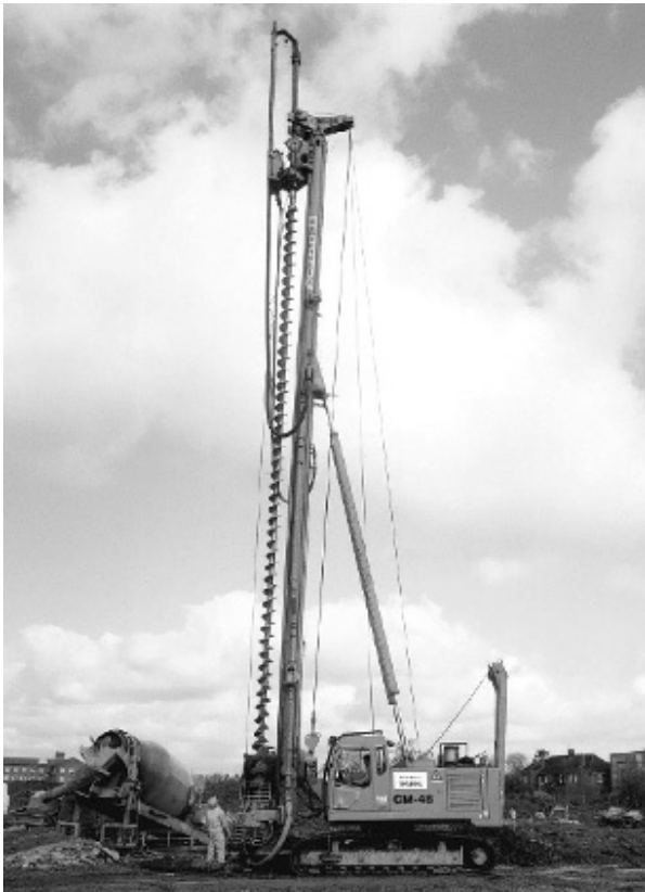
Figure 9.3 Pile installation: non-displacement piling (CFA) (image courtesy of Cementation Skanska Ltd.).
