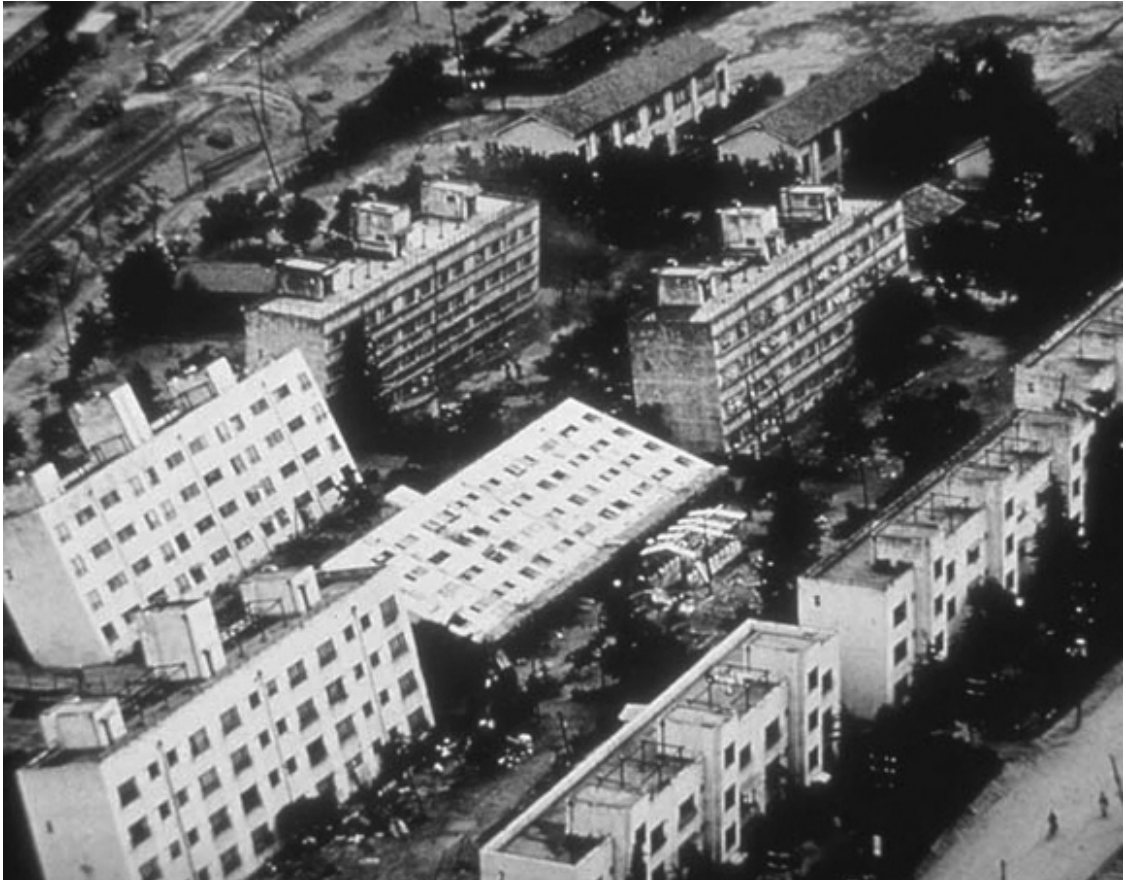
Figure 3.10 Foundation failure due to liquefaction, 1964 Niigata earthquake, Japan.
