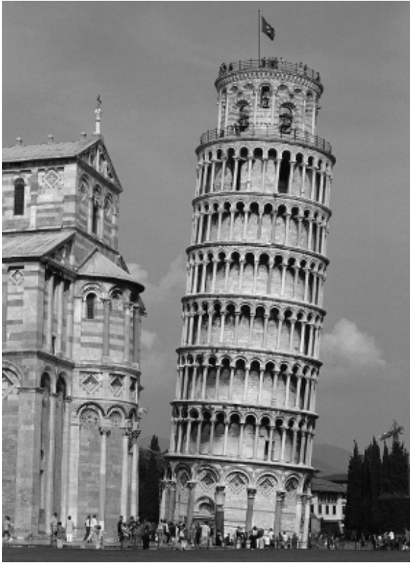
Figure 10.3 The ‘Leaning Tower of Pisa’: an example of excessive tilt (image courtesy of Guy Vanderelst/Photographer’s Choice/Getty Images).
