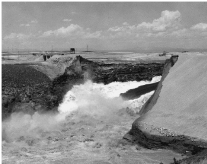
Figure 2.18 Failure of the Teton Dam, 1976 (photo courtesy of the Bureau of Reclamation).
