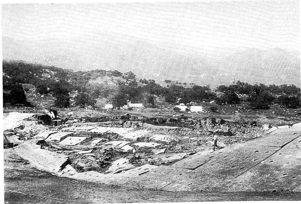
Figure 1.5 Liquefaction failure of Sheffield Dam following the 1925 Santa Barbara earthquake (K. Steinbrugge collection; courtesy of EERC, Univ. of California).
