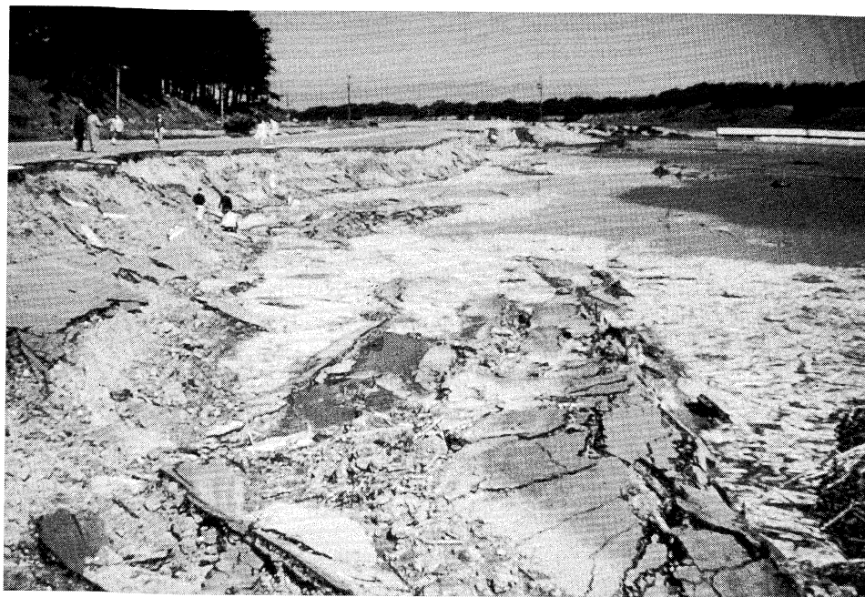
Figure 9.1 A small flow slide along the shore of Lake Merced in San Francisco in 1957 (photo by M. Bonilla; courtesy of USGS).
