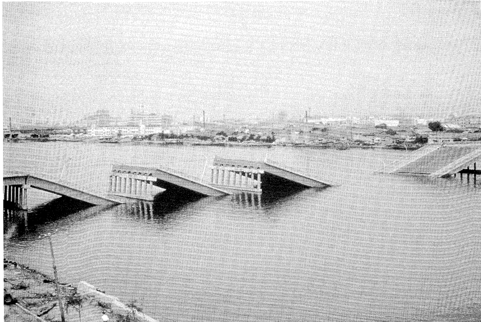
Figure 1.9 The Showa Bridge following the 1964 Niigata earthquake. Lateral spreading caused bridge pier foundations to move and rotate sufficiently for simply supported bridge spans to fall (courtesy of USGS).
