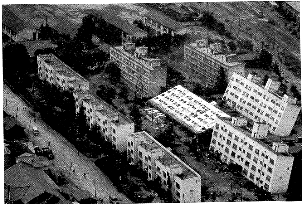
Figure 1.6 Liquefaction-induced bearing capacity failures of the Kawagishi-cho apartment buildings following the 1964 Niigata earthquake (courtesy of USGS).
