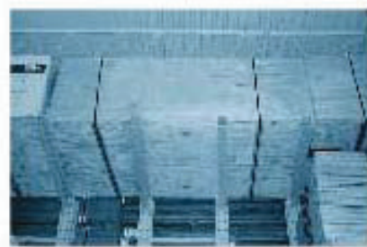
For safety purposes these cantilevered beams that support sheets of plywood must be designed for both strength and a restricted amount of deflection.
