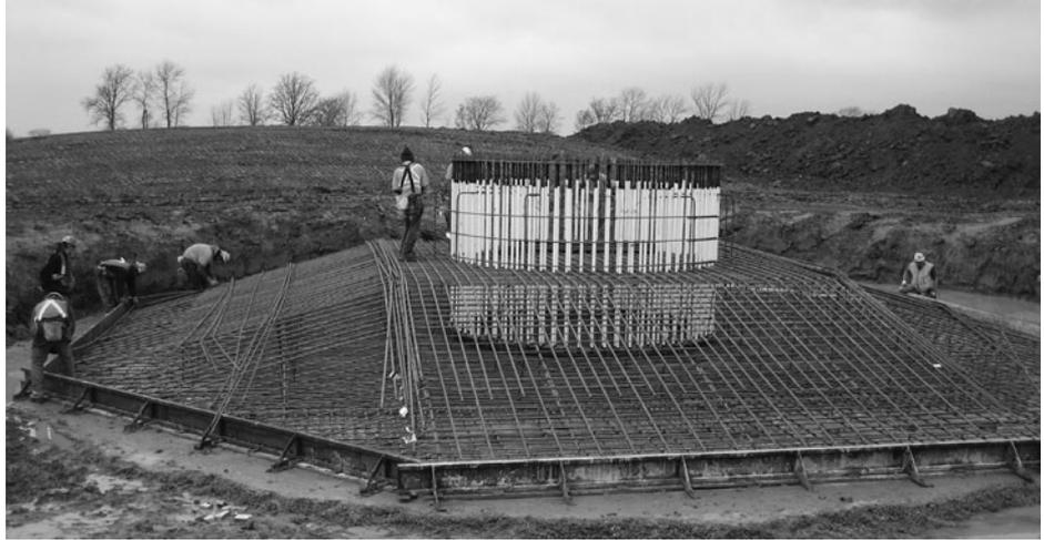
*This wind turbine foundation was installed at Invenergy's Raleigh Wind Energy Center in Ontario, Canada to support a 1.5 MW turbine with an 80 meter hub height. It consists of 313 cubic yards of 4350 psi concrete, 38,000 lbs of reinforcing steel and is designed to withstand an overturning moment of 29,000 kip-ft. Each of the 140 anchor bolts shown in the photo is post-tensioned to 72 kips.*
