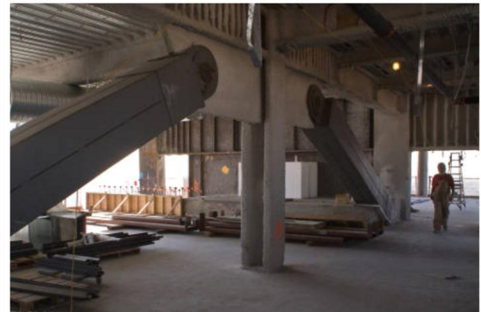
Buckling-restrained braces at 28 th floor (transition from hotel to condo)
