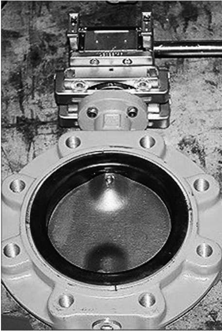
Figure 10-6. Butterfly Valve with Mechanical Locking Device. (Courtesy of Netherlocks, Holland)
