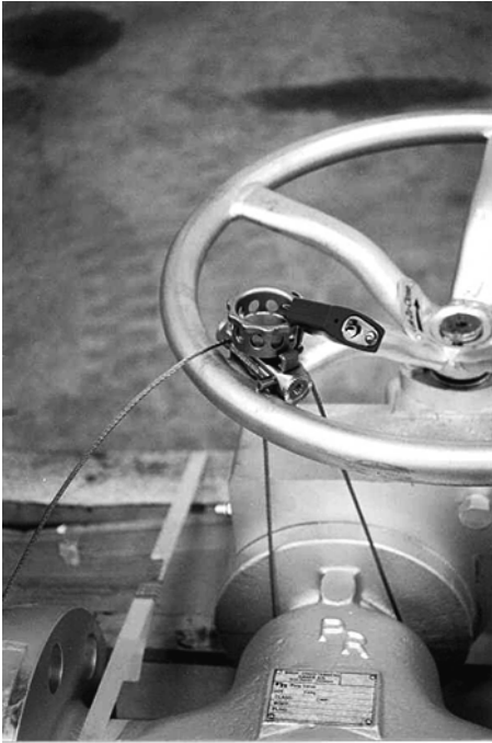
Figure 10-1. Wire on Gearbox with Independent Padlock Butt Weld. (Courtesy of Netherlocks, Holland)
