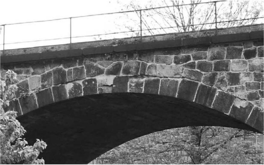
**Fig. 6-12.** Sliding spandrel wall
