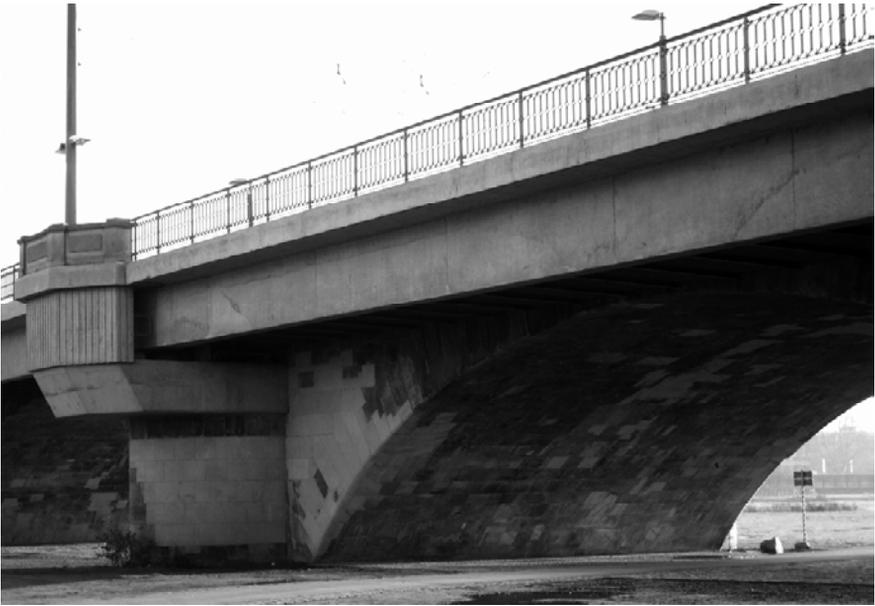
**Fig. 6-28.** Example of arch bridge width increase by an attached beam
