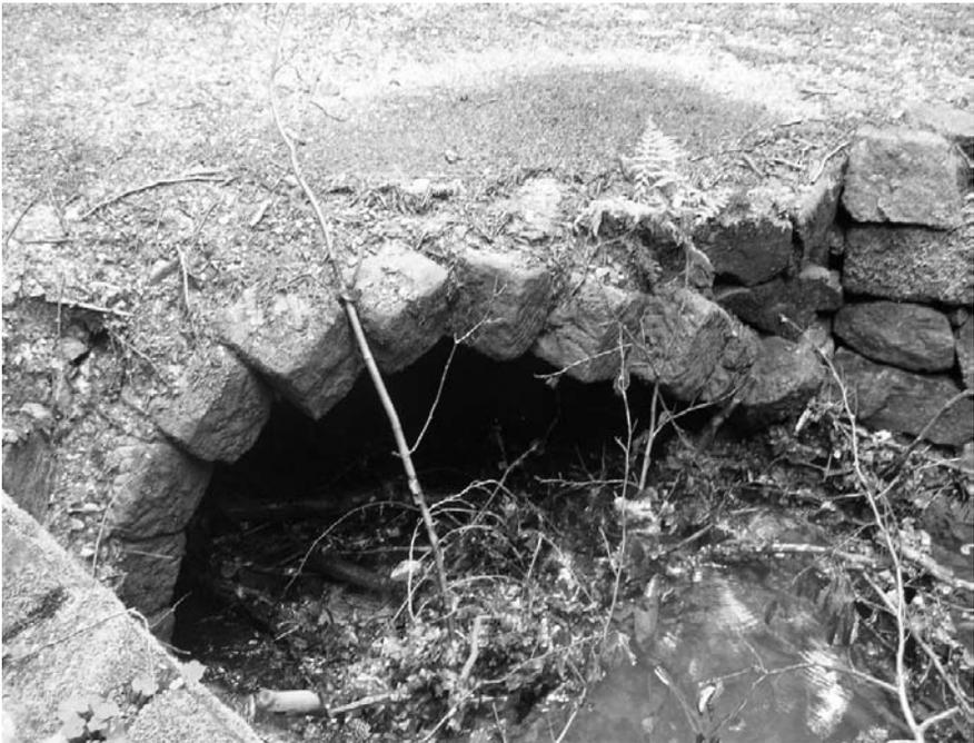
**Fig. 1-34.** Example of protruding stones to achieve skewness
