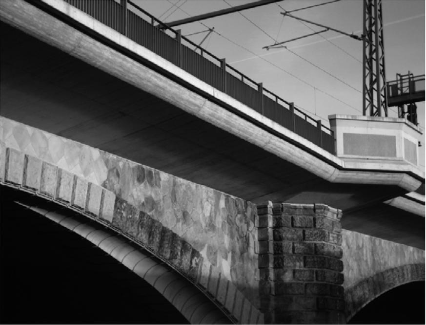
**Fig. 6-19.** Example of arch bridge width increase by a concrete slab
