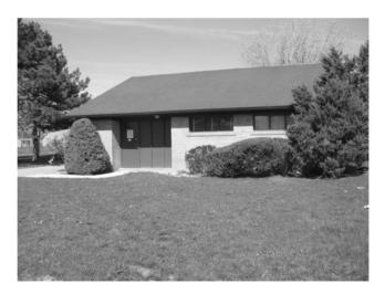
Figure 9.3 A covert electrical substation.
