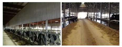
Fig. 11. Baffles installed in a cross-ventilated (left) and a tunnel-ventilated (right) retrofit barn.
