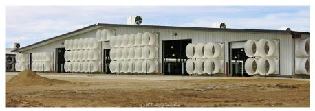
Fig. 13. A hybrid ventilation system with fans at the end-wall for summer ventilation and cupola fans for winter ventilation.
