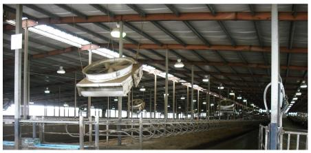
**Fig. 9.** Hybrid-ventilated barn with cyclone fans over the stalls to provide fast-moving air in the stall microenvironment and a closed ridge with a cupola system.
