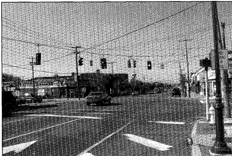
Figure 19.30: A Typical Span-Wire Signal Installation
