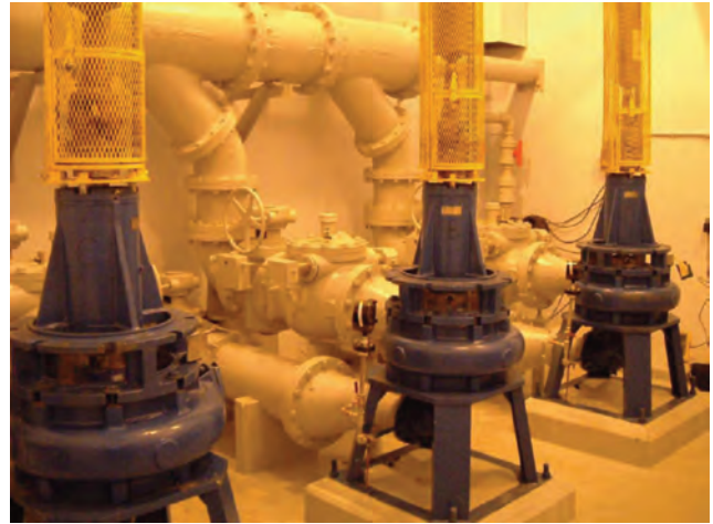
Figure 41. Sewage Pumps Mounted on Fabricated Stands.
