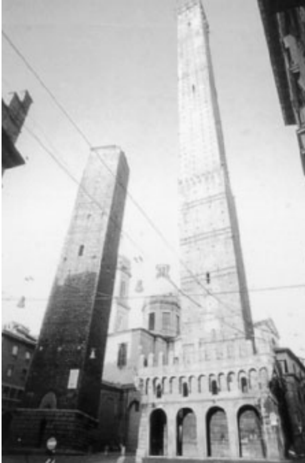
Figure 1.2 Tilting of Garisenda Tower (left) and Asinelli Tower (right) in Bologna, Italy (Courtesy of Braja M. Das, Henderson, Nevada)
