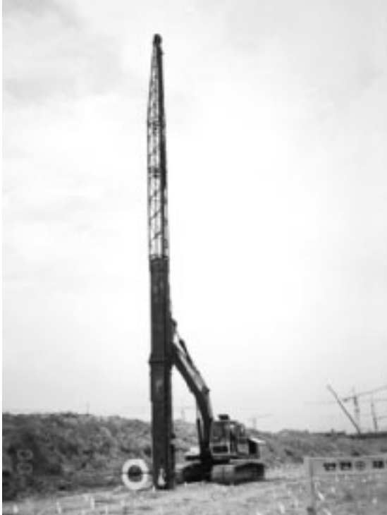
Figure 11.38 Installation of PVDs in progress (Courtesy of E.C. Shin, University of Inchon, South Korea)
