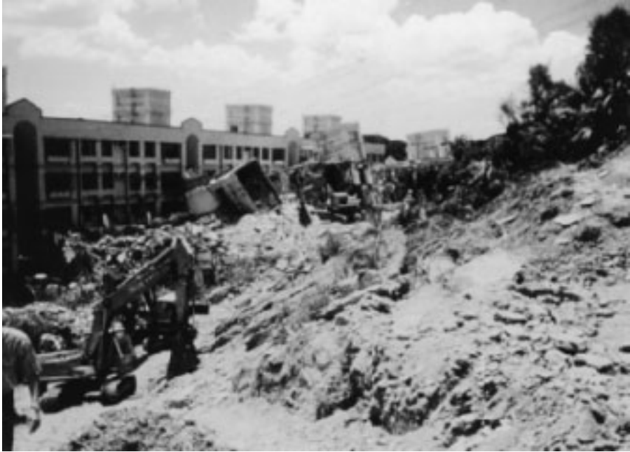
Figure 15.2 Soil and rock “fall” in a slope (Courtesy of E.C. Shin, University of Incheon, South Korea)
