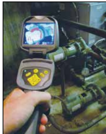
FIGURE 2. Problems such as overheated bearings can be diagnosed with a thermal imaging camera, which provides an alternative to direct-contact temperature sensors, especially for components that may be hard to reach, inaccessible or potentially hazardous
