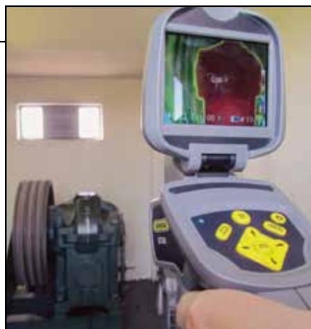
FIGURE 5. When operators are able to monitor the thermal profile of equipment and systems using a remote monitoring technique, they can plan for the most appropriate and timely intervention to address a deteriorating condition
