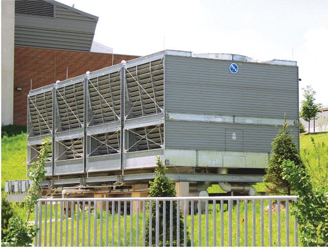
**Photograph 2: Crossflow Cooling Tower Installation**
