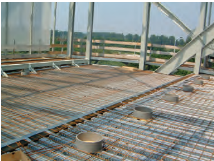
Composite slab used in the auditorium area
