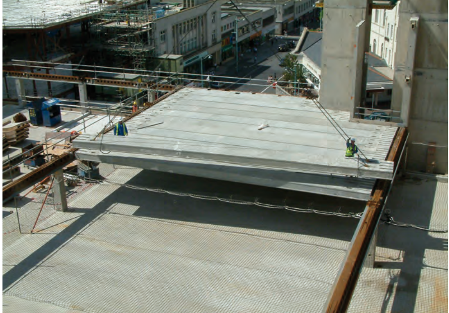
Figure 3.15 Precast concrete units placed on non-composite beams
