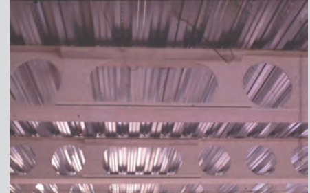
Figure 2.2 Elongated openings in beams with horizontal stiffeners
