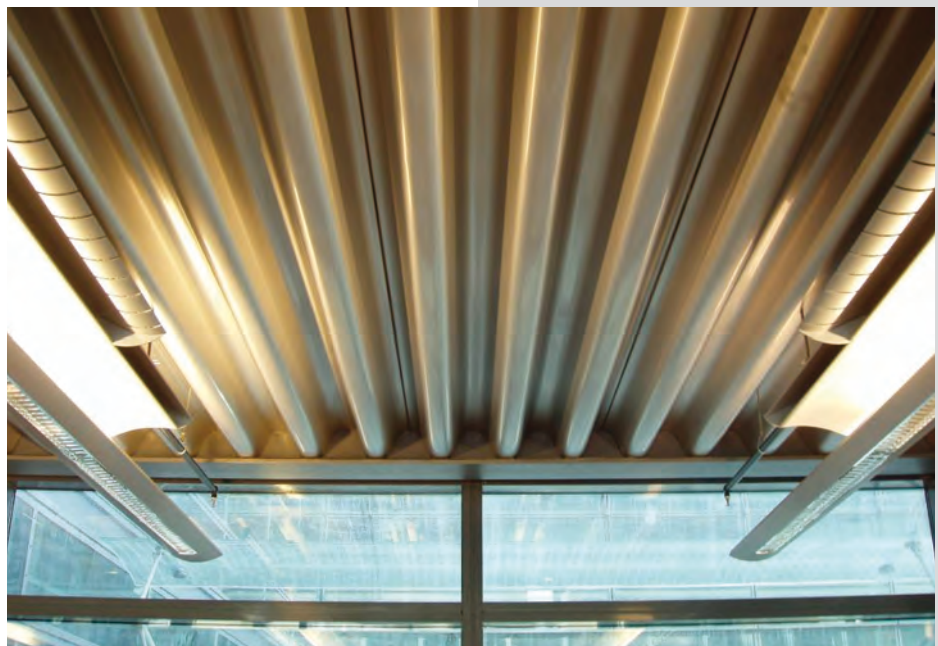
Figure 2.4 Stainless steel composite decking used at the Luxembourg Chamber of Commerce Vasconi Architects
