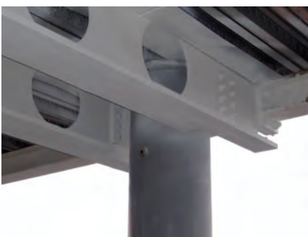
Tubular column connection
