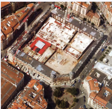
Top view of the construction site (May 2006)
