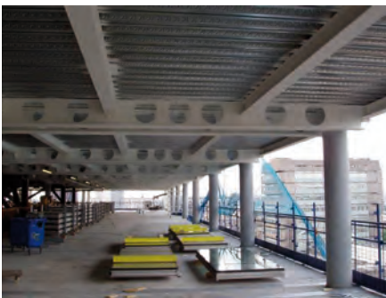
Pairs of cellular beams
