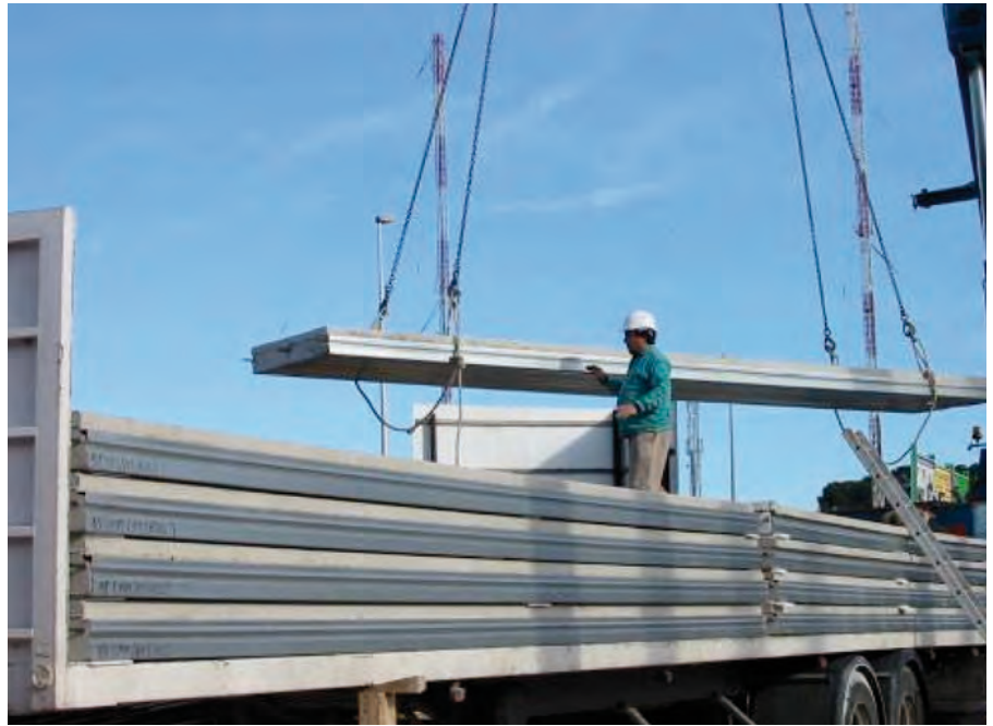
Figure 4.2 Delivery of Cofradal 200 to site
