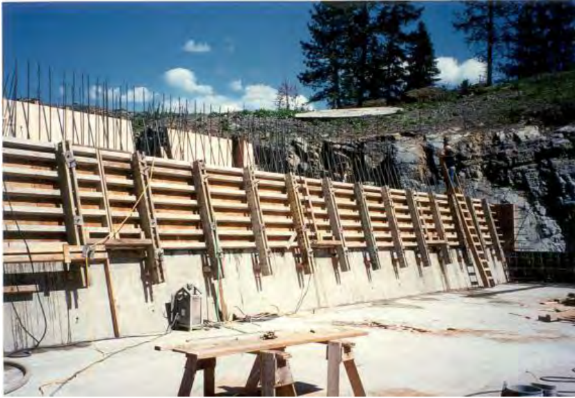
FIGURE 8.5 Monolith dam construction cantilevered form.
