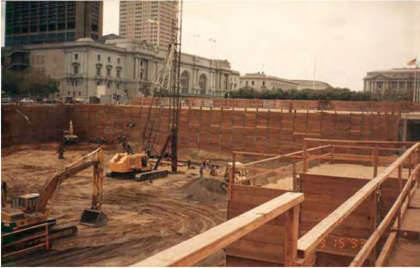
FIGURE 6.6 Lagging system in place.
