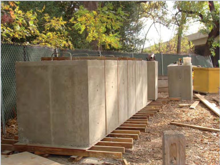
FIGURE 9.CS7 Counterweights (deadmen) on casting bed.
