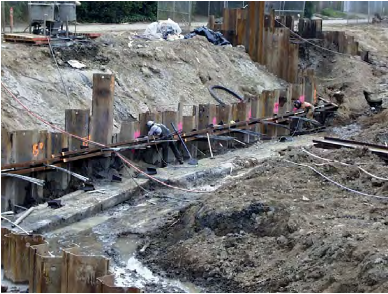
FIGURE 7.10 Double channel water system with tiebacks.
