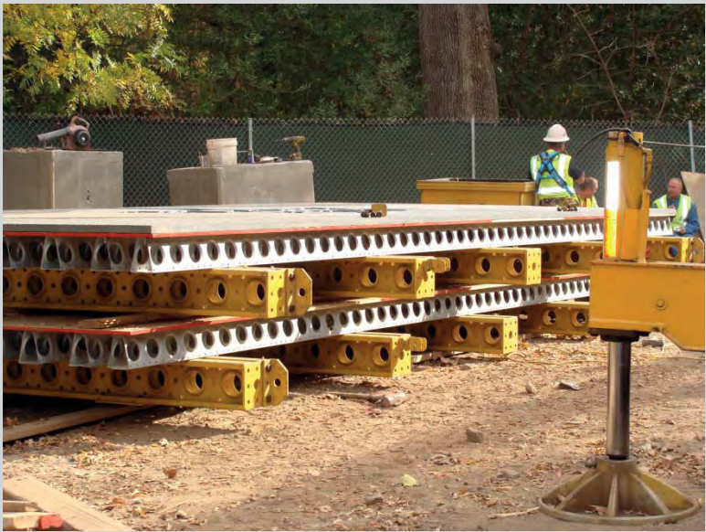
FIGURE 9.CS8 Prefabricated wall forms with form liner.
