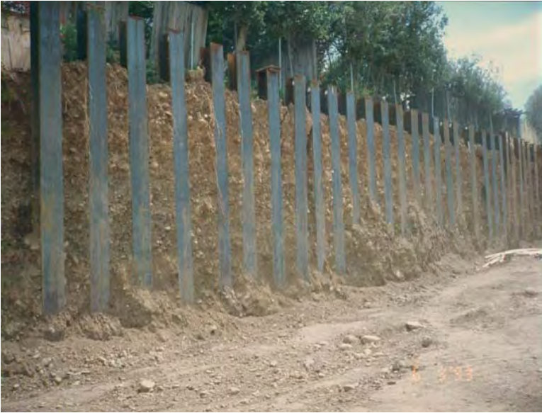
FIGURE 6.19 Soldier beams without lagging.
