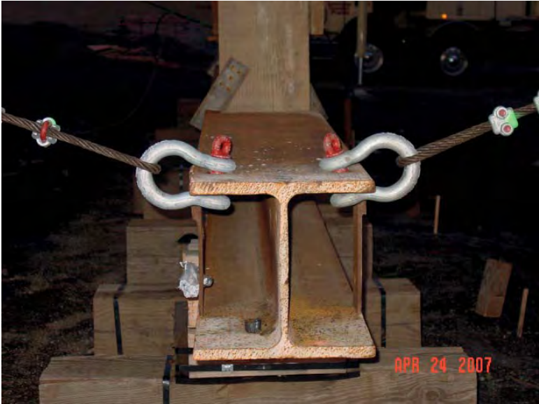
FIGURE 11.28 Longitudinal bracing connected to bottom cap.
