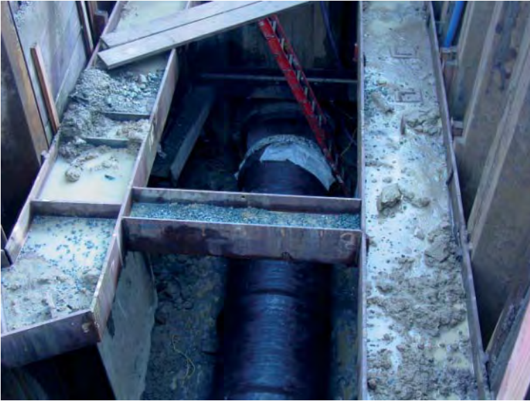
FIGURE 7.17 Strut supporting walers.
