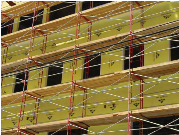
FIGURE 4.4 Scaffolding used for building construction.
