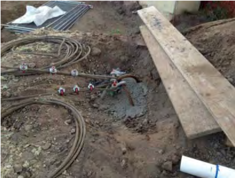
FIGURE 11.22 Drilled pile anchor.
