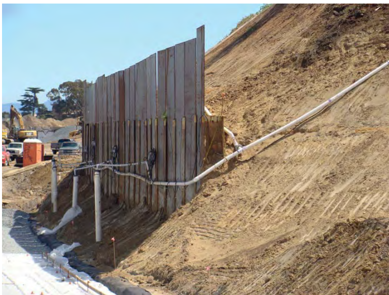
FIGURE 6.9 Soldier beam and plate with dewatering system.
