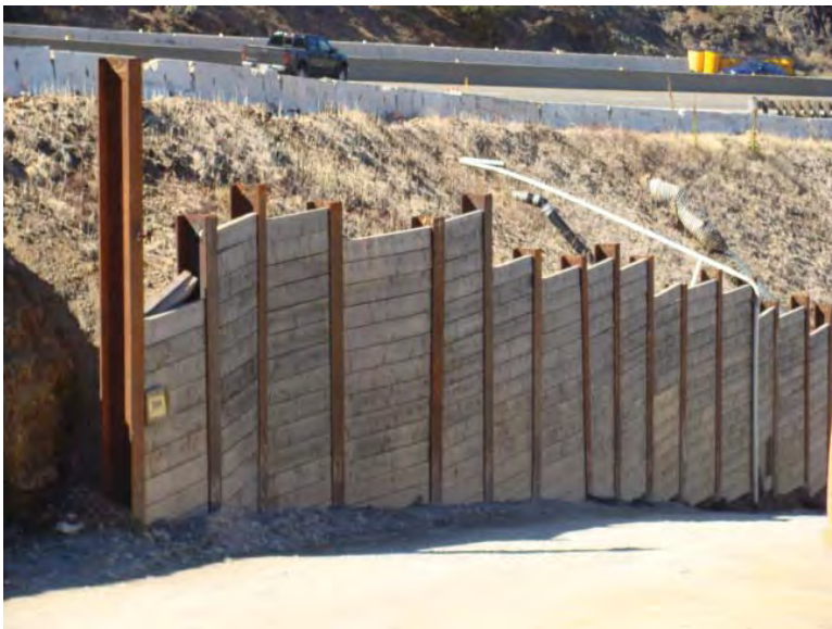
FIGURE 6.4 Cantilevered soldier beam system.
