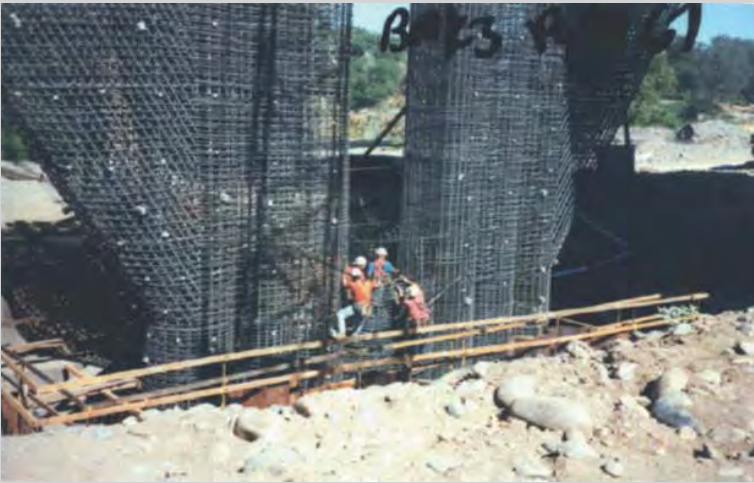
FIGURE 11.CS2 Installing braces.
