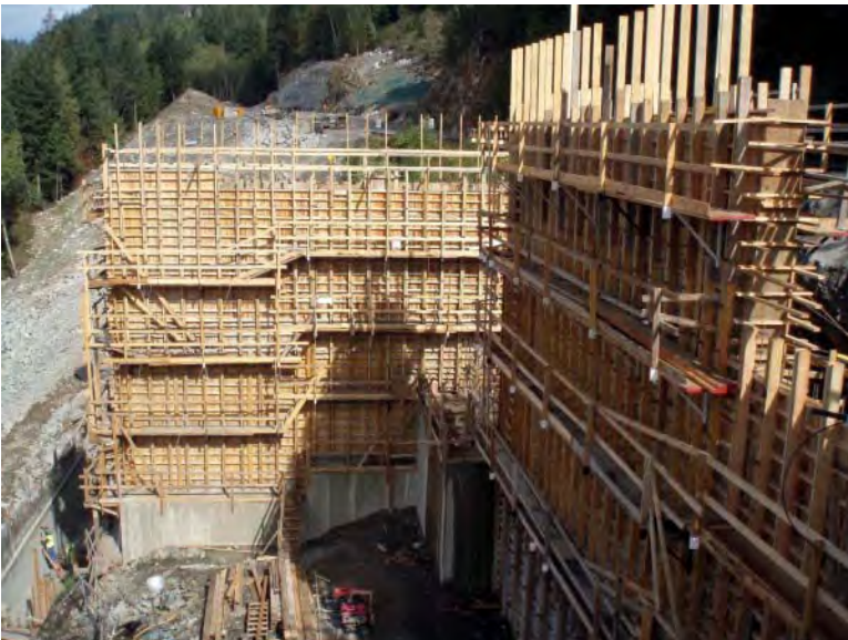
FIGURE 9.4 Typical 2 \times 4 and plywood formwork.
