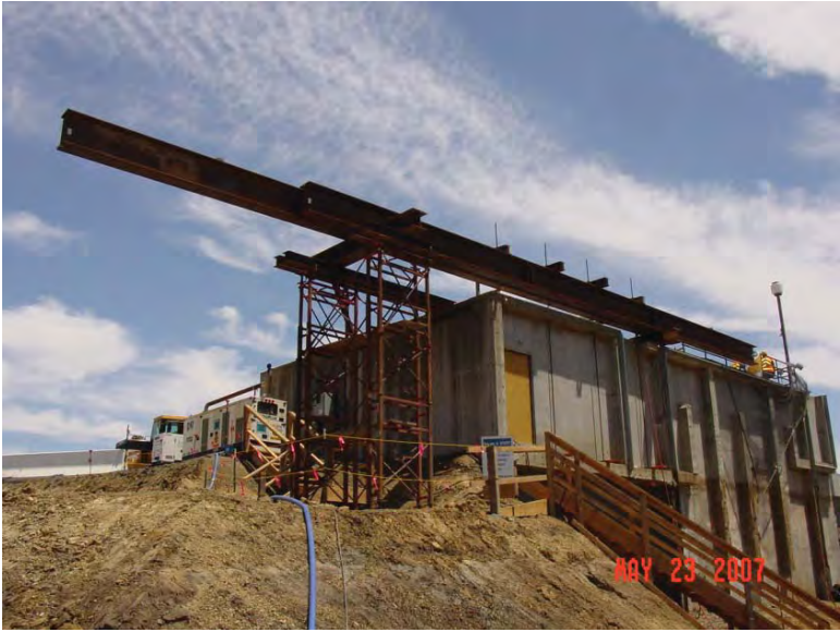
FIGURE 13.2 Temporary support of an existing structure.
