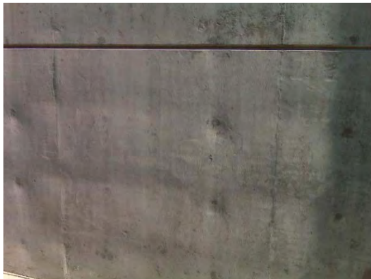
FIGURE 9.2 Plywood and stud deflection.
