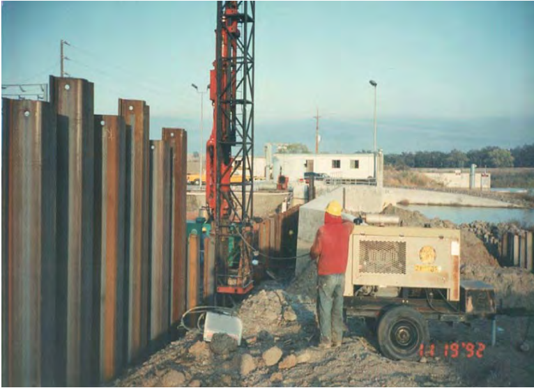
FIGURE 7.6 Sheet pile driving with an impact hammer.
