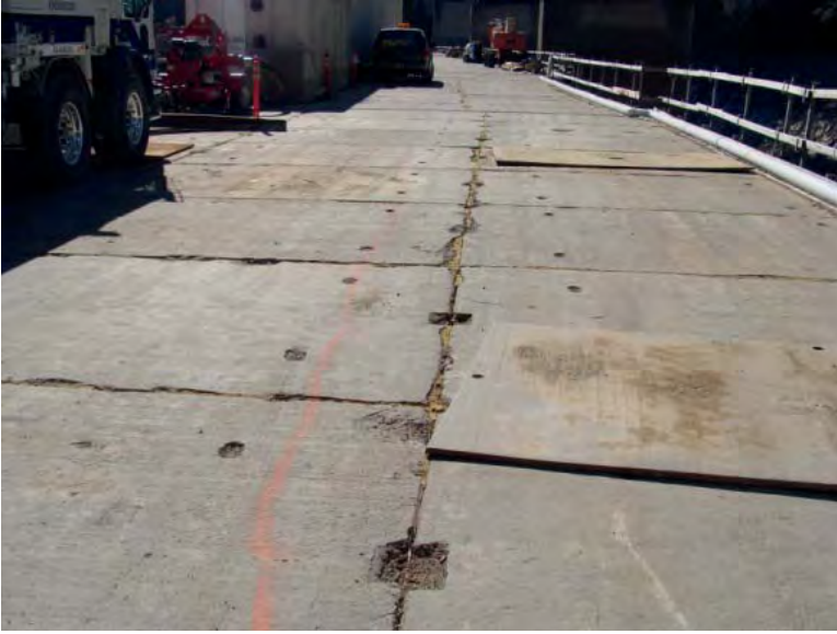
FIGURE 12.6 Precast concrete trestle deck.
