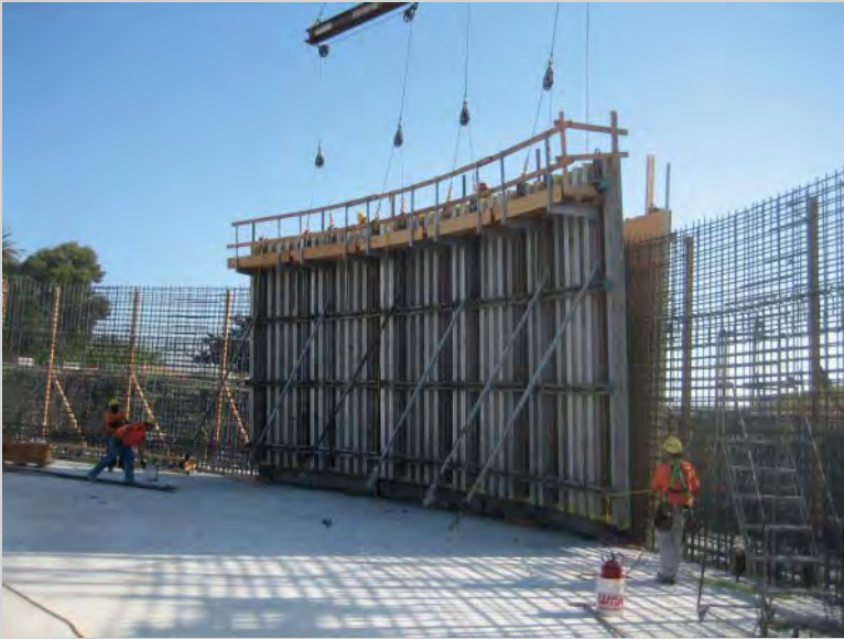
FIGURE 9.CS2 Aluminum and rolled steel channel radius forms.
