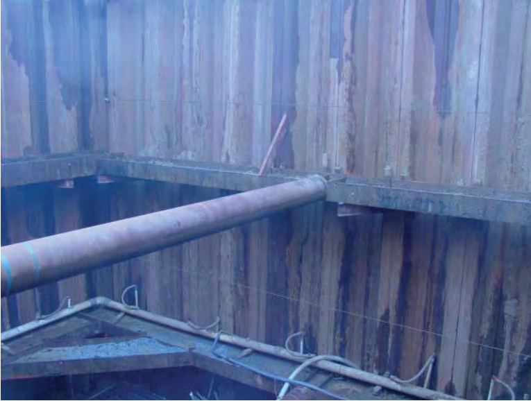
FIGURE 7.4 Sheet pile, waler, and strut system.
