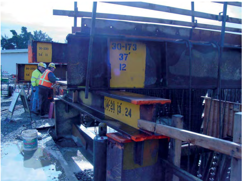
FIGURE 12.3 Stringer supported by cap beam.
