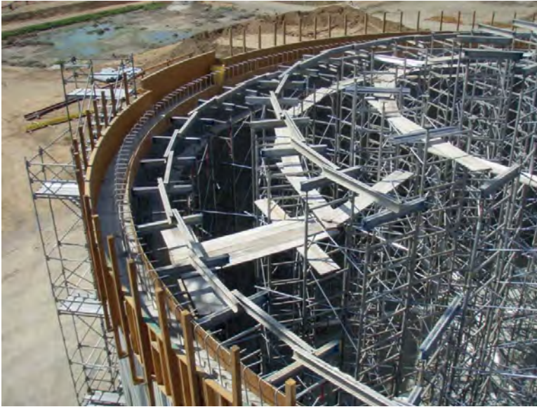
FIGURE 10.2 Water tank falsework using aluminum system.
