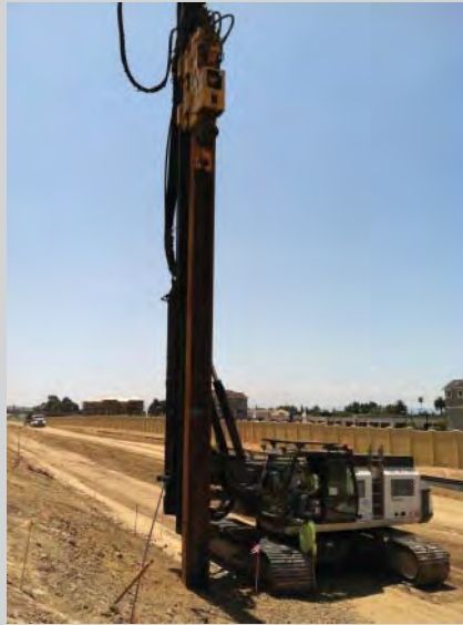
FIGURE 6.CS1 Soldier beam and plate system.
