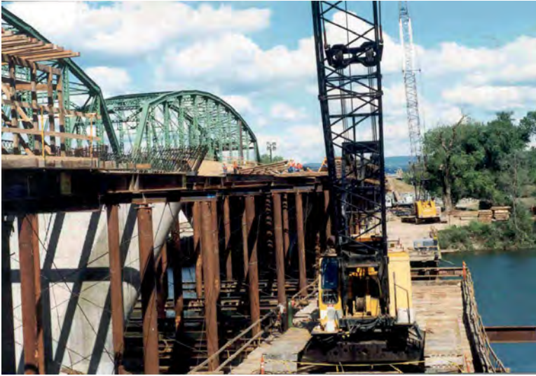
FIGURE 10.1 Pipe post falsework.
