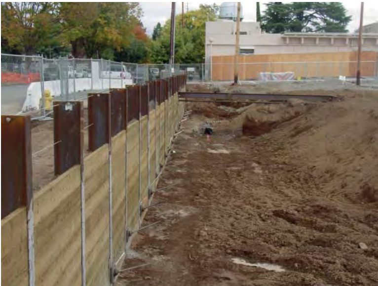
FIGURE 6.29 Soldier beam and lagging wall with tieback and no waler, Enloe Hospital, Chico, California.
