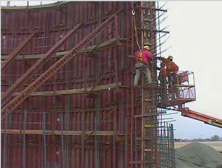
FIGURE 9.CS1 Steel forms used for a digester tank.
