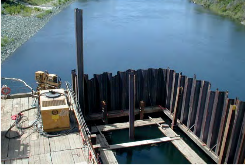
FIGURE 7.14 Internal waler in a river cofferdam.
