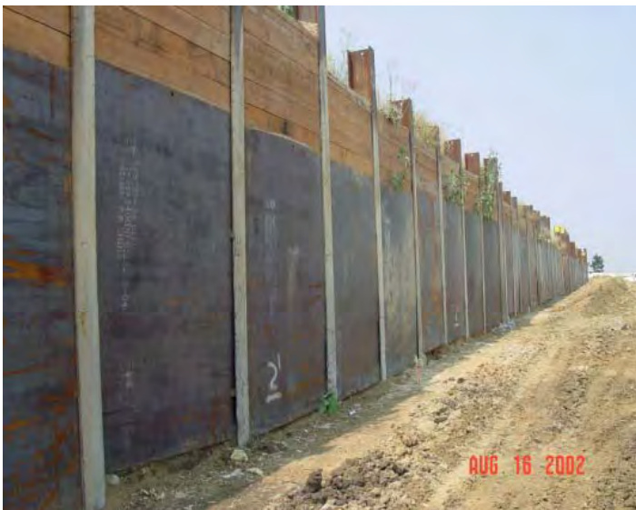
FIGURE 6.8 Combined wood and steel plate lagging.
