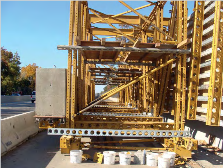
FIGURE 9.CS6 Traveling truss with counterweights.
