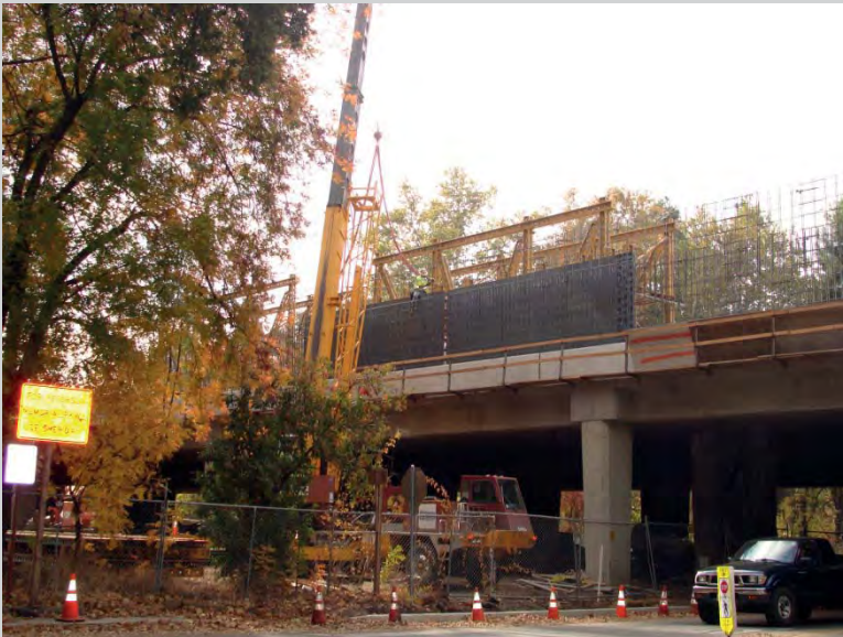
FIGURE 9.CS5B Crane hoisting first form into place.
