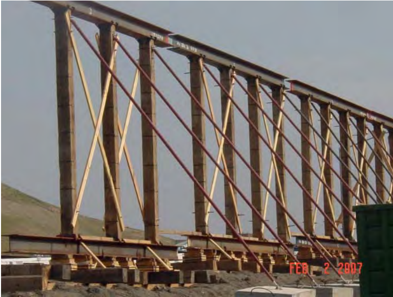
FIGURE 11.9 Falsework bent supported by pipe braces.
