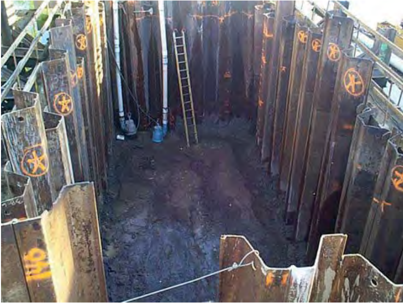
FIGURE 5.28 Sheet pile cofferdam with external walers.
