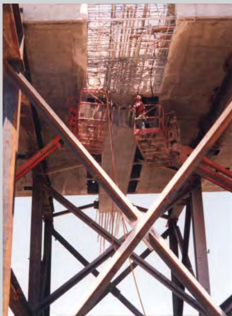
FIGURE 13.CS3 Typical bent cap replacement.
