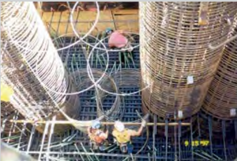
FIGURE 11.CS3 Placing of intermediate hoop reinforcing.
