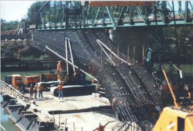
FIGURE 11.CS1 Hoisting of rebar cage.
