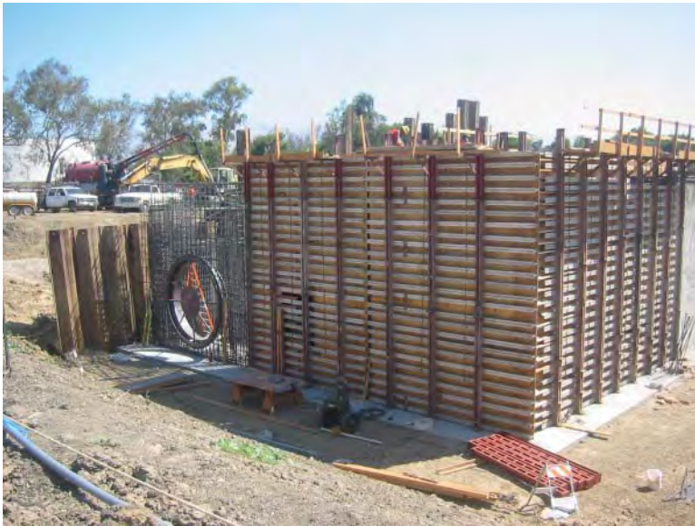
FIGURE 9.8 Composite form using alumina beams and steel channels.
