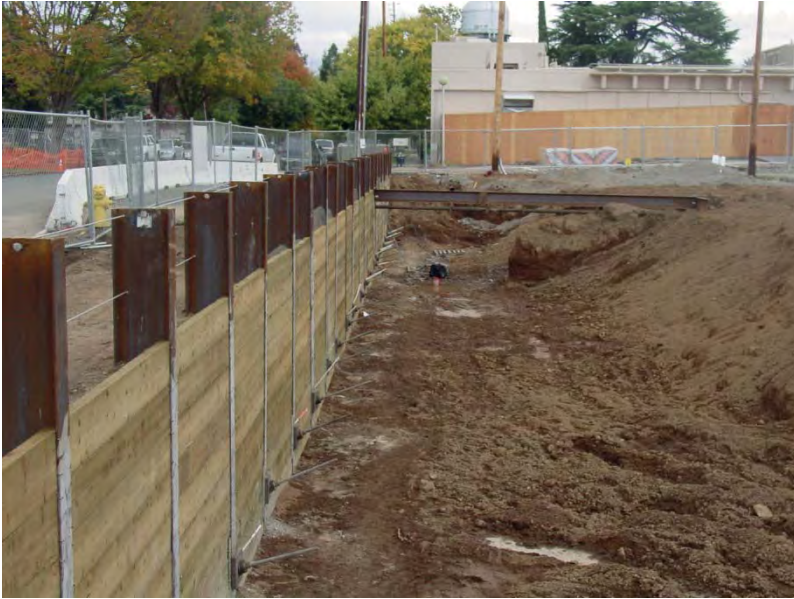
FIGURE 3.15 Soldier beam and lagging system.
