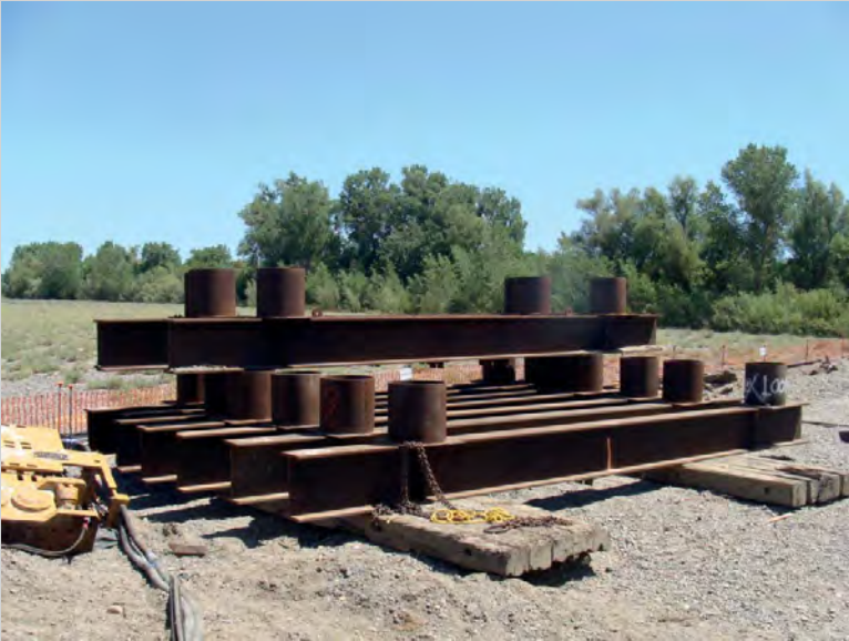
FIGURE 12.CS7 Prefabricated pile caps.
