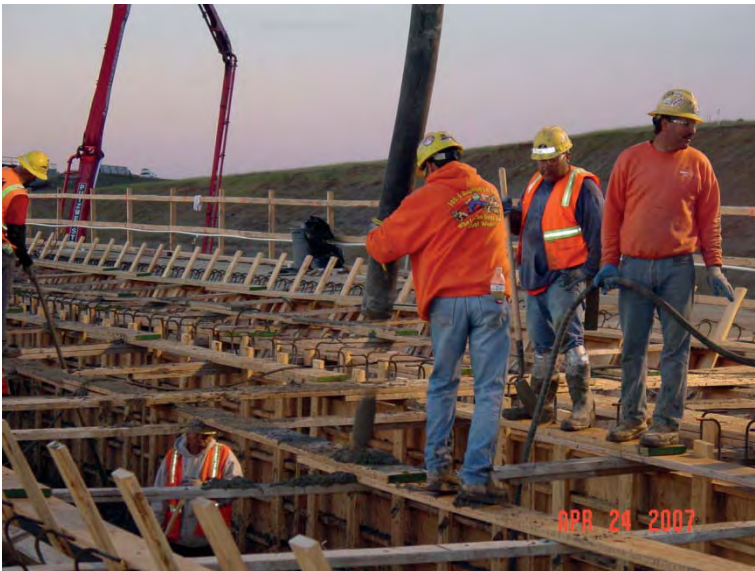
FIGURE 3.10 Concrete placement on a bridge superstructure.
