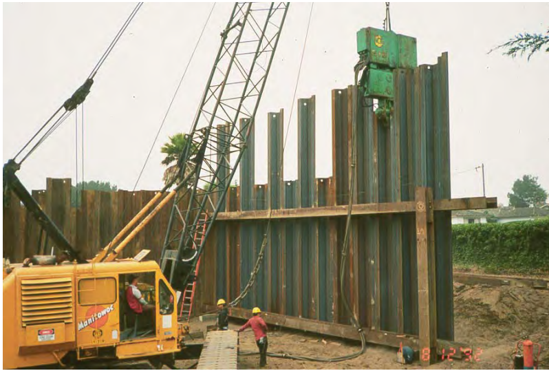
FIGURE 7.7 Two-tier driving template.
