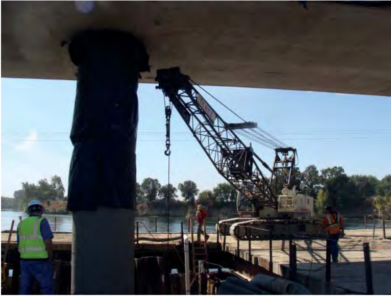
FIGURE 12.1 Driving sheet pile from work trestle.
