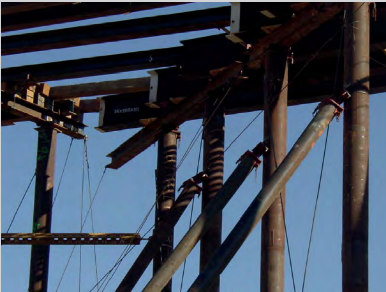
FIGURE 10.CS2 Push-pull braces added to falsework.
