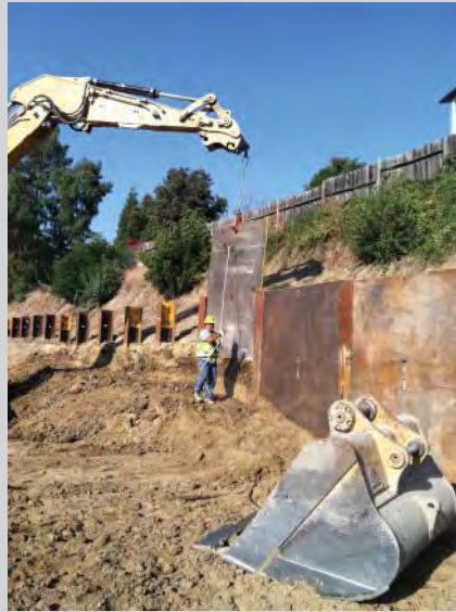
FIGURE 6.CS2 Plate installation.
