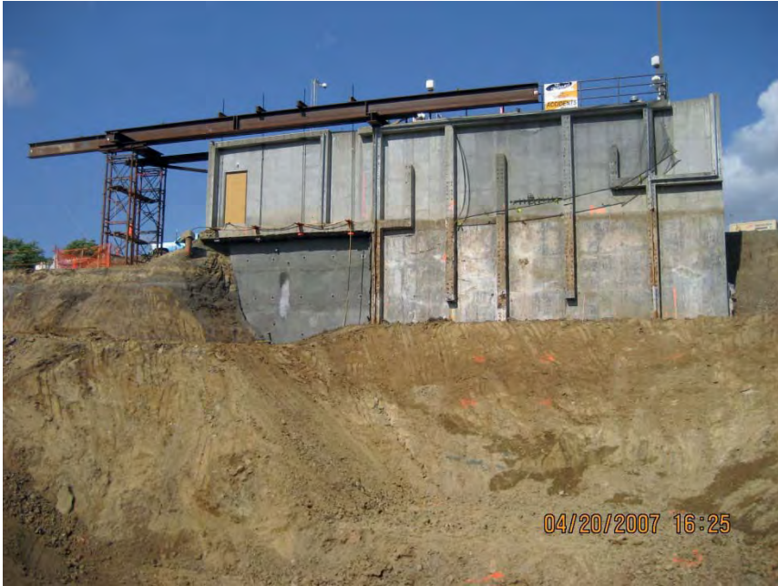
FIGURE 3.18 Temporary support of an existing structure.
