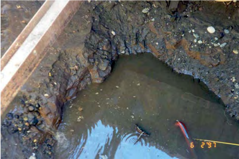
FIGURE 5.26 Soil conditions in a sheet pile cofferdam.
