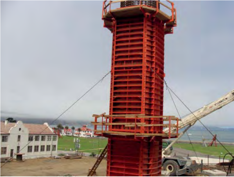
FIGURE 11.19 Pier guying system.
