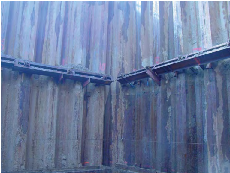
FIGURE 5.19 Double steel channel waler with tiebacks.
