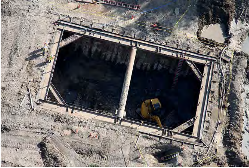
FIGURE 7.20 Aerial view of a strutted cofferdam.
