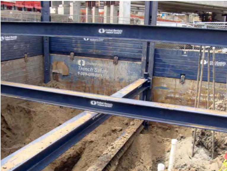
FIGURE 5.29 Slide rail system.
