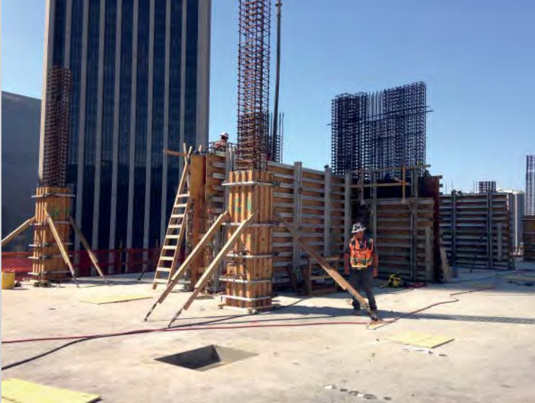
FIGURE 10.CS8 Concrete gravity columns and shear walls (courtesy of Charles Pankow, Ltd and Doka Forms).
