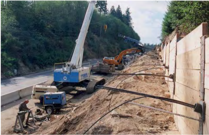
FIGURE 6.23 Soldier beam shoring with tiebacks.
