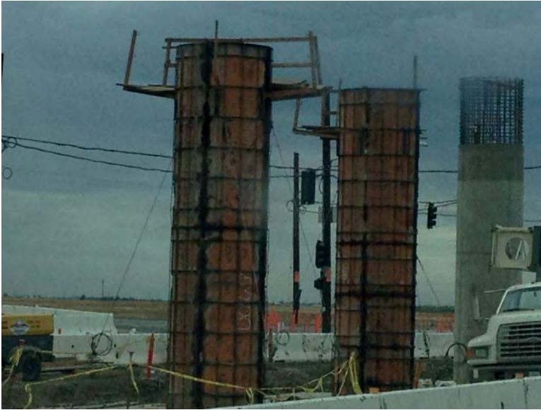
FIGURE 11.11 Pier forms guyed with wire rope.
