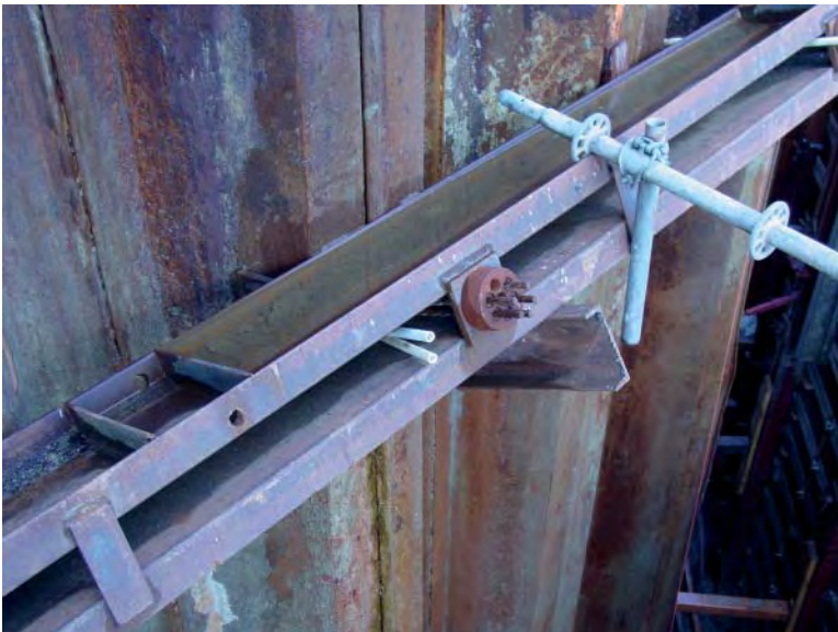
FIGURE 7.3 Double channel waler system before excavation.
