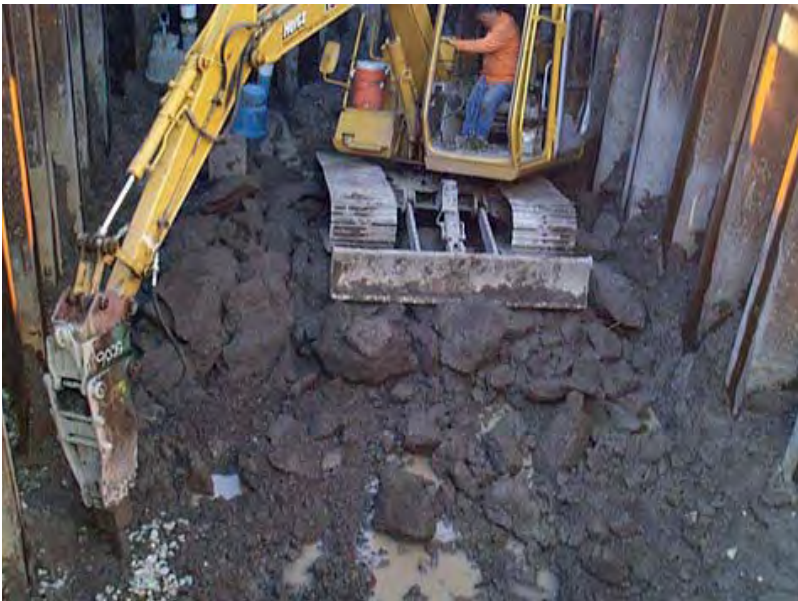
FIGURE 5.27 Methods of excavation for cemented soils.
