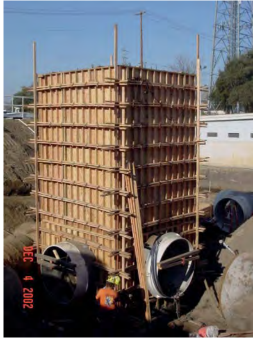
FIGURE 9.6 Junction box formed with all-wood forms.
