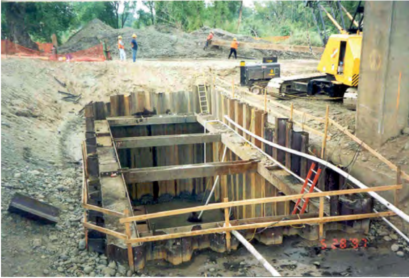
FIGURE 7.19 Struts used in a floodplain cofferdam.
