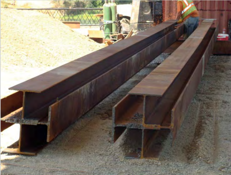
FIGURE 12.CS5 Star pile.
