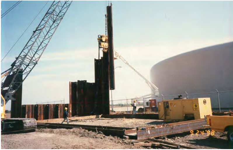
FIGURE 7.5 Pile driving operation using vibratory hammer.
