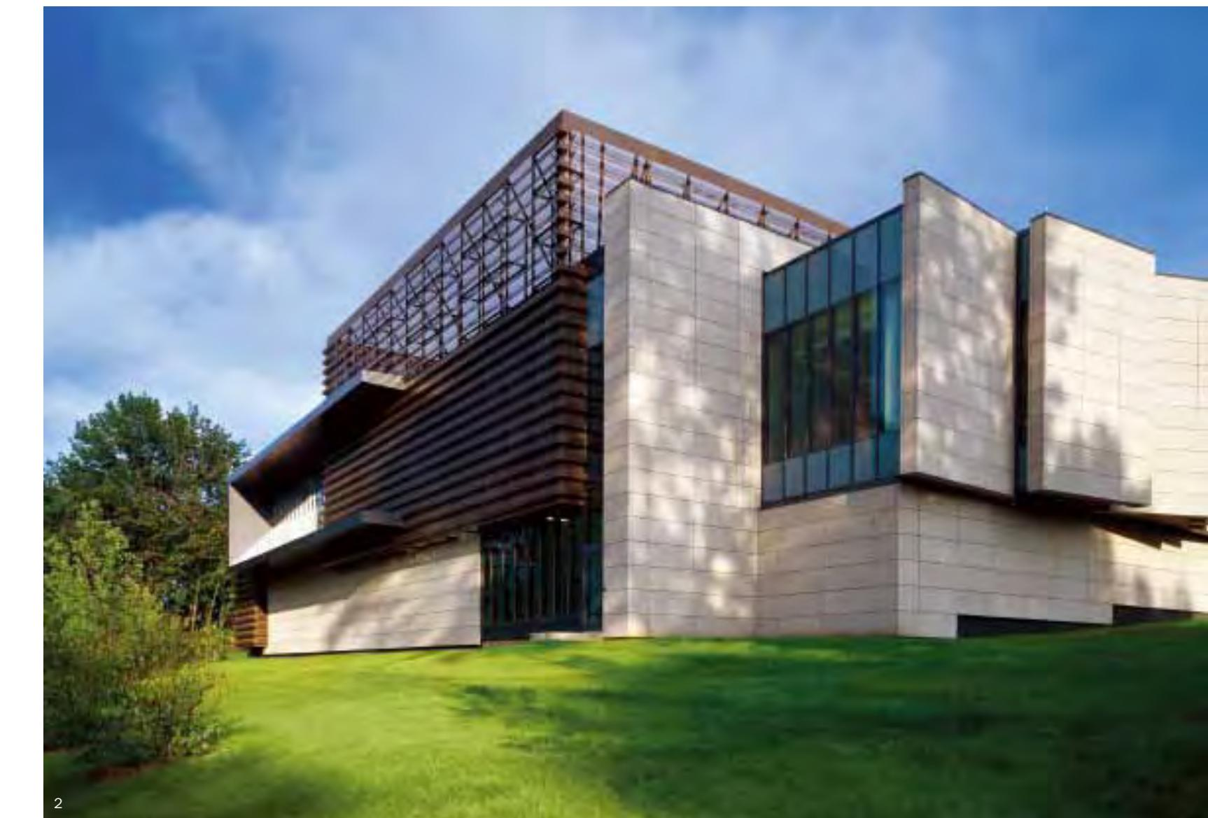
1. View of entry façade showing layering of the limestone panels
