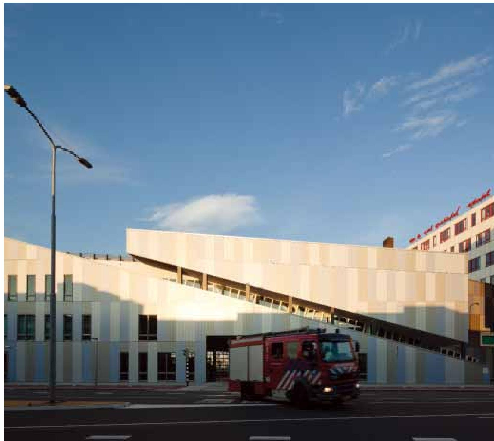
1. The visible strong slanting line on the front and back of the building forms the access ramp for the parking on the roof'
