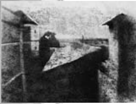
The first photograph shows a view of roofs and chimneys.
