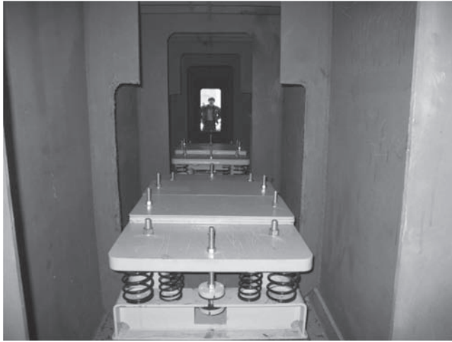
Figure 14. Vertical TMD inside steel box girder.
