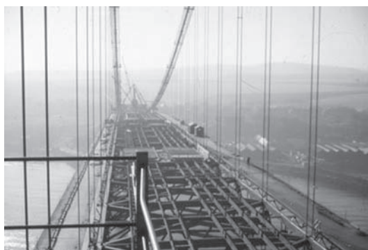
Figure 2. Deck structure showing longitudinal stringer beams during construction.
