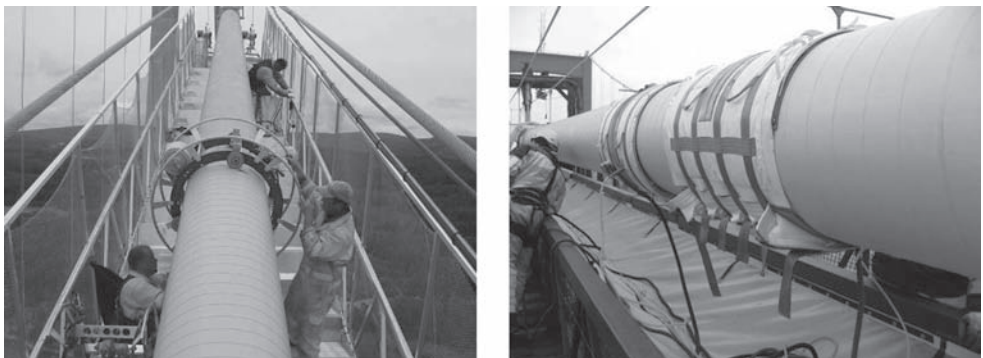
Figure 9. Wrapping with wrapping machine and bonding with heat blankets.
