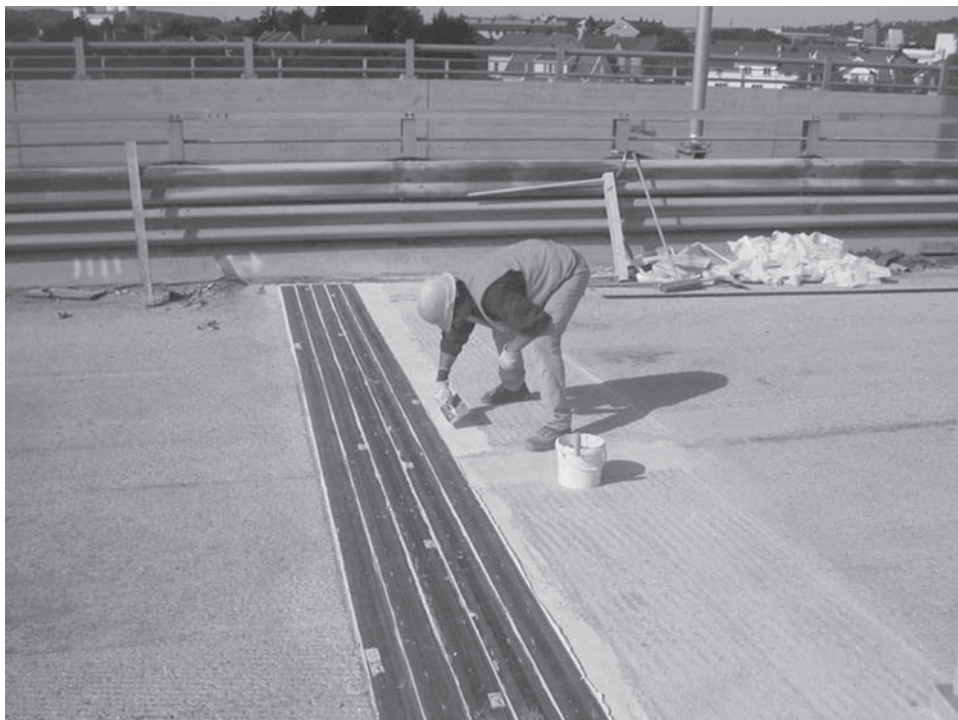
Figure 10. Carbon fiber reinforcement plates.
