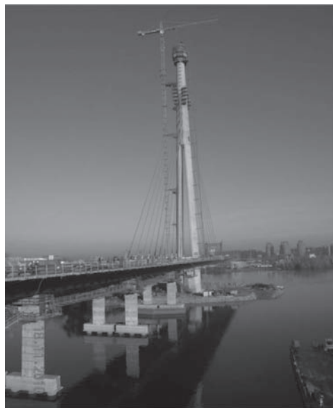
Figure 9. Tower, stage 36 of 39, elevation +161 m, November 2010.
