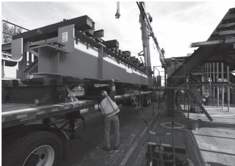
Figure 2. Prefabricated spans with ties attached.
