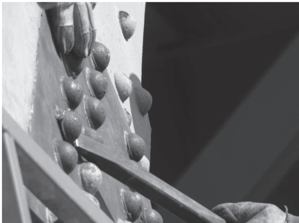
Figure 3. Mechanical rivet removal with hell dog.
