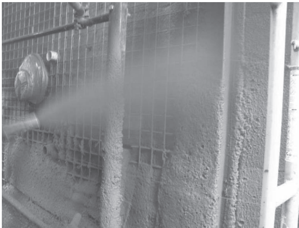
Figure 3. Shotcrete, note PVC pipe used to guide thickness.
