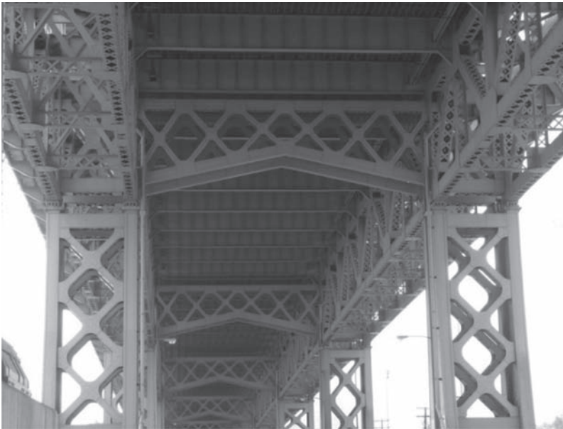
Figure 1. Deck truss spans.
