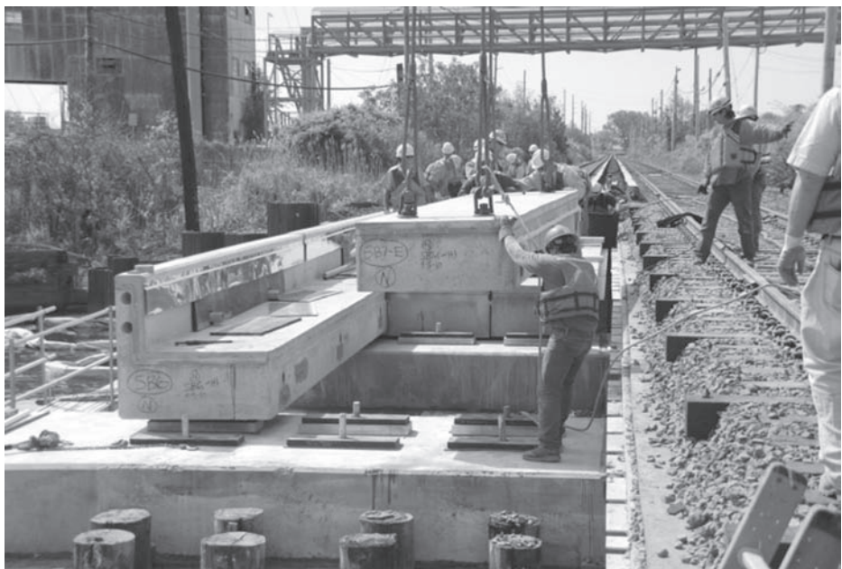
Figure 9. Installation of precast box beams.
