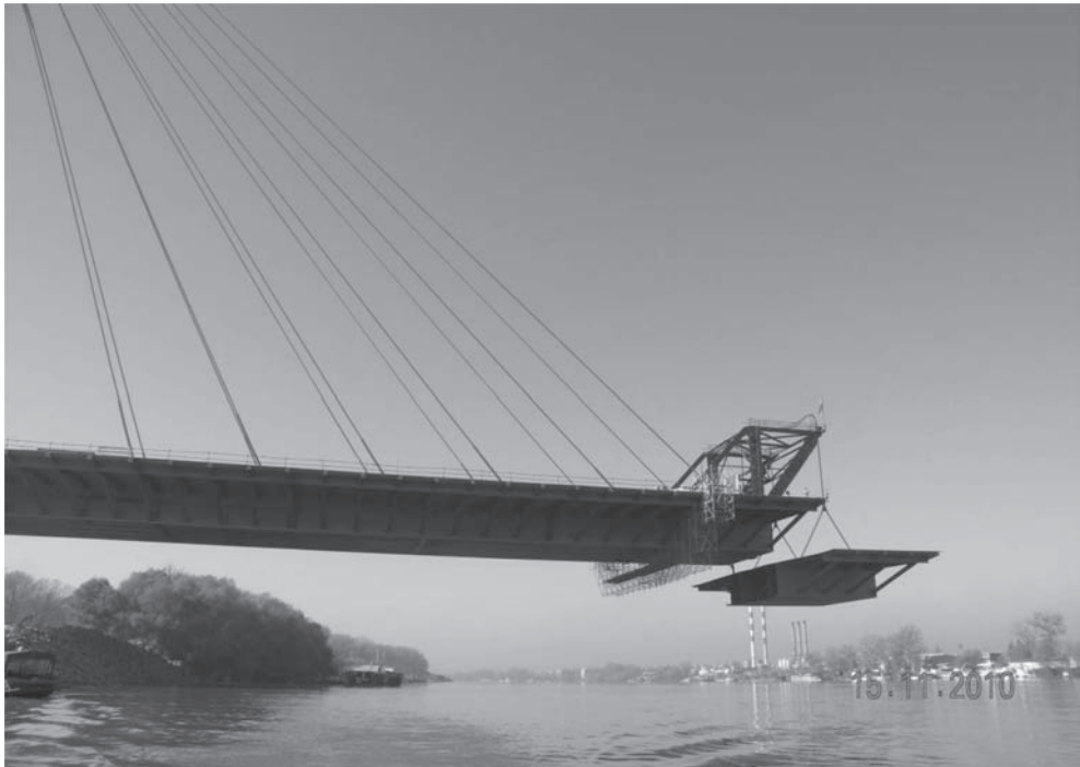
Figure 13. Free cantilevering erection, lifting of segment M7.
