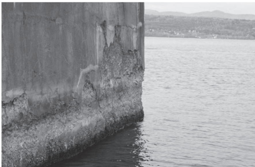
Figure 3. Pier 5 concrete deterioration in September 2009 ( Photo courtesy of NYSDOT ).
