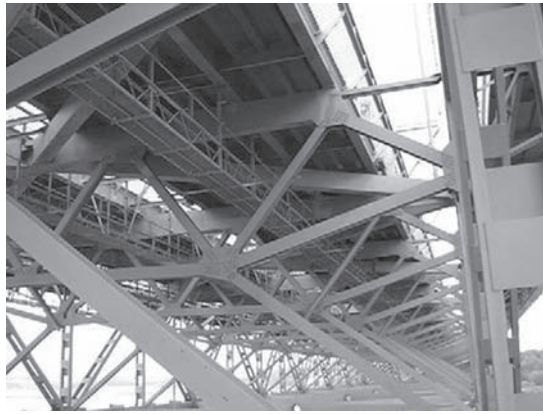
Figure 3. Deck truss showing longitudinal air gaps.
