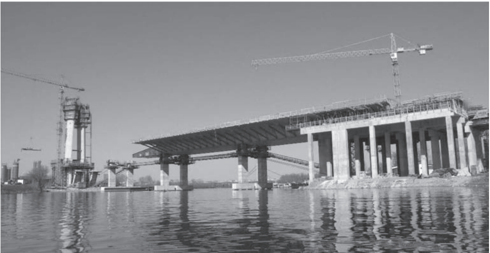
Figure 7. Incrementally launched Back Span, elevated construction yard.
