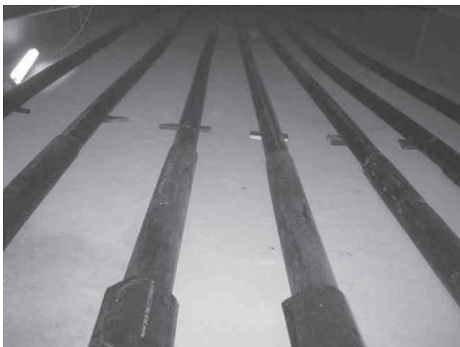
Figure 11. External cables in position.
