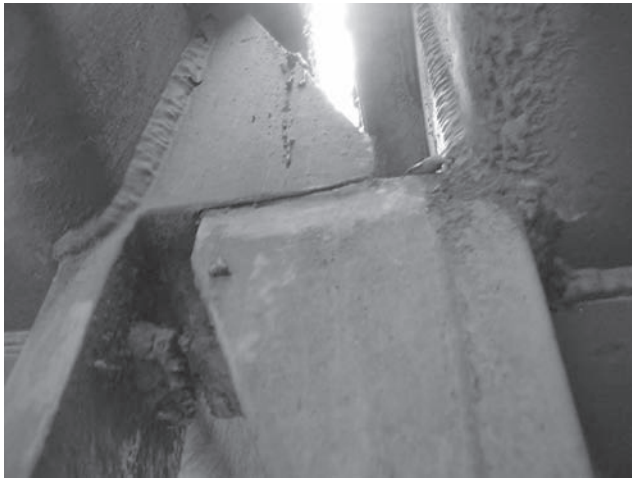
Figure 8. Existing half joint bearing block detail.
