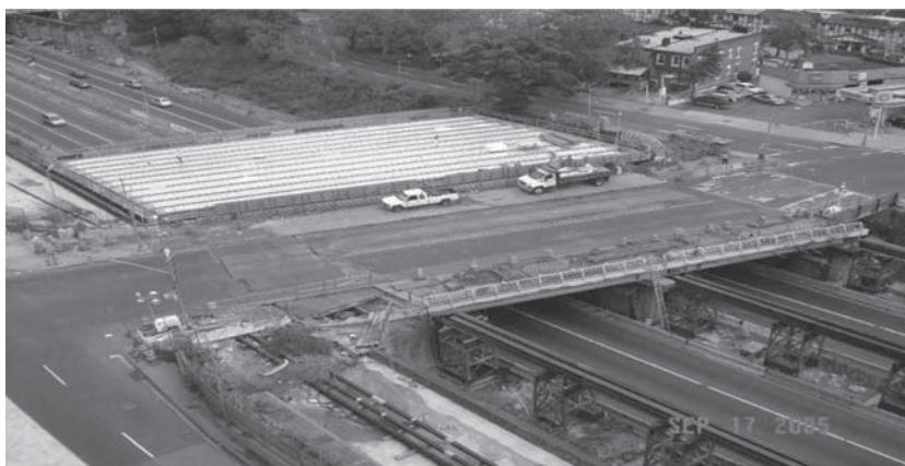
Figure 1. Tier 1 ABC Project—Jamaica Avenue over Van Wyck Expressway, New York. Weekend replacement using a lateral slide.
