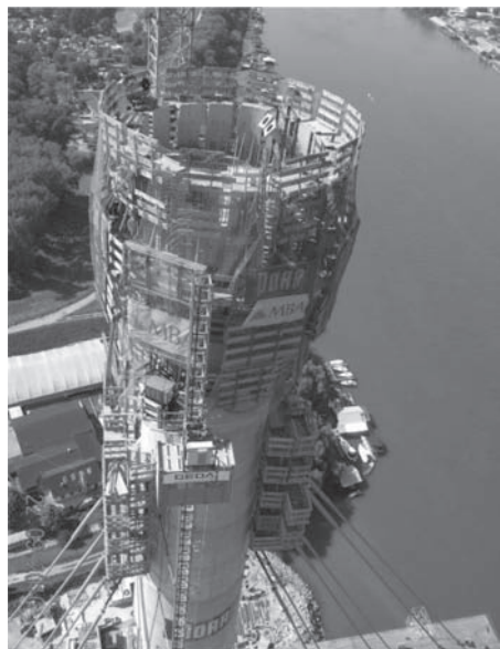
Figure 8. Climbing form of the upper cone at stay anchorage area.
