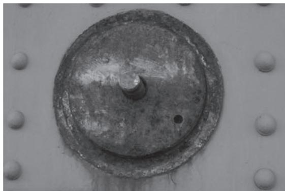
Figure 3. Truss pin inspection—surface corrosion behind pin cover.
