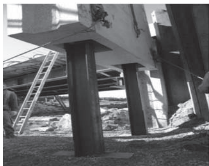
Figure 6. Precast abutment on steel H-piles.
