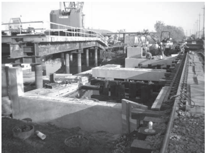
Figure 8. Precast concrete pier caps & abutments at Powell Creek Bridge.
