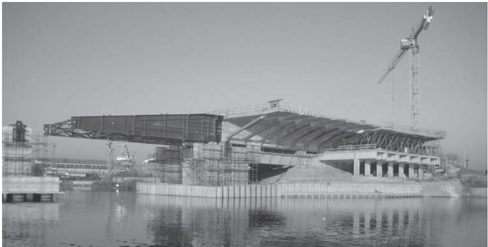
Figure 16. Launching of side span situation in November 2010.
