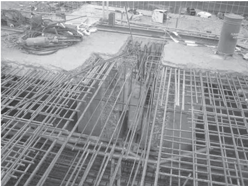
Figure 8. Chiselling in the hinge area.
