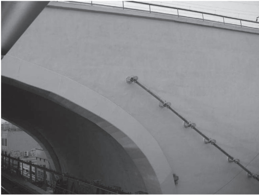
Figure 4. Finished surface, note new drain pipes with cleanout and added arch structure.
