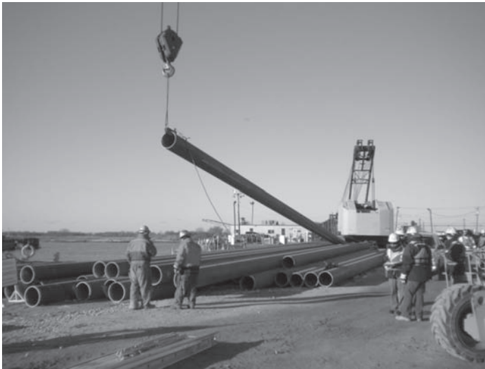
Figure 7. Steel pipe piles, 50 cm diameter.
