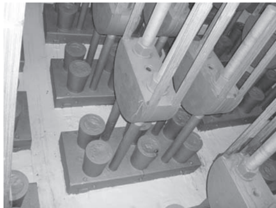
Figure 13. Anchorage strand shoe detail.
