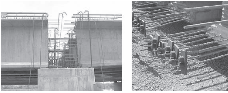
Figure 2. Precast girder connections—extended strands.
