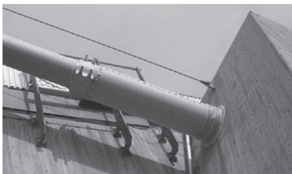
Figure 12. Shroud that is currently being replaced by a new airtight shroud.
