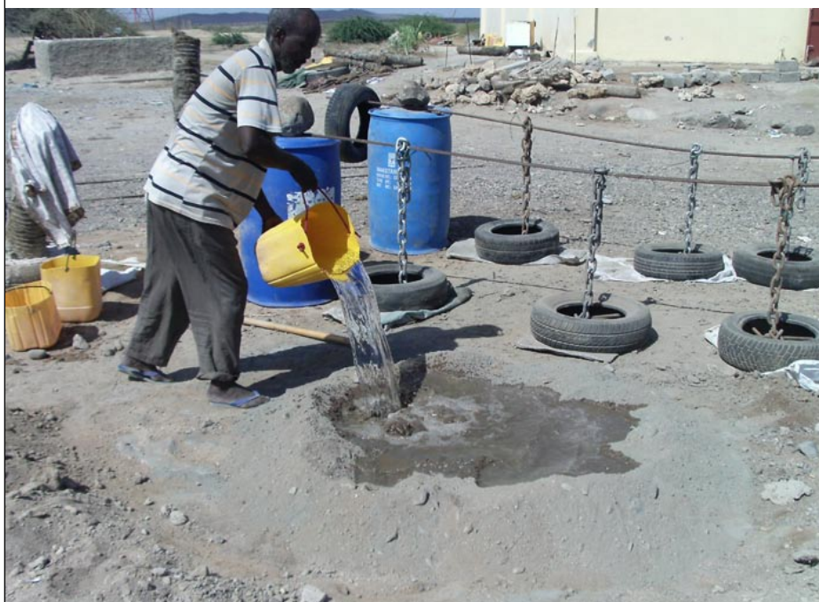
PLATE A3.1 Mixing concrete
