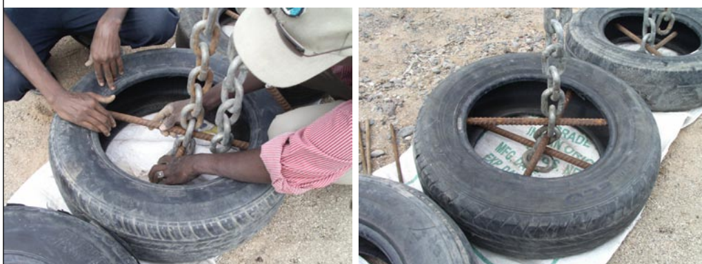
PLATE 15 Crossed iron bars in the tyres
