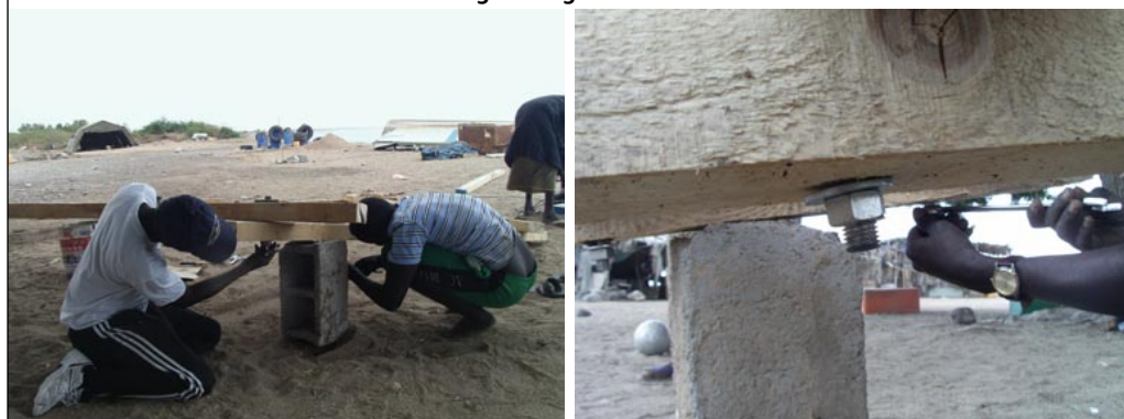
PLATE 24 Tightening of screws
