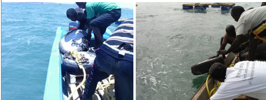
PLATE 38 Lowering the mooring posts into the sea
