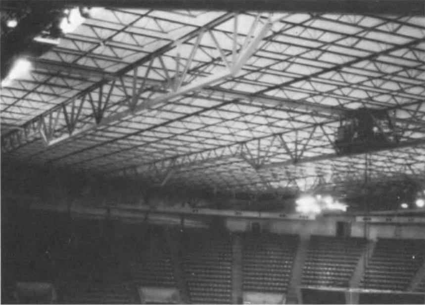
Fig. 3.10. Long-span joist roof system of the American Royal Arena in Kansas City, Missouri (courtesy of U.S. Steel Corp.).
