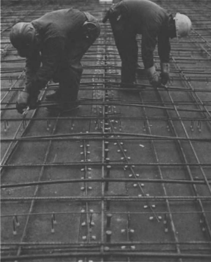
Fig. 9.2. An interior girder of the building whose spandrel beam is shown in Fig. 9.1. Note how reinforcing bars and post-tensioning strands drape over the girder toward the top of the slab to provide negative moment reinforcement.
