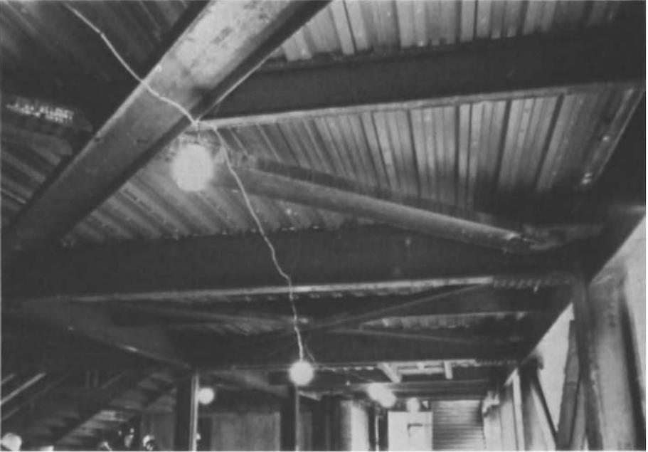
Fig. 2.3. Lateral bracing for a floor system made with channel sections.
