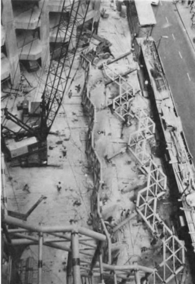
Fig. 0.3. Fabrication of special trusses at a job site to be used for the wall and roof structural system for the atrium lobby of an office building. Note that the trusses, made from tubular sections, are partially prefabricated in the shop to transportable lengths and assembled at the site to form each member.
