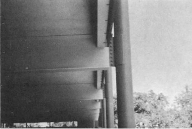
Fig. 4.1. Detail of a wide-flange beam to pipe column connection.
