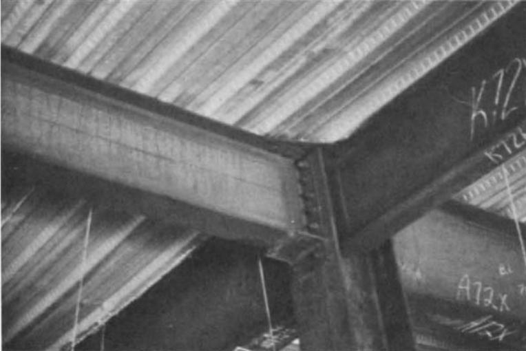
Fig. 5.3. A beam-to-column shear connection with web angles.
