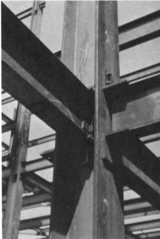
Fig. 7.4. A beam-to-column moment connection with flange angles.
