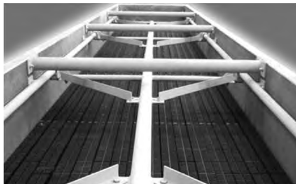
FIGURE 18.16 Rake-type sootblower for cleaning gilled tube economisers.
