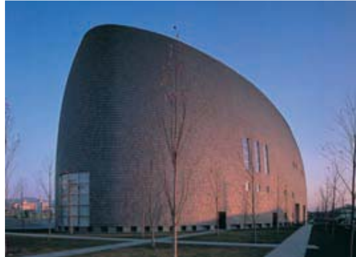
Nara Centennial Hall, Japan. Architect: Arata Isozaki
