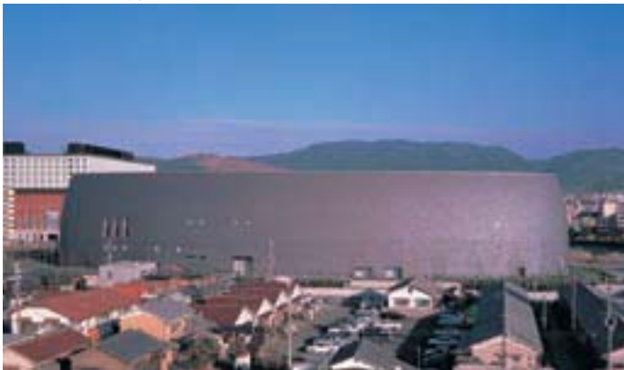
Nara Centennial Hall, Japan. Architect: Arata Isozaki
