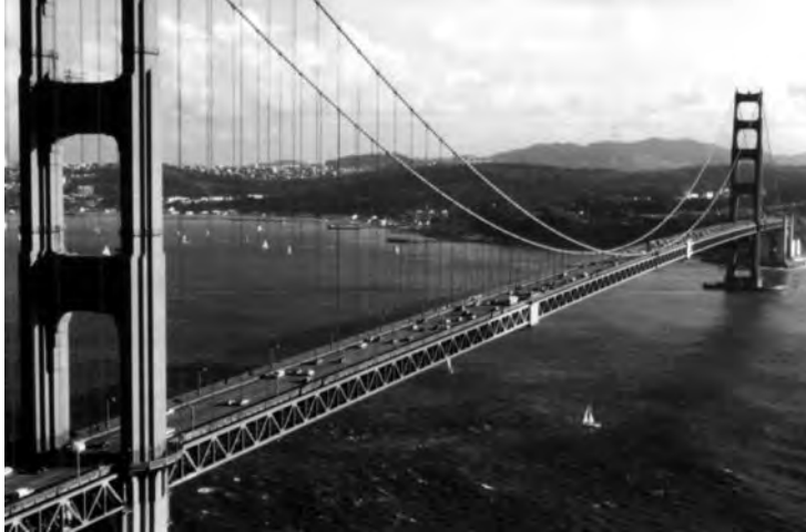
Figure 2.1.2e Golden Gate Bridge, San Francisco, California. The fundamental natural vibration periods of this suspension bridge with the main span of 4200 ft are 18.2 sec for transverse vibration, 10.9 sec for vertical vibration, 3.81 sec for longitudinal vibration, and 4.43 sec for torsional vibration. These vibration properties were determined from recorded motions of the bridge under ambient (wind, traffic, etc.) conditions. (Courtesy of International Structural Slides.)
