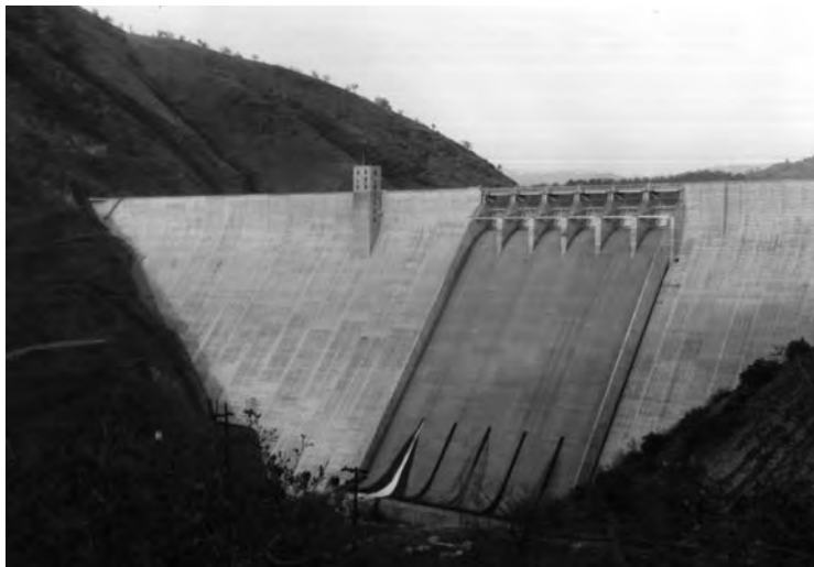
Figure 2.1.2d Pine Flat Dam on the Kings River, near Fresno, California. The fundamental natural vibration period of this 400-ft-high concrete gravity dam was measured by forced vibration tests to be 0.288 sec and 0.306 sec with the reservoir depth at 310 ft and 345 ft, respectively.
