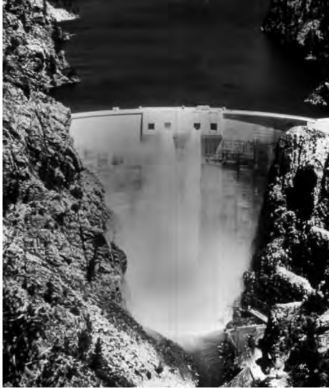
Figure 1.10.2 Morrow Point Dam, a 465-ft-high arch dam, on the Gunnison River, Colorado. Determined by forced vibrations tests, the fundamental natural vibration period of the dam in antisymmetric vibration is 0.268 sec with the reservoir partially full and 0.303 sec with a full reservoir. (Courtesy of U.S Bureau of Reclamation.)
