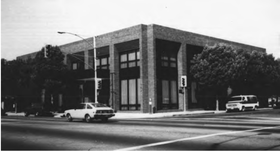
Figure 13.4.1 First Federal Savings building, a two-story reinforced-concrete building (with a partial basement) in Pomona, California. (Courtesy of California Strong Motion Instrumentation Program.)
