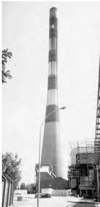
Figure 2.1.2f Reinforced-concrete chimney, located in Aramon, France. The fundamental natural vibration period of this 250-m-high chimney is 3.57 sec; it was determined from records of wind-induced vibration.
