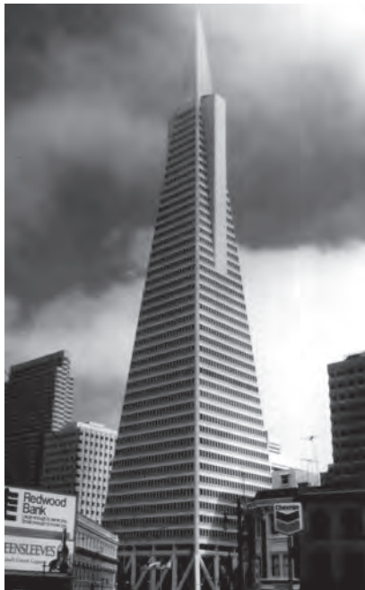
Figure 2.1.2b Transamerica Building, San Francisco, California. The fundamental natural vibration periods of this 49-story steel building, tapered in elevation, are 2.90 sec for north–south vibration and also for east–west vibration. These vibration properties were determined by forced vibration tests. (Courtesy of International Structural Slides.)
