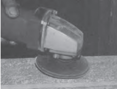
Grinding the Concrete Surface
