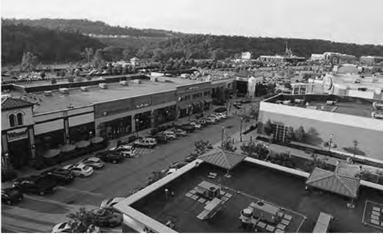
FIGURE 3.18 The Waterfront, the sprawling entertainment, retail, and residential complex in Homestead, Pennsylvania, was once a brownfield. (Photo by Matt Freed of the Post-Gazette .)
