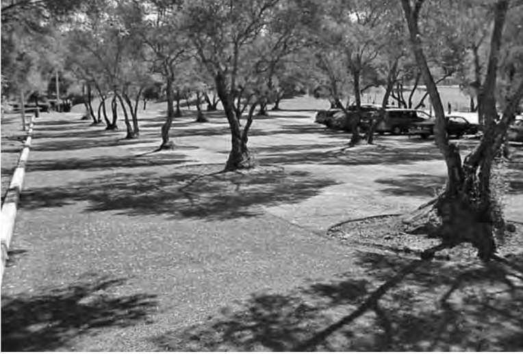
FIGURE 7.8 Pervious concrete in Miller Park, Fair Oaks, California, saved 23 mature olive trees. This parking area is designed to retain aesthetics while providing function and ADA compliance. (From Youngs, A. California–Nevada Cement Association presentation, available at www.concreteresources.net ; click “Pervious Concrete.”)
