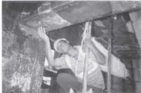
Repair of Hairline Cracks
