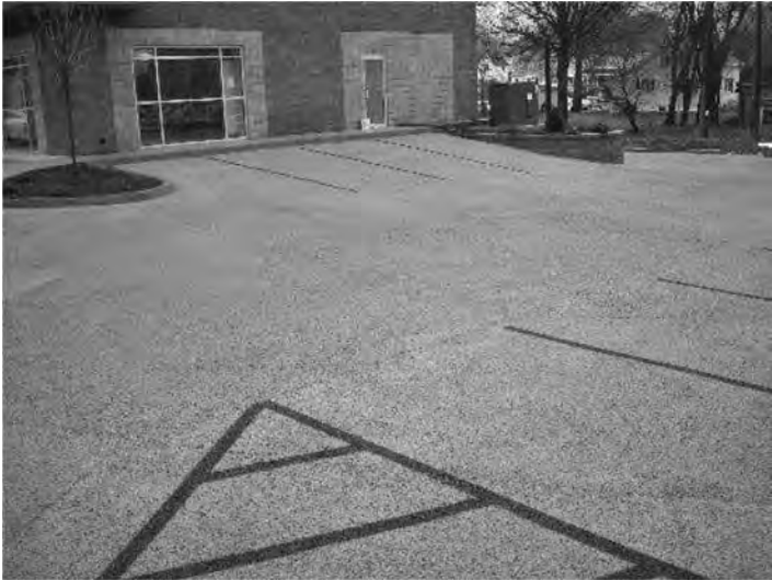
FIGURE 7.6 Parking lot with pervious concrete.
