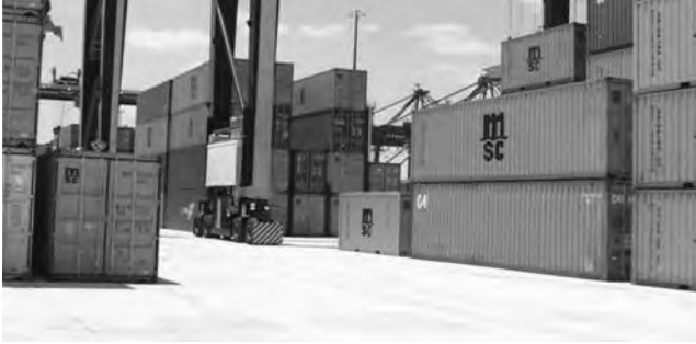
FIGURE 6.13 Port facility in Houston, Texas. (From Harrington, D. et al. 2010. Guide for roller compacted concrete pavements. Ames, IA: CP Tech Center and PCA.)
