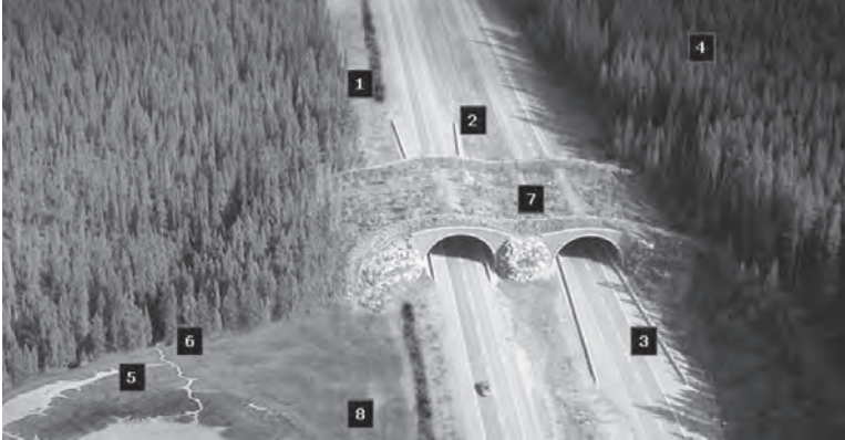
FIGURE 3.19 Technologies involved in green highways. (From http://www.greenhighways.org ; accessed July 10, 2009. Photo: Tony Clevenger.)
