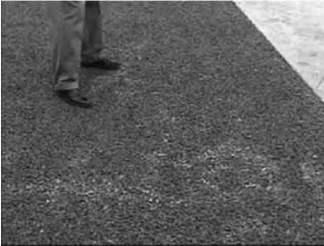
FIGURE 7.1 Demonstration of water draining in pervious concrete. (Courtesy of Green Builder.)
