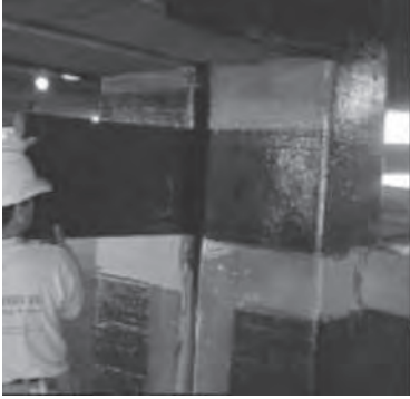
Wrapping with Carbon Fiber
