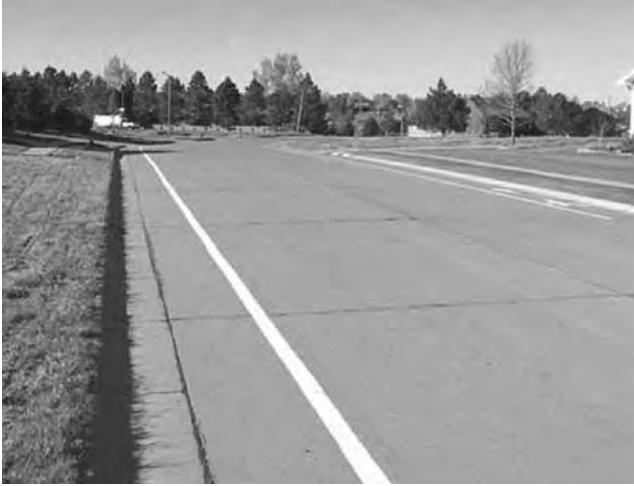
FIGURE 6.15 RCC pavement/street used as a local road. (From Harrington, D. et al. 2010. Guide for roller compacted concrete pavements. Ames, IA: CP Tech Center and PCA.)
