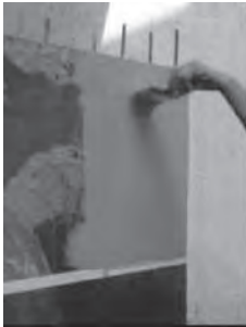
Application of Saturant
