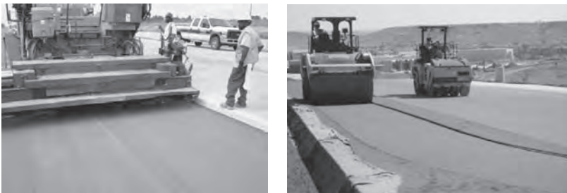
FIGURE 6.9 RCC laying and compaction. (Courtesy of John Edwards.)
