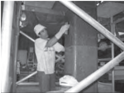
Application of Saturant on FRP Wrapping
