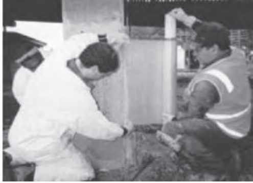
Wrapping with Glass Fiber
