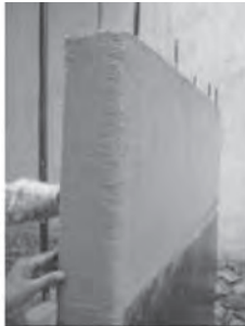
Application of Saturant
