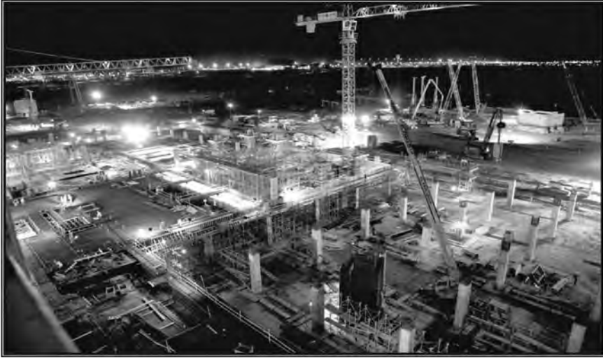
FIGURE 9.5 Masdar Institute under construction.
