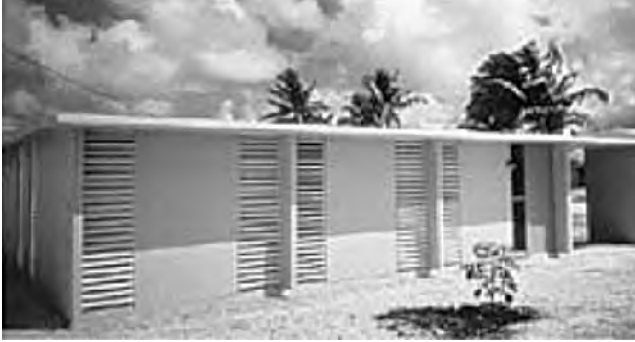
FIGURE 4.1 A typical house design that was constructed in Guam. Nearly 40 years after their initial construction, the homes have demonstrated an excellent record of disaster performance and over 6,000 such homes have been constructed. (From Warnes, C. E. 2008. Disaster-resistant shell houses. Concrete International , May 2008.)
