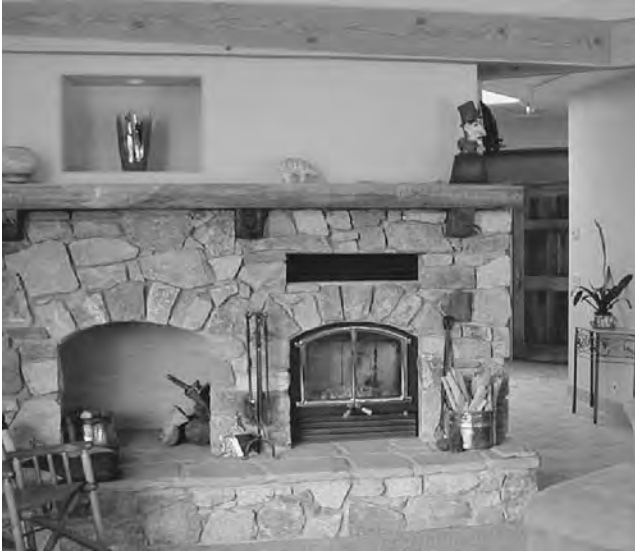
FIGURE 4.7 Efficient fireplace system that successfully heats a 4600-ft 2 ICF home in winter. (Author's photo.)
