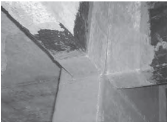
RC Columns after Completion of FRP Wrapping
