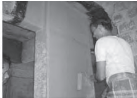
Application of Saturant on FRP Wrapping
