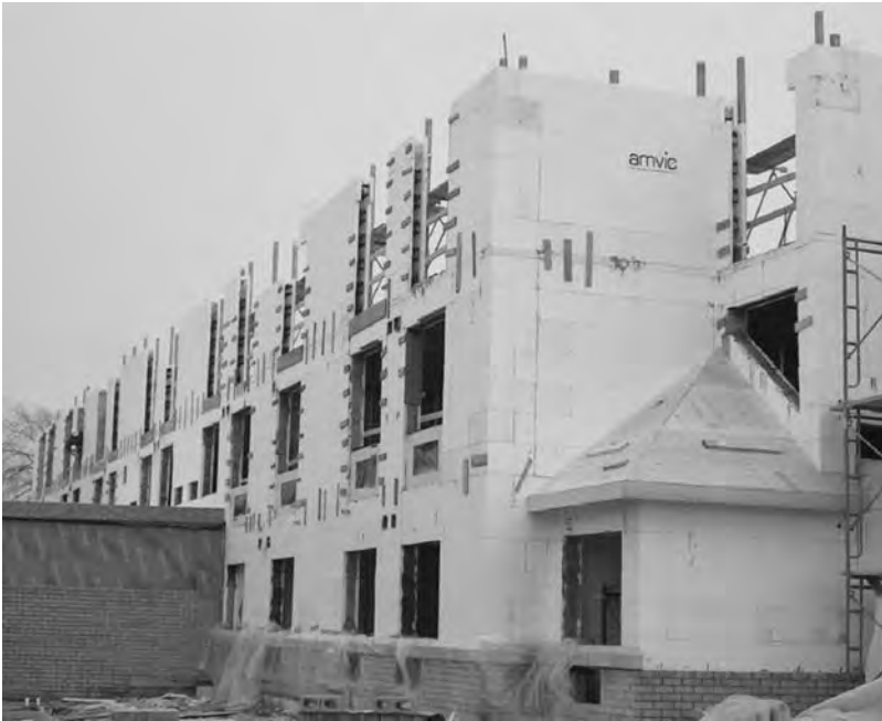
FIGURE 4.12 Best Western during construction. (Courtesy of Amvic Building Systems.)
