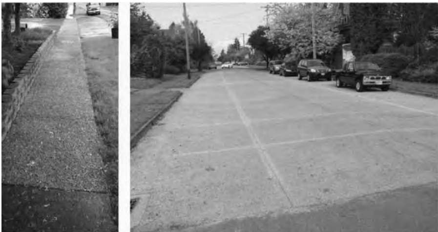
FIGURE 7.5 Sidewalk and low-volume pavements.
