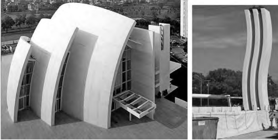
FIGURE 3.13 Jubilee Church in Rome and the gateway sculptures at the new I-35W bridge at Minneapolis, where self-cleaning photocatalytic concrete has been used. (From http://www.concretedecor.net ; http://projects.dot.state.mn.us/35wbridge .)
