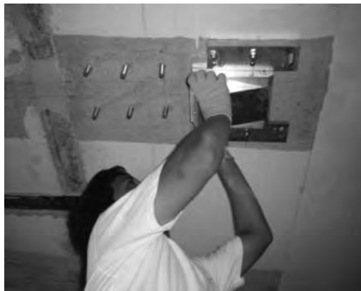
FIGURE 10.7 Positioning of laminate clamping device between L-clamps.
