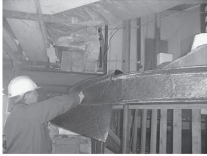
**13.8** Boots Store Nottingham, upgrading a curved-in-plan steel beam with high modulus, site cured pre-impregnated CFRP composite (by kind permission of Taylor Woodrow Technical Centre, UK and ACG Derbyshire UK, and Elsevier for Fig. 13.7a from Hollaway and Head, 2001).
