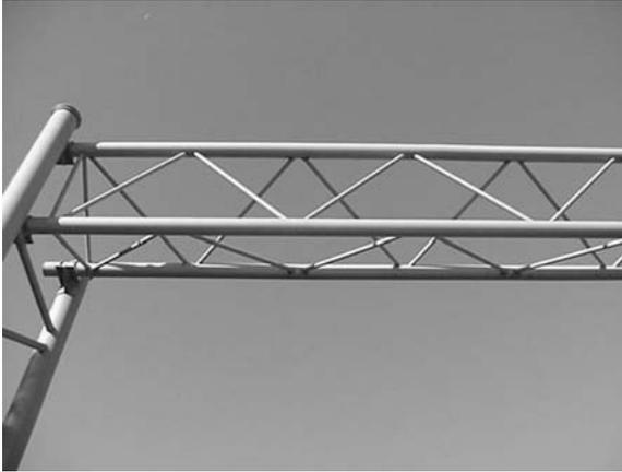
13.7 Tri-truss aluminium overhead sign support structure (by kind permission of Professor C Pantelides, University of Utah, USA).
