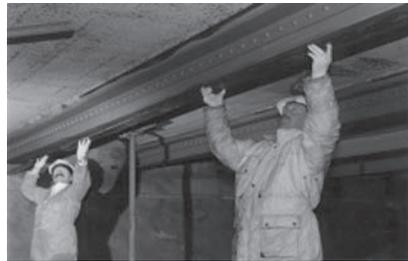
**13.9** Strengthening Slattocks Steel Bridge with unstressed pultruded CFRP plates. Location: Rochdale, UK (by kind permission of Mouchel Parkman, West Byfleet, UK).
