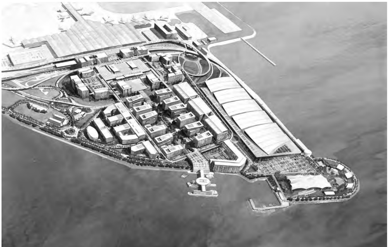
▲ 6.56 SkyCity (and ferry jetty) (Source: website www.hongkongairport.com ).
