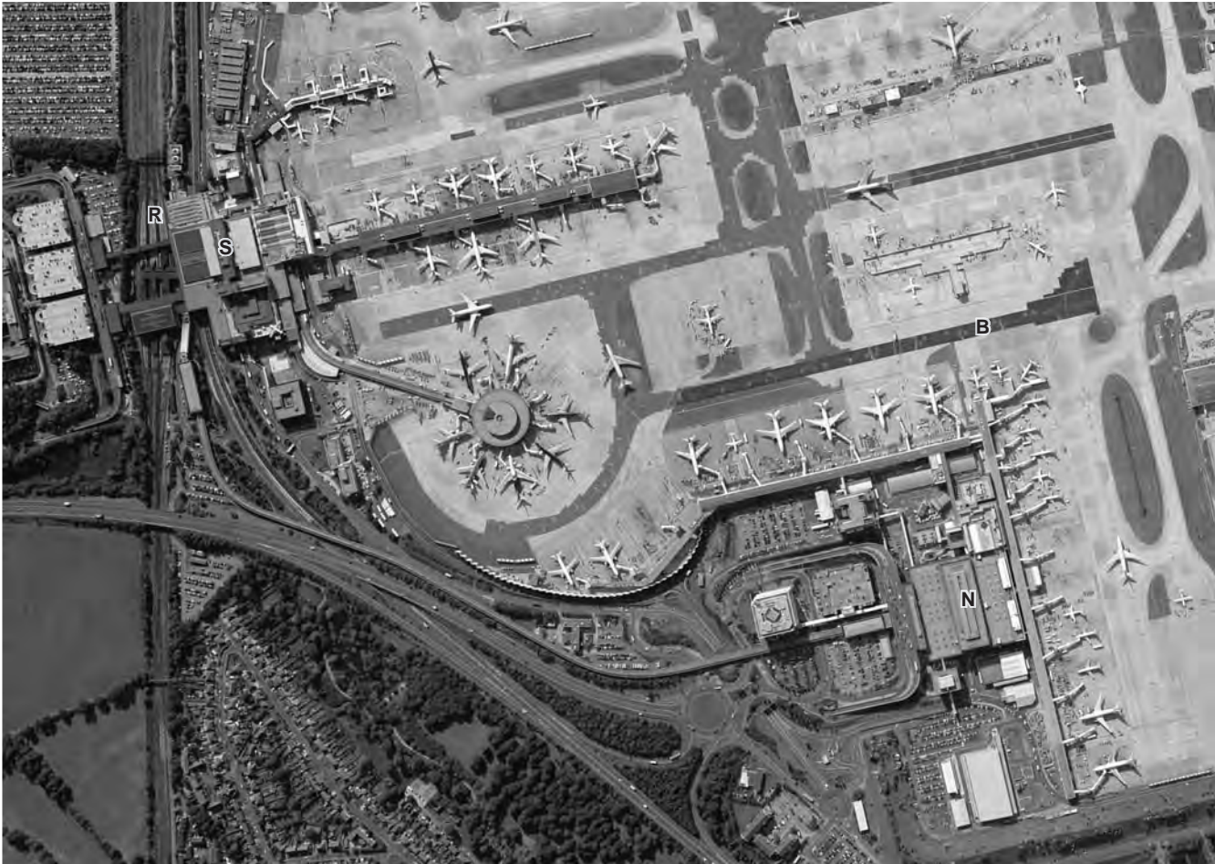
▲ 6.51 Gatwick Airport: aerial photo (courtesy of www.baa.com/photolibrary).
