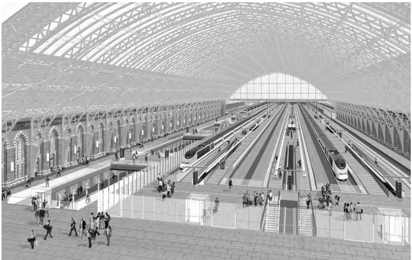
▲ 6.144 Interior view inside train-shed (Courtesy of CTRL Press Office).
