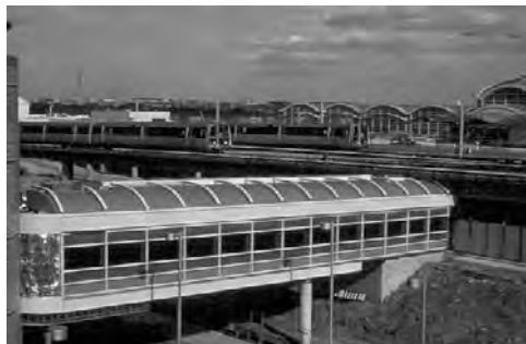
▲ 6.100 (a, b) Metro at airport terminal (Courtesy of Metropolitan Washington Airport Authority).
