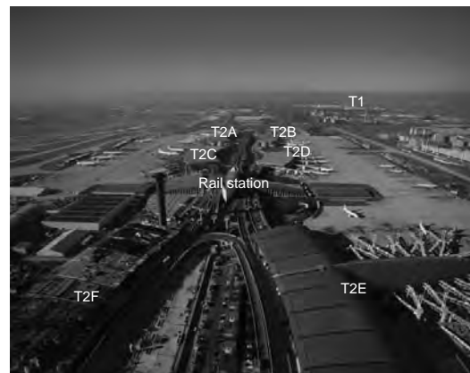
▲ 6.33 Paris Charles de Gaulle Airport, aerial view, 2003 (Courtesy of Aeroports de Paris).
