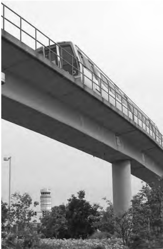
▲ 6.101 Metro leaving airport (Courtesy of Metropolitan Washington Airport Authority).
