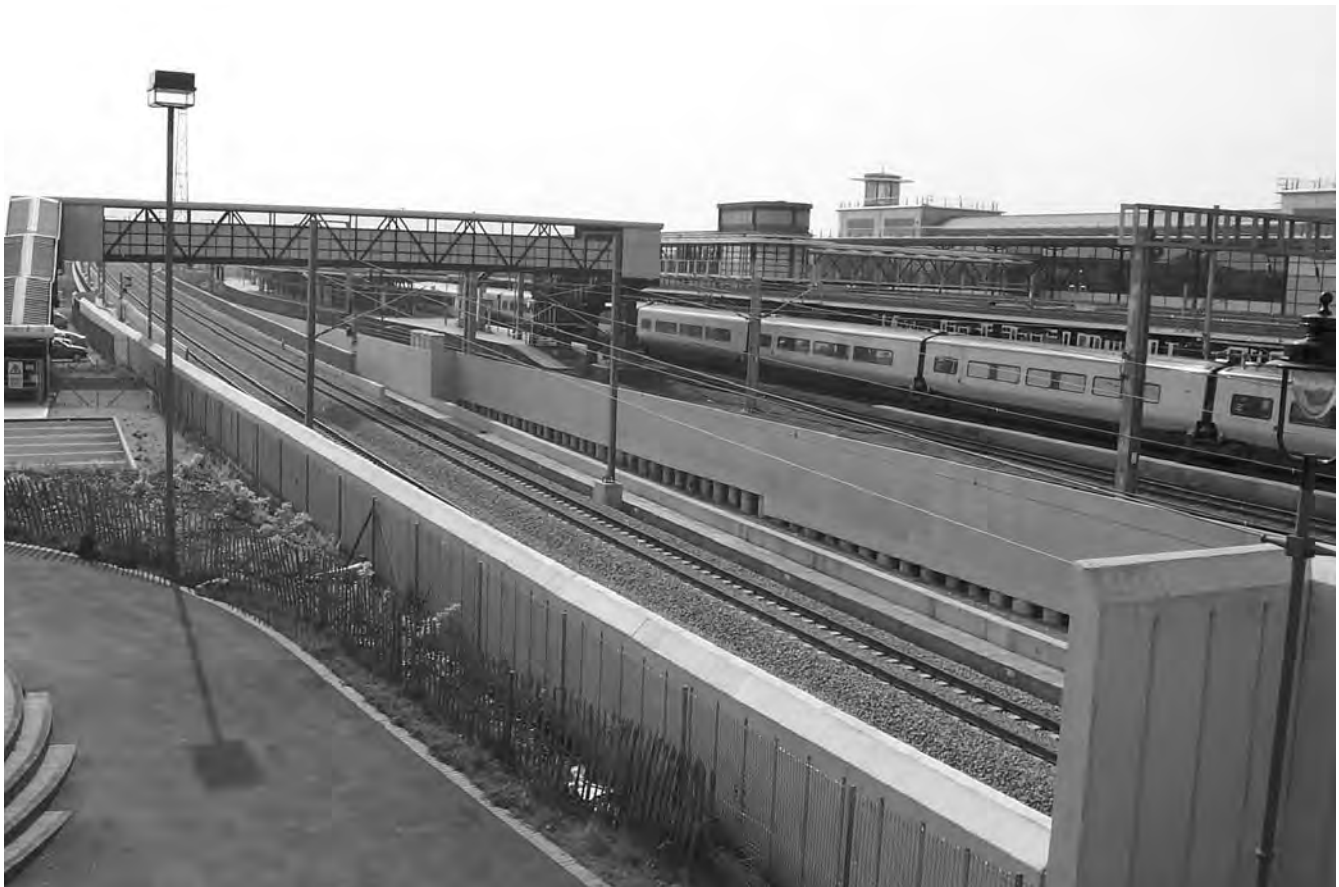
▲ 6.126 Railway-side photo showing bypass for non-stop trains, domestic platform, international station and terminal building in background.
