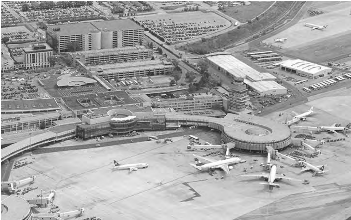
▲ 6.10 Vienna Airport: existing aerial photo – CAT station below landside terminal (Courtesy of Vienna International Airport).
