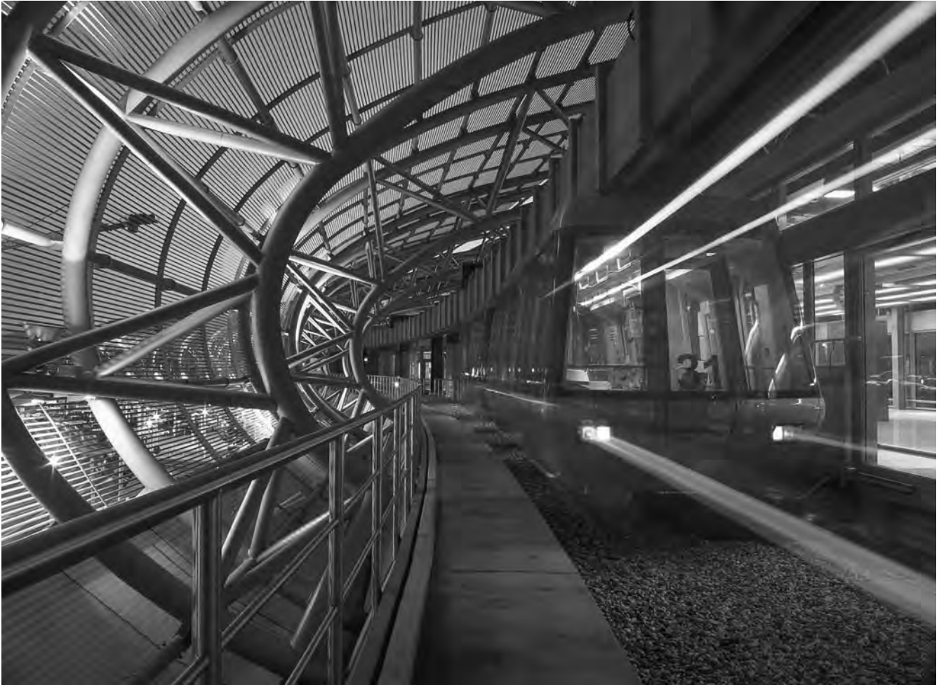
▲ 6.119 Photo of Skytrain 'inside' terminal (Courtesy of Düsseldorf International).
