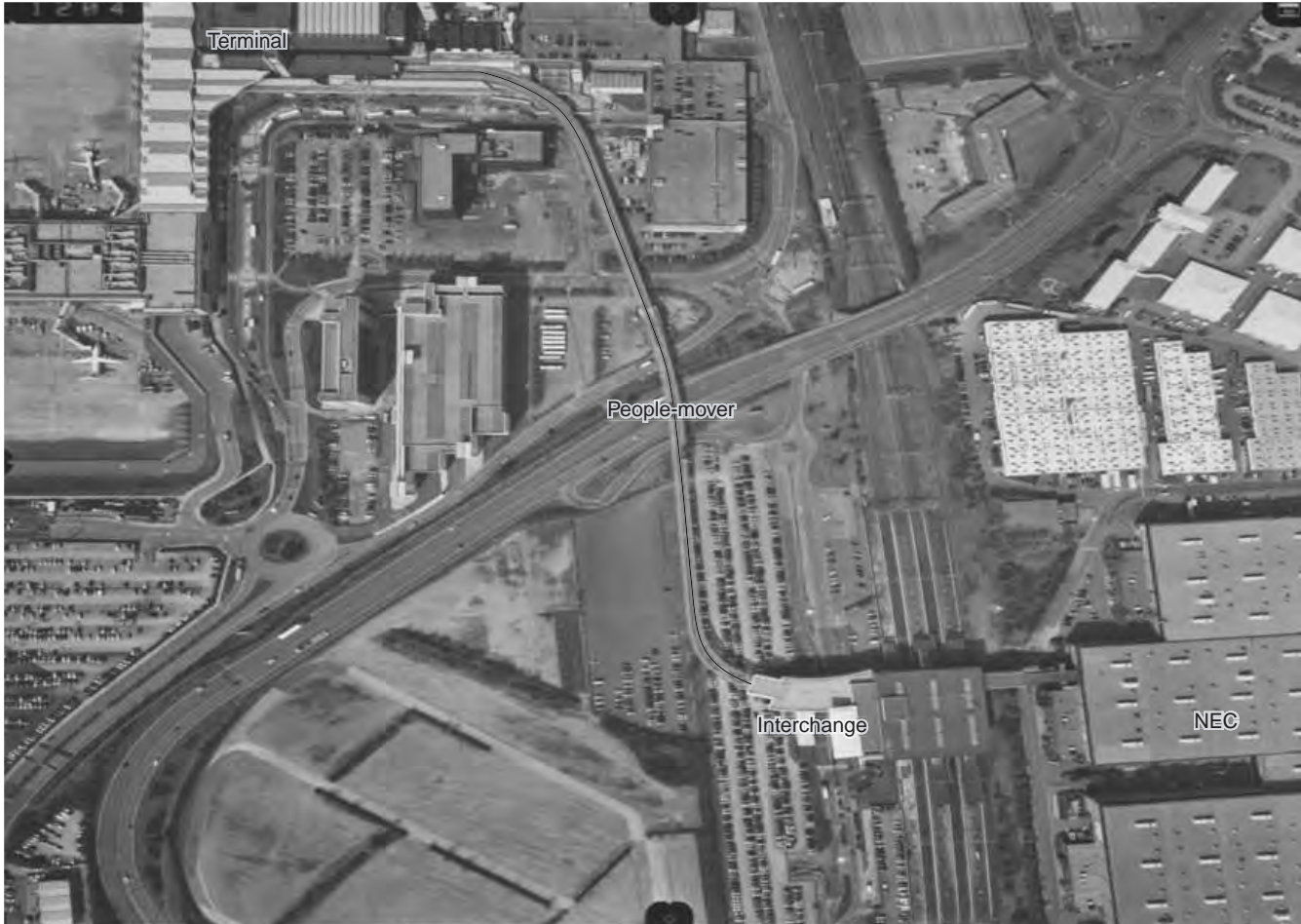
▲ 6.66 Birmingham International Airport: aerial photo, showing airport and NEC (Courtesy of Birmingham International Airport Ltd).
