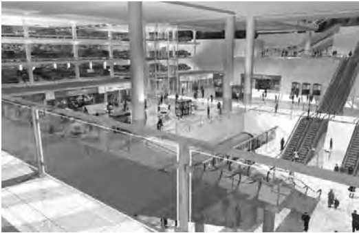
▲ 4.1 The rail parkway: circulation area and LRT platforms (Figures 4.1–4.6 courtesy of Halliburton KBR/YRM Architects Designers Planners).
