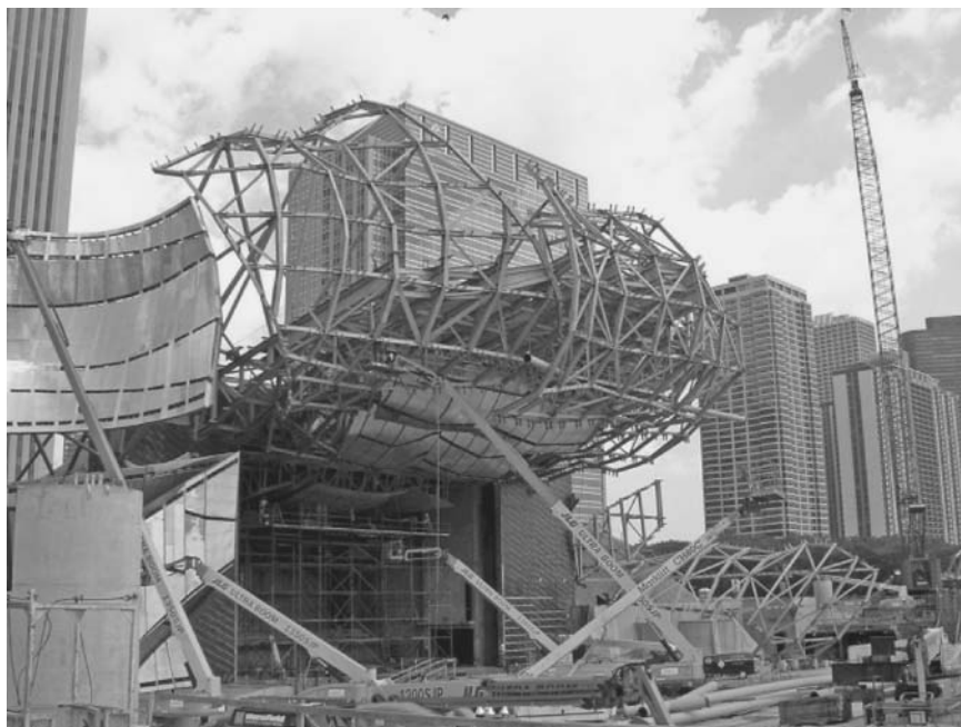
Figure 7.38 Using 3D coordinate system to locate steel—Millennium Park, Chicago, Illinois.
