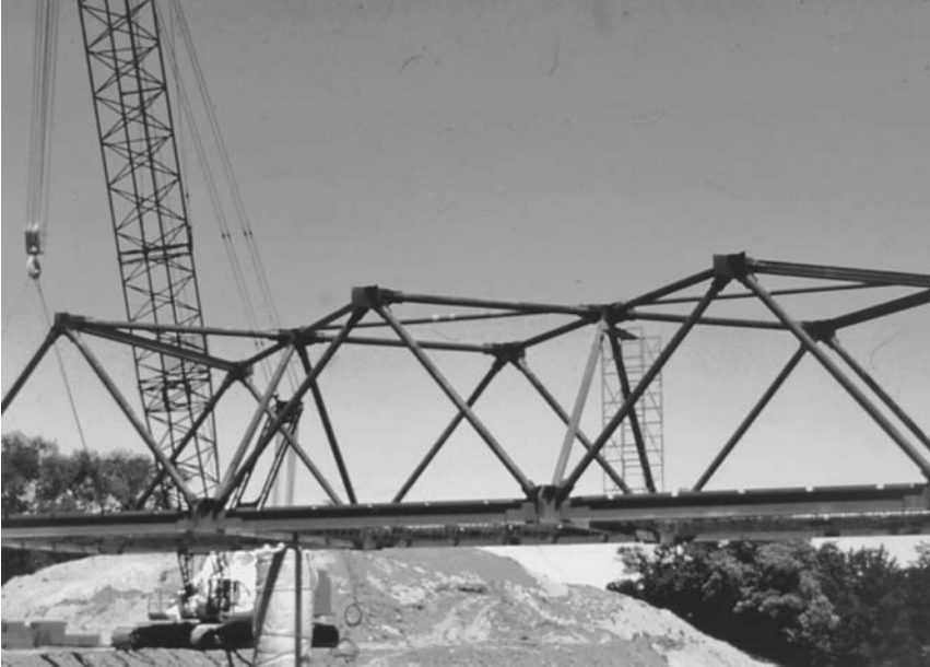
Figure 7.7 Space-frame module 42 by 126 ft being lifted into place—Carver-Hawkeye Arena.
