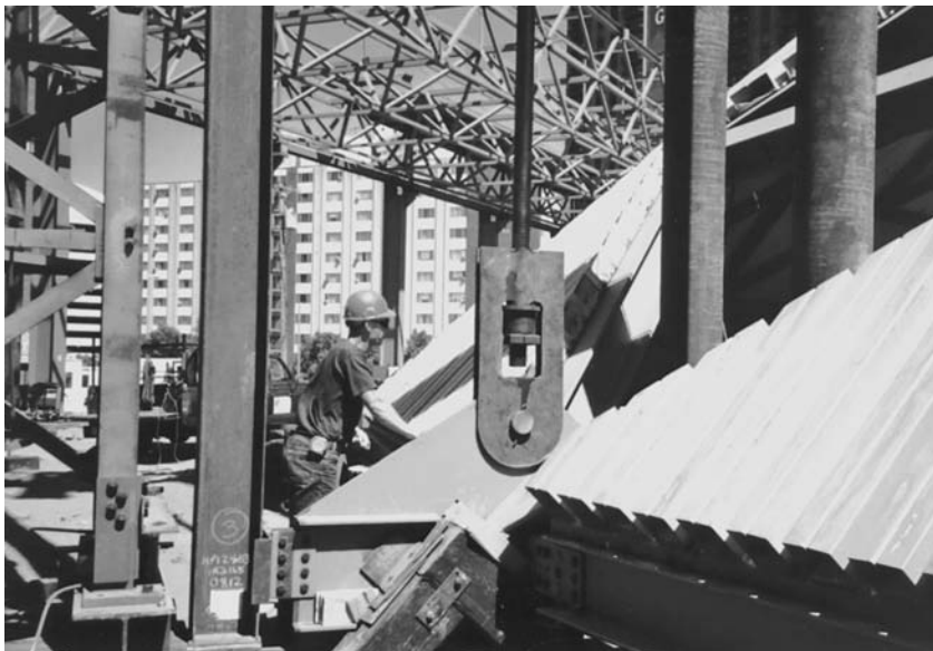
Figure 7.27 Jacking rods in position for lifting dome—Minneapolis Convention Center.
