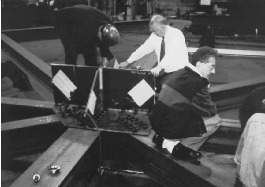
Figure 7.4 Trial joint assembly to establish bolt tensioning and inspection procedures—NWA Hangar, S. E. McClier and Computerized Structural Design.
