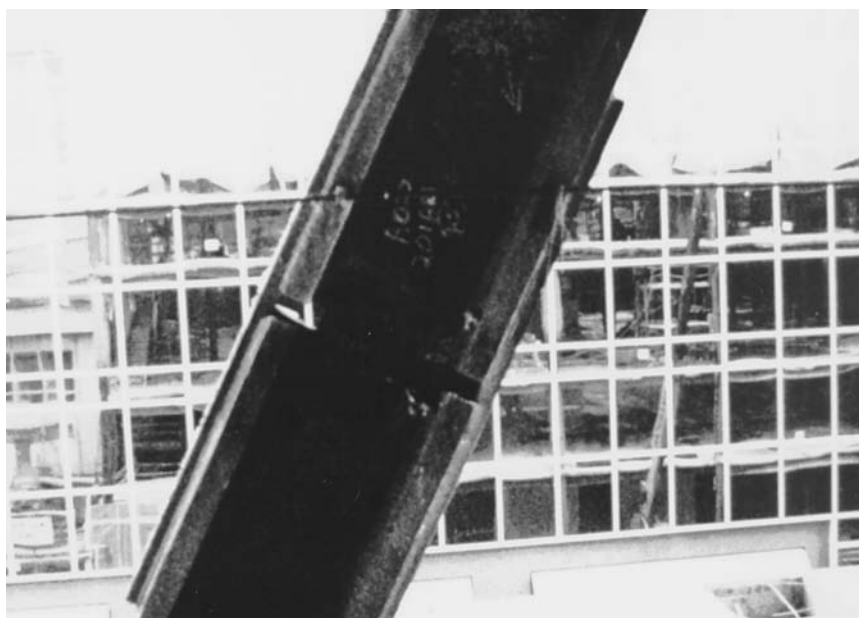
Figure 7.17 Adjustable midheight splice of bracing diagonal—Plaza Seven.
