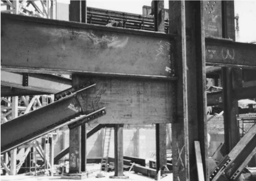
Figure 7.1 Large gusset plate due to concentric work point for brace.
