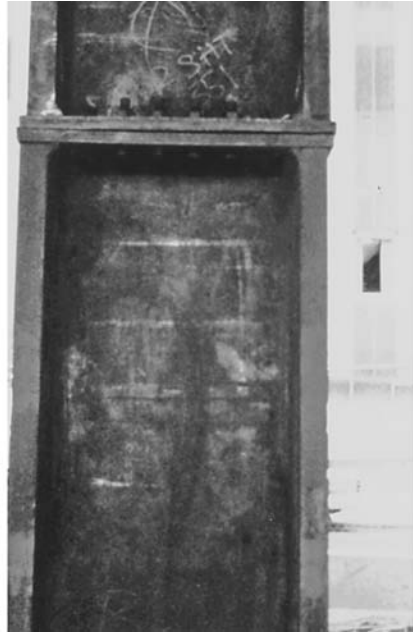
Figure 7.15 Splice of vierendeel verticals showing alignment—Norwest Financial Center.
