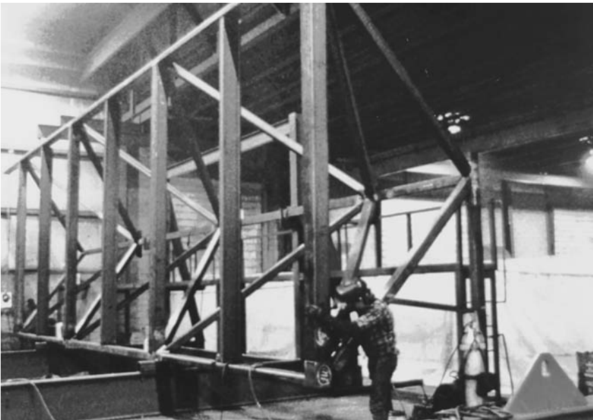
Figure 7.8 Space-frame module 15 by 60 ft rotated for shop welding—Minneapolis Convention Center, S. E. Skilling, Ward, Magnusson and Barkshire.
