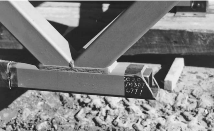
Figure 7.23 Space-frame bottom-chord splice connection—Minneapolis Convention Center.
