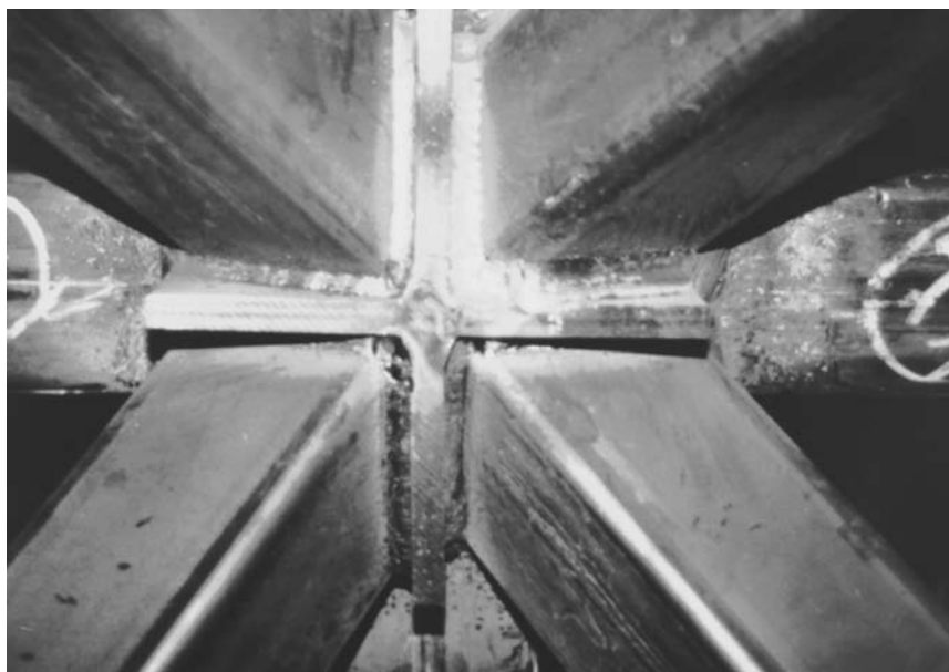
Figure 7.22 Space-frame bottom-chord showing weld—Minneapolis Convention Center.
