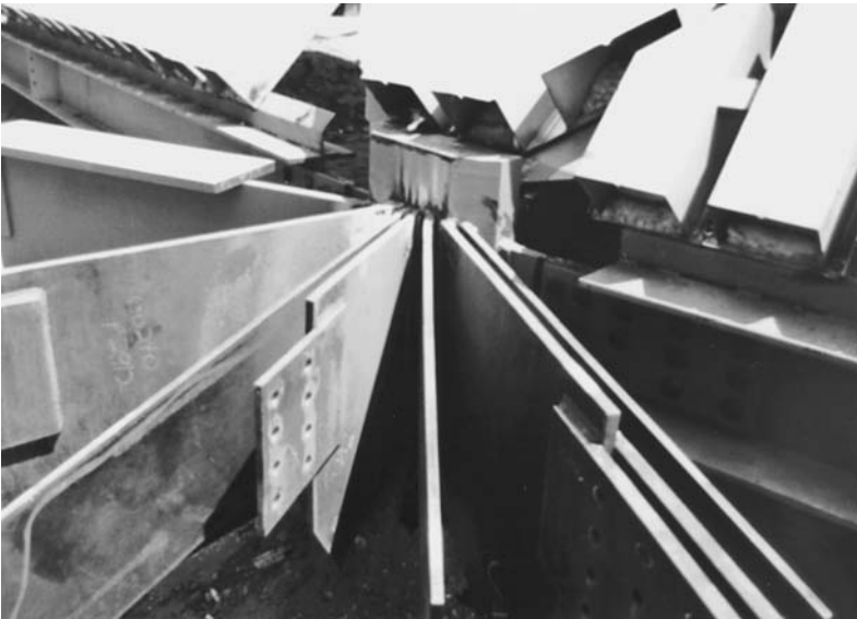
Figure 7.24 Gusset-plate connections for pipe struts to dome—Minneapolis Convention Center.
