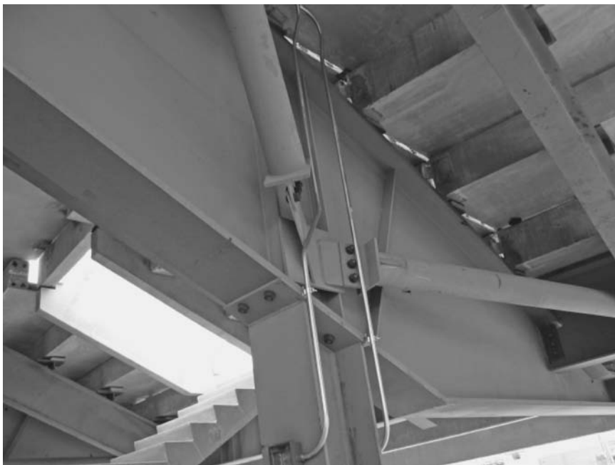
Figure 7.31 Steel raker with precast seating erected—University of Minnesota, TCF Stadium.
