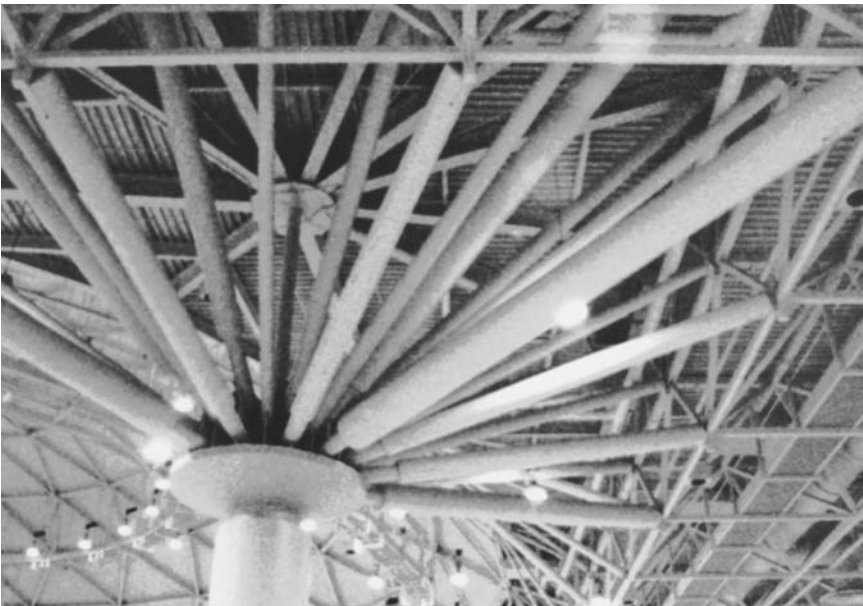
Figure 7.19 Dome and space-frame column and pipe supports—Minneapolis Convention Center.
