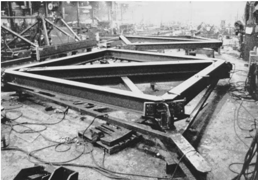
Figure 7.25 Lamella dome module in fabrication—Minneapolis Convention Center.
