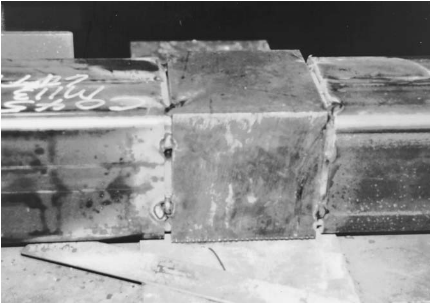
Figure 7.9 Solid 6-in 2 reinforcement for HSS joint—Minneapolis Convention Center.
