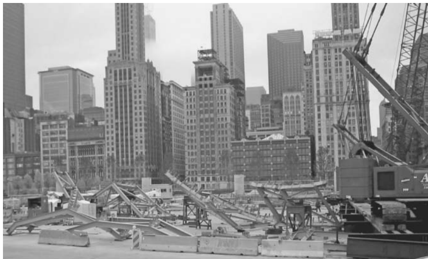
Figure 7.37 Subassembly shoring—Millennium Park, Chicago, Illinois.
