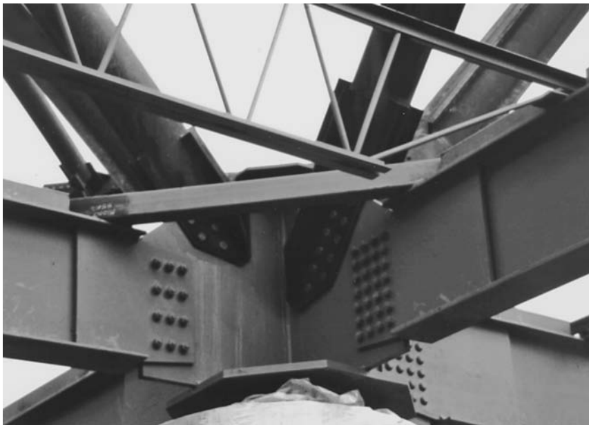
Figure 7.10 Bottom chord connection for space truss—Carver-Hawkeye Arena.
