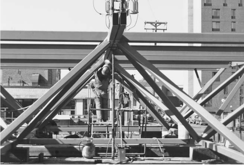
Figure 7.20 Top-chord field splice of delta space frame—Minneapolis Convention Center.
