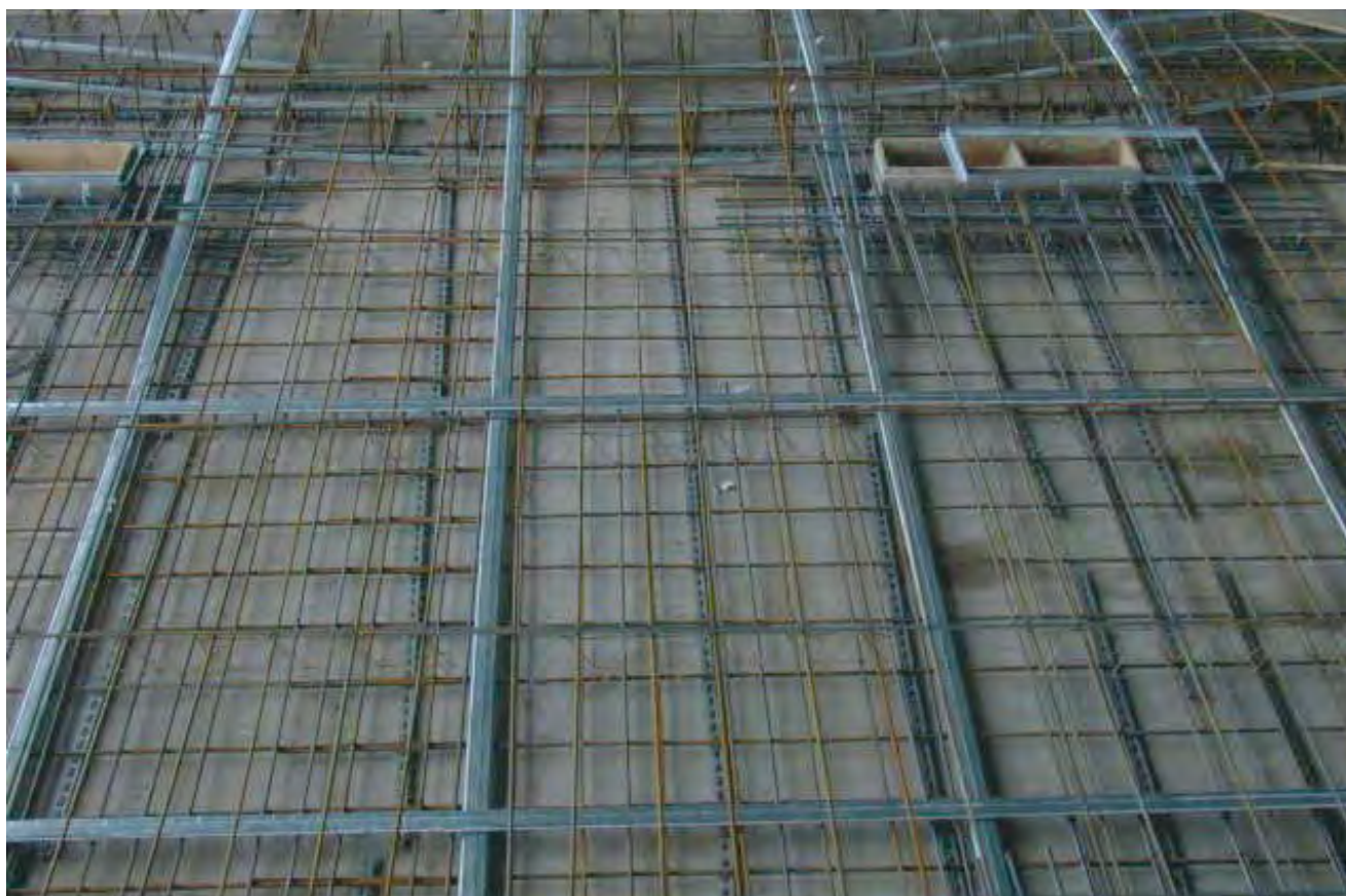
Figure 7.33 Slab and beam tendons in post tensioned slab (courtesy of Sir Robert McAlpine Ltd)
