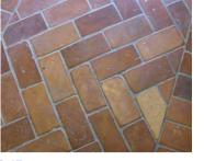
Old bricks can be cut into tiles with thickness approx. 1,6 cm and used as flooring. Source: Stavne gård.
