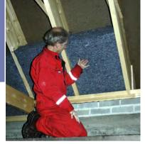
Insulation matting of recycled textiles. Source: Rolf Jacobsen/Ultimat. on recycled textiles are now becoming quite common (Figure 14.27). Discarded textiles are collected, and synthetic textiles are removed so that the final product contains over 95% wool and cotton. It is shredded and then heated to 120 °C while fibres of polyester (10–15% by weight) are melted in as a binder. Ammonium phosphate fire retardant may be added.
