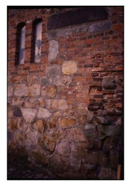
13.16 Wall with a mixture of recycled bricks and stones.
