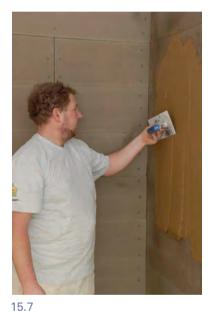
These are made of pure, clay rich earth reinforced with natural fibres such as wood shavings or shredded straw. They may be supplied with tongue and groove joints. As panels they are produced in dimensions up to 120 cm and are from 25 to 50 mm thick. Blocks are typically 10 cm thick and strong enough to use for internal partition walls.
