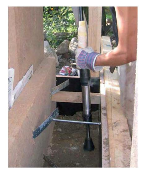
Ramming earth with pneumatic equipment. Source: Claytec.
