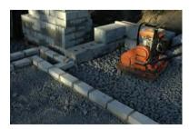
Expanded granules of recycled glass used as thermal insulation and capillary breaking layer in foundation. Gaia Tjøme, 2005.
