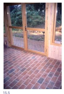
Floor covering of brick in sand, which are easy to remove and re-use.
