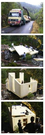
(A), (B), (C), (D). 4 phases in the erection of a kindergarten in massive wood elements. Rauli, Flekkefjord (Norway). Gaia Lista, 2005.
