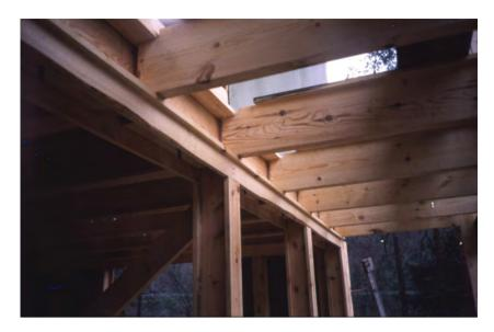
A structure designed for re-use. The structure is produced of prefabricated and standardized monomaterial components in wood and concrete, which can easily be dismantled and re-used. Gaia Lista, 1995.
