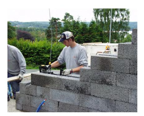
**13.5** *Mortar free construction with concrete lightweight blocks.* Source: Maxit.
