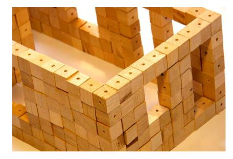
The 'climate cube' building system consists of massive wooden blocks, see Figure 13.44, piled up to complete walls. The cubes are connected to each other with wooden plugs. No glues are used and the blocks can be easily disassembled for re-use. Gaia Lista, 2005.
