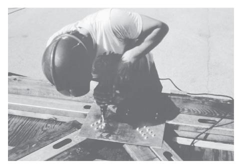
A worker tightens the last screws to complete a connection in a light gauge steel roof truss. The truss members are held in alignment during assembly by a simple jig made of plywood and blocks of framing lumber. (Courtesy of Unimast Incorporated—www.unimast.com)
