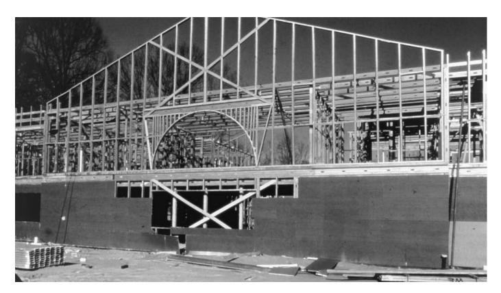
FIGURE 12.17 Gypsum sheathing panels have been screwed onto most of the ground-floor walls of this large commercial building. (Courtesy of Unimast Incorporated—www.unimast.com)
