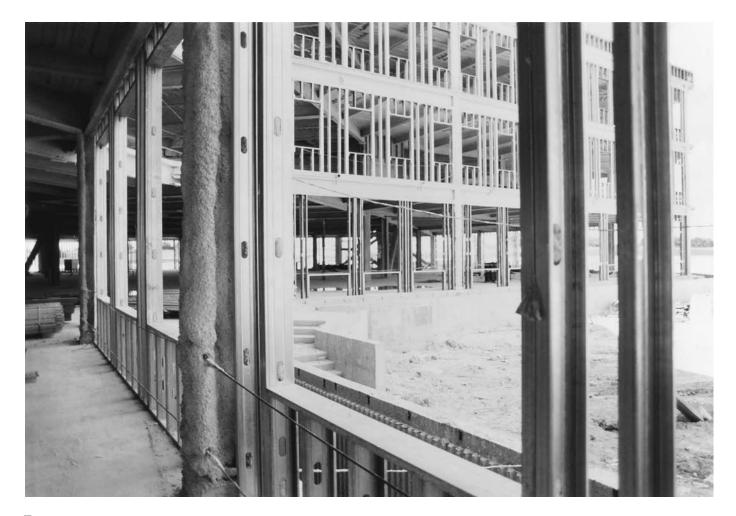
FIGURE 12.13 Light gauge steel stud walls frame the exterior walls of a building whose floors and roof are framed with structural steel. (Courtesy of Unimast Incorporated—www.unimast. com)
