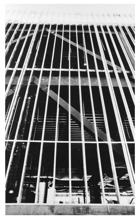
FIGURE 12.14 The straightness of steel studs is apparent in these tall walls that enclose a building framed with structural steel. (Courtesy of Unimast Incorporated www.unimast.com)
