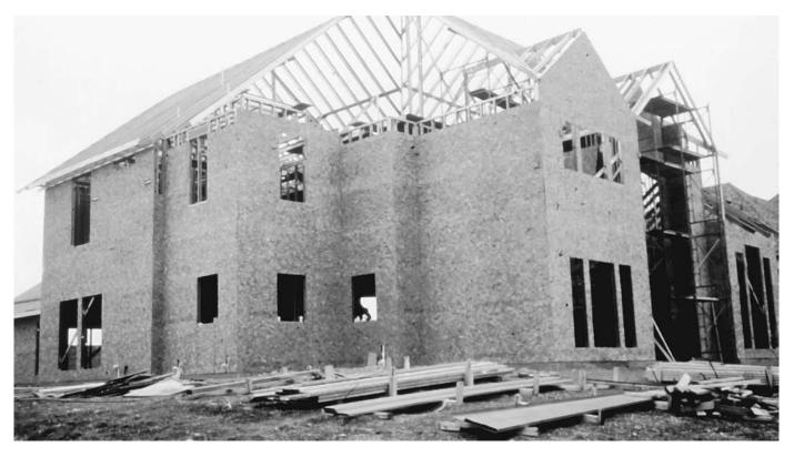
FIGURE 12.18 Waferboard (a wood panel product similar to OSB) sheaths the walls of a house framed with light gauge steel studs, joists, and rafters. (Courtesy of Unimast Incorporated—www.unimast.com)
