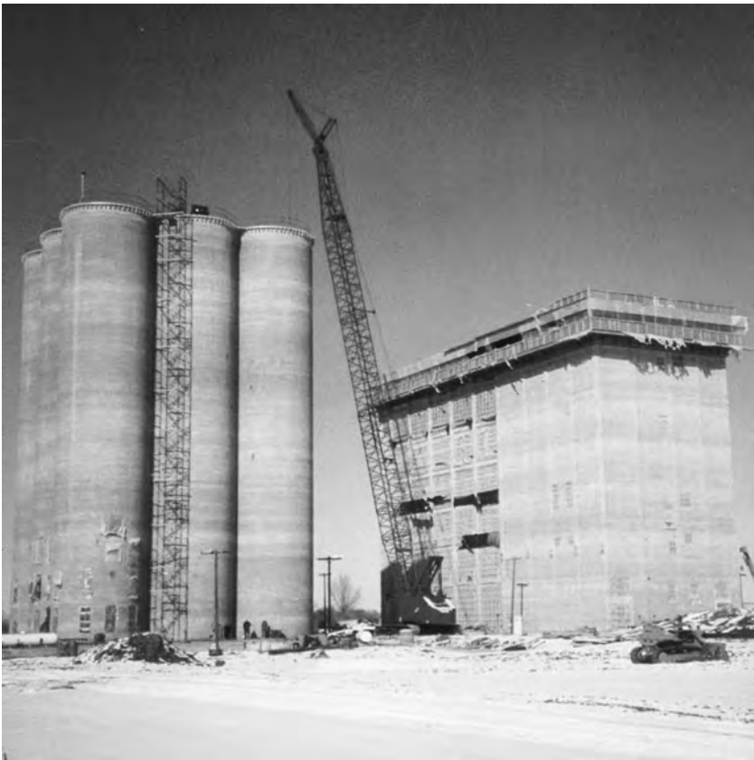
FIGURE 15-7 Grain storage and mill building slipformed in South Sioux City, Nebraska. (Source: Younglove Construction Company)
