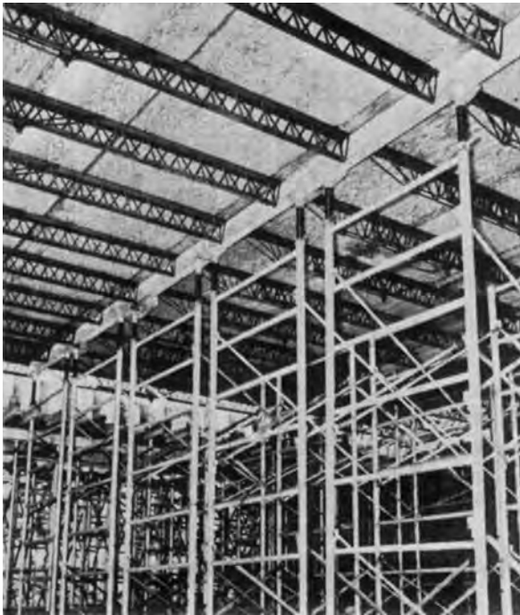
FIGURE 12-15 Plywood decking installed directly over horizontal shoring. (Source: Patent Construction Systems)
