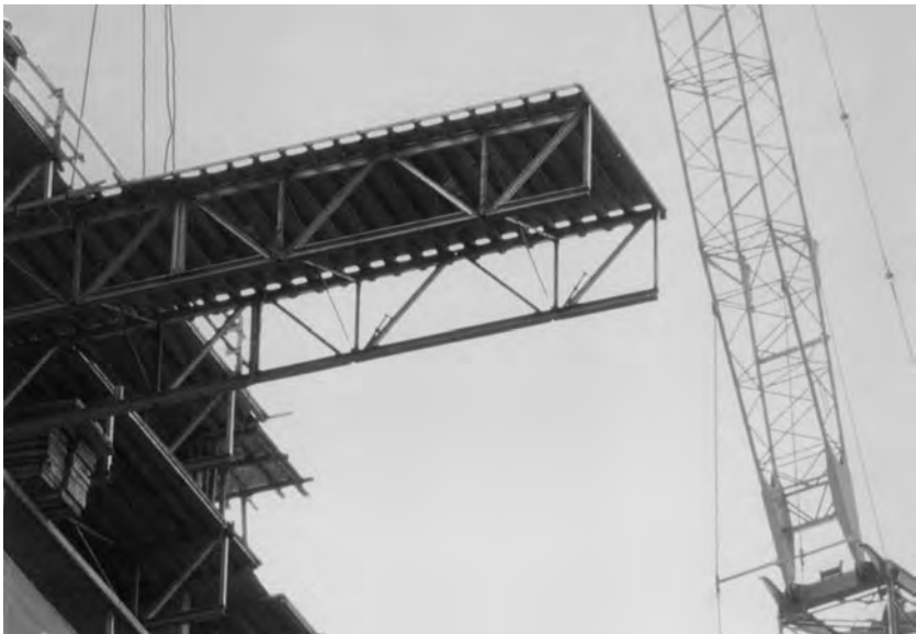
FIGURE 17-14 Landing a flying form table at a new location. (Source: Patent Construction Systems)
