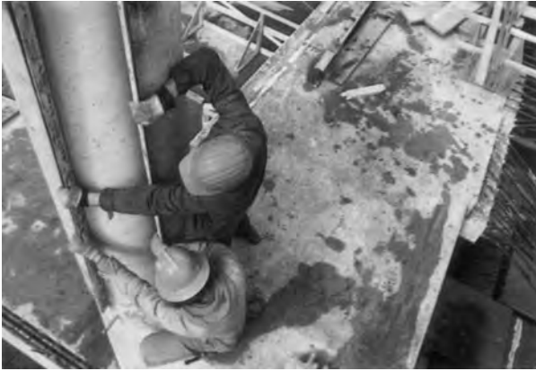
FIGURE 10-22 Opening form after pour. (Source: Symons Corporation)
