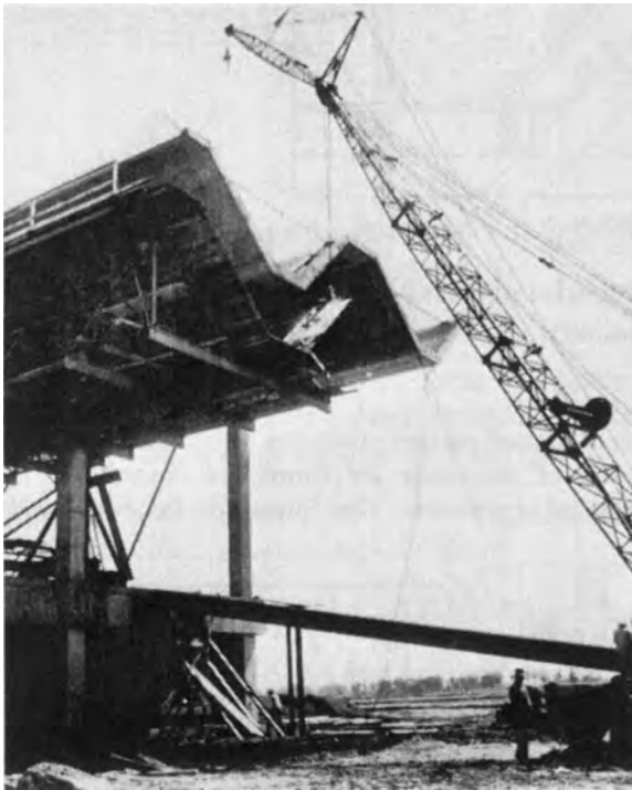
FIGURE 14-14 Plywood sheathing used to cast concrete roof member. (Source: APA—The Engineered Wood Association)
