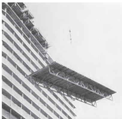
(a) Lifting a flying form table
