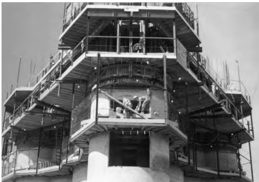
FIGURE 15-9 Slipform assembly for 568-ft tower. (Source: Sundt Corporation)
