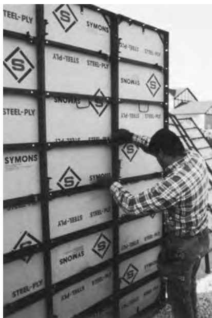
FIGURE 9-41 Hand setting modular panels. (Source: Symons Corporation)
