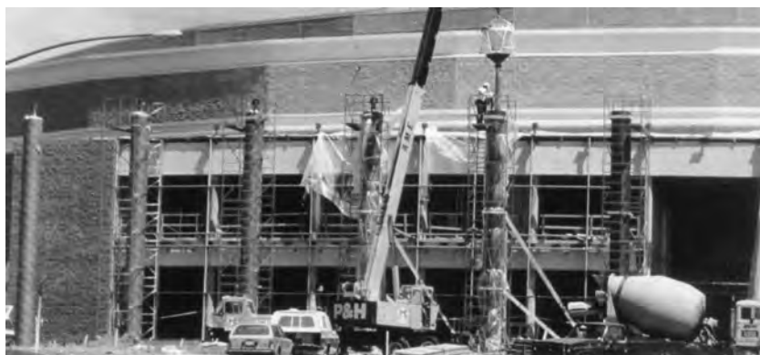
FIGURE 10-16 Placement of concrete in round fiber tube columns. (Source: Sonoco Products Company)
