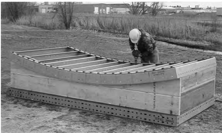
FIGURE 9-47 Tightening bolts on tension strap to obtain the desired radius for a curved wall. (Source: EFCO)
