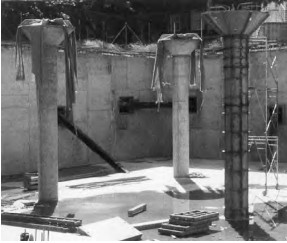
FIGURE 10-19 Steel column forms with capitals. (Source: EFCO)
