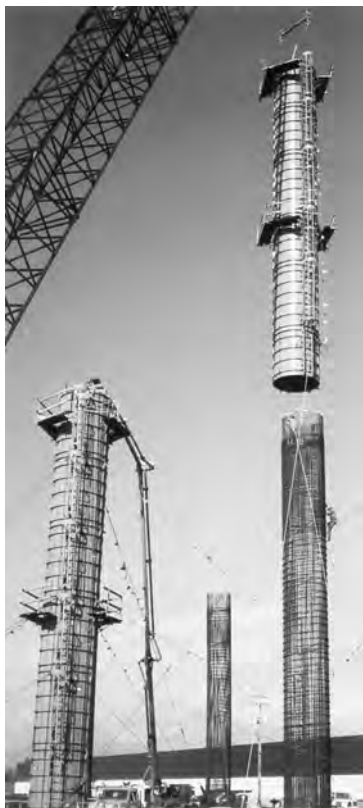
FIGURE 10-18 Slipping one-piece steel round column form over reinforcement. (Source: EFCO)
