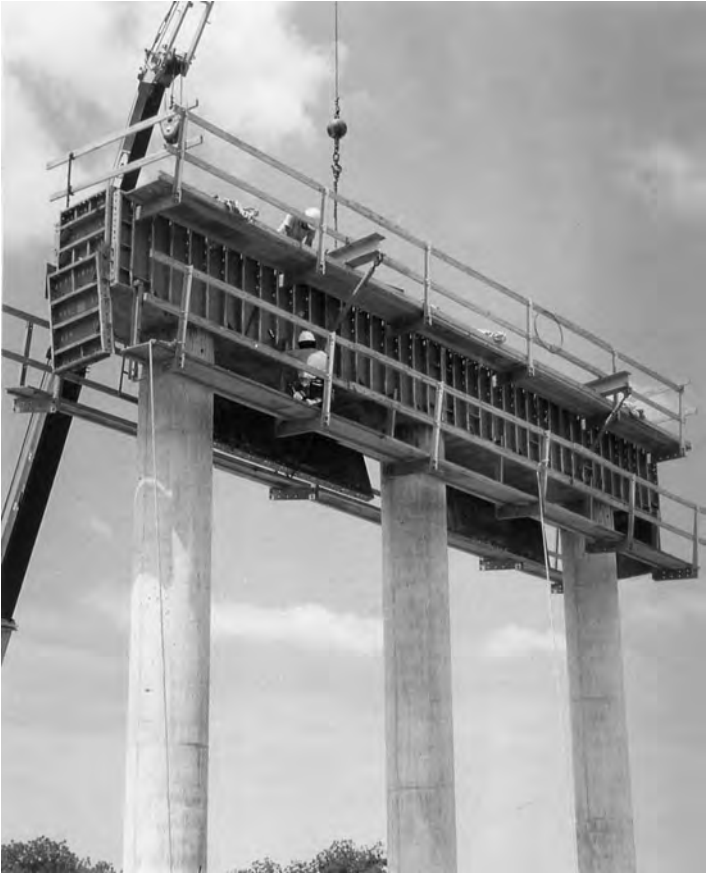
FIGURE 16-12 All-steel forming system for bridge structures. ( Source: EFCO )
