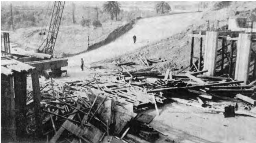
FIGURE 7-2 This falsework collapsed while being adjusted to grade.
