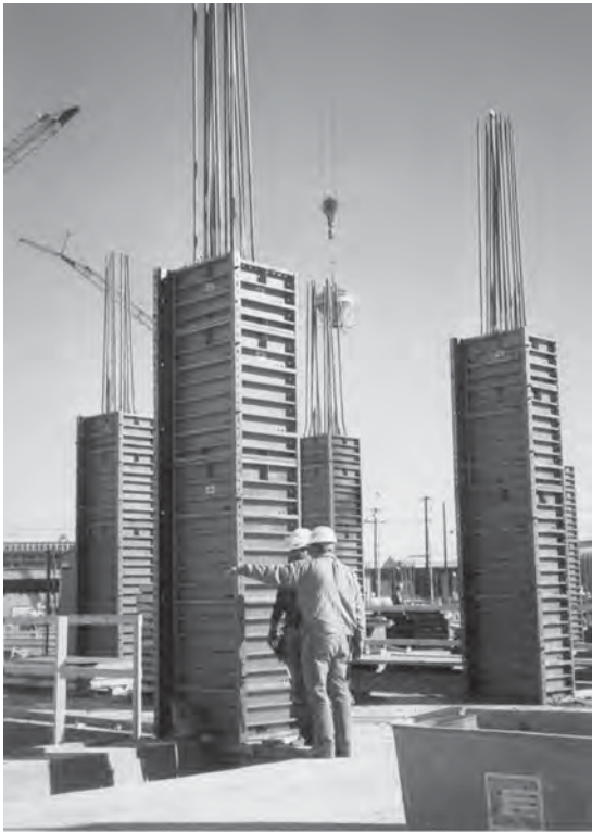
(a) Positioning all-metal column form
