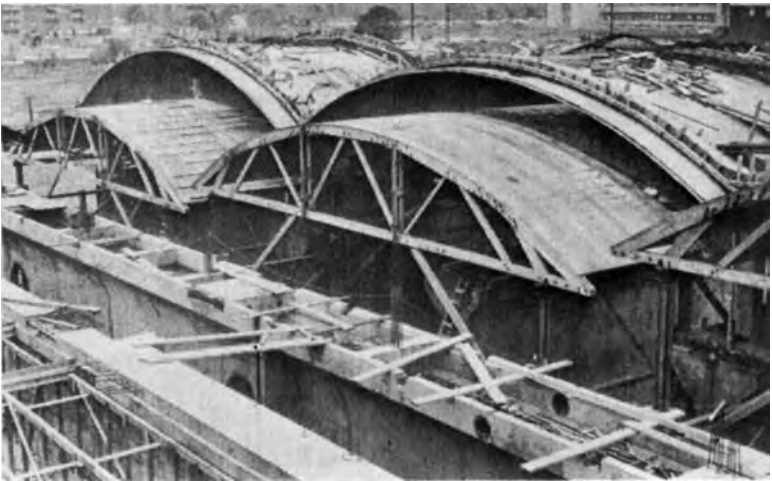
FIGURE 13-7 Formwork for a circular shell roof lowered for moving to new location. (Source: Construction Methods and Equipment )
