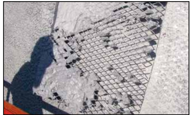
Figure 49: Exposed Zinc Mesh
