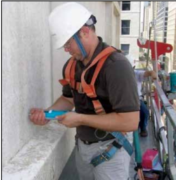
Figure 10: Rebound (Schmidt) Hammer Test
