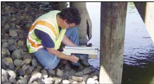
Figure 5: Resistance Drill for Detecting Decay in a Wooden Member (Reference 10)
