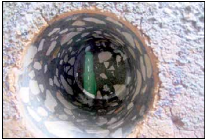
Figure 37: Epoxy Coated Reinforcement Bar with 5.5" Cover
