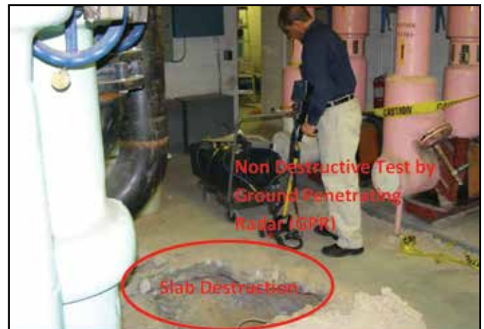
Figure 1: Non-Destructive Evaluation versus Destructive Evaluation for Void Detection
