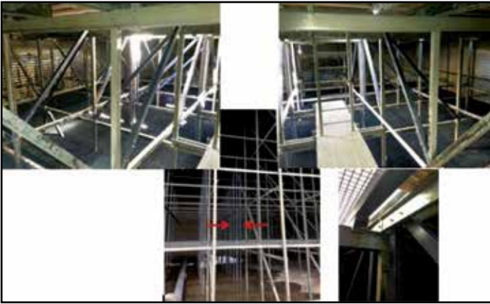
Top pictures show completed installation of supports Center: vertical supports (x6) Bottom right: connection of supports to motor mounting frame Overall mechanical install went very smoothly: 5 man crew, 5 days (day shift only) and crew had no prior experience with this.
