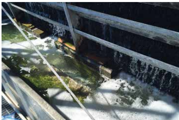
Figure 2: CMIT/MIT surfactant blend causes minimal foaming during field trial testing.
