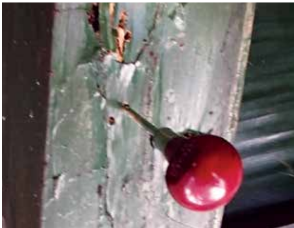
Figure 24: Wood pick probe used in evaluating depth of deterioration in wood
