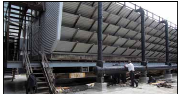
Figure 53: General View of Cooling Tower Supported on Steel Framing
