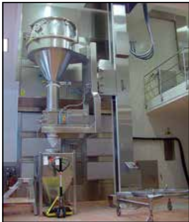
Müller lifting equipment in action
