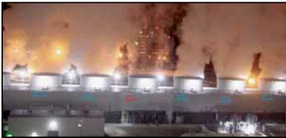
Figure 17: Heavy Plume Conditions during Night-time Operation in Winter
