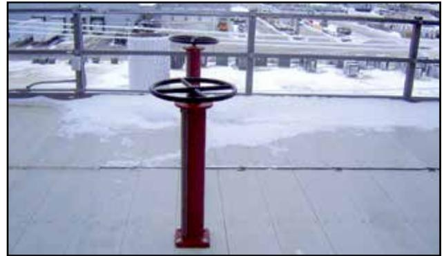
Figure 14: Valve Actuators on Fan Deck
